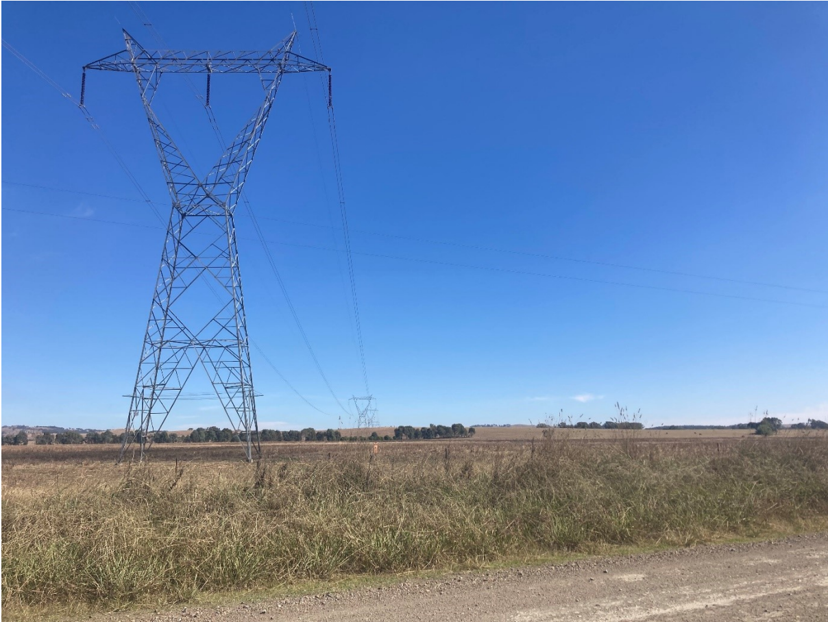
Figure 5-3 Area within the project footprint, near Big Springs (south-east of Gregadoo). View to the north-west showing cropping land and existing transmission Line 51
