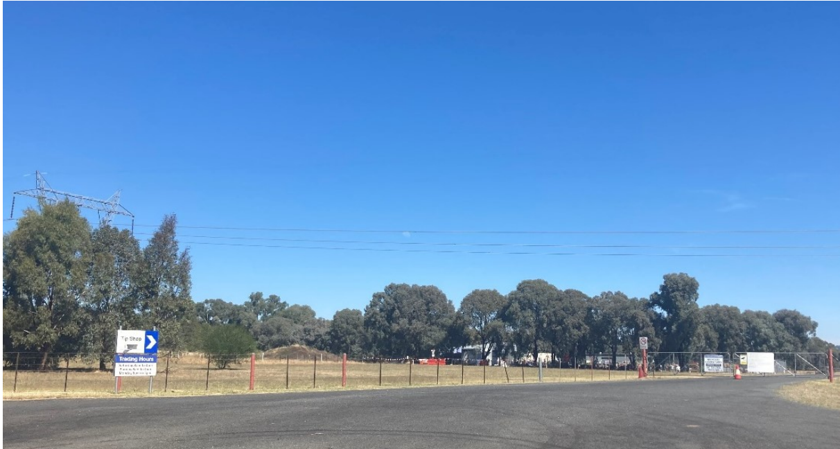
Figure 5-12 Area within the project footprint, alongside Ashfords Road, Gregadoo, approximately 350 metres south of the existing Wagga 330 kV substation, showing the Gregadoo Waste Management Centre Tip Shop and existing transmission lines.
