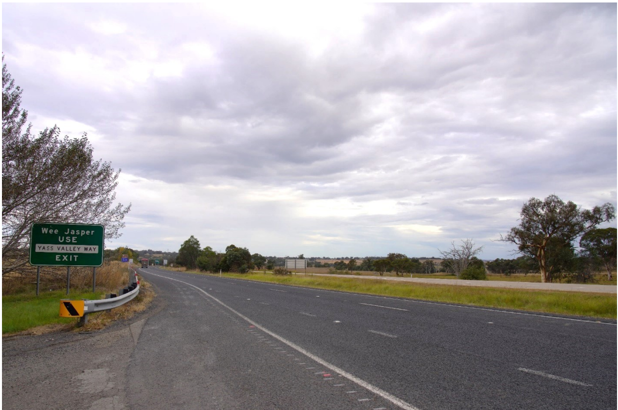
FIGURE 7-43 VIEW EAST FROM THE HUME HIGHWAY, YASS
