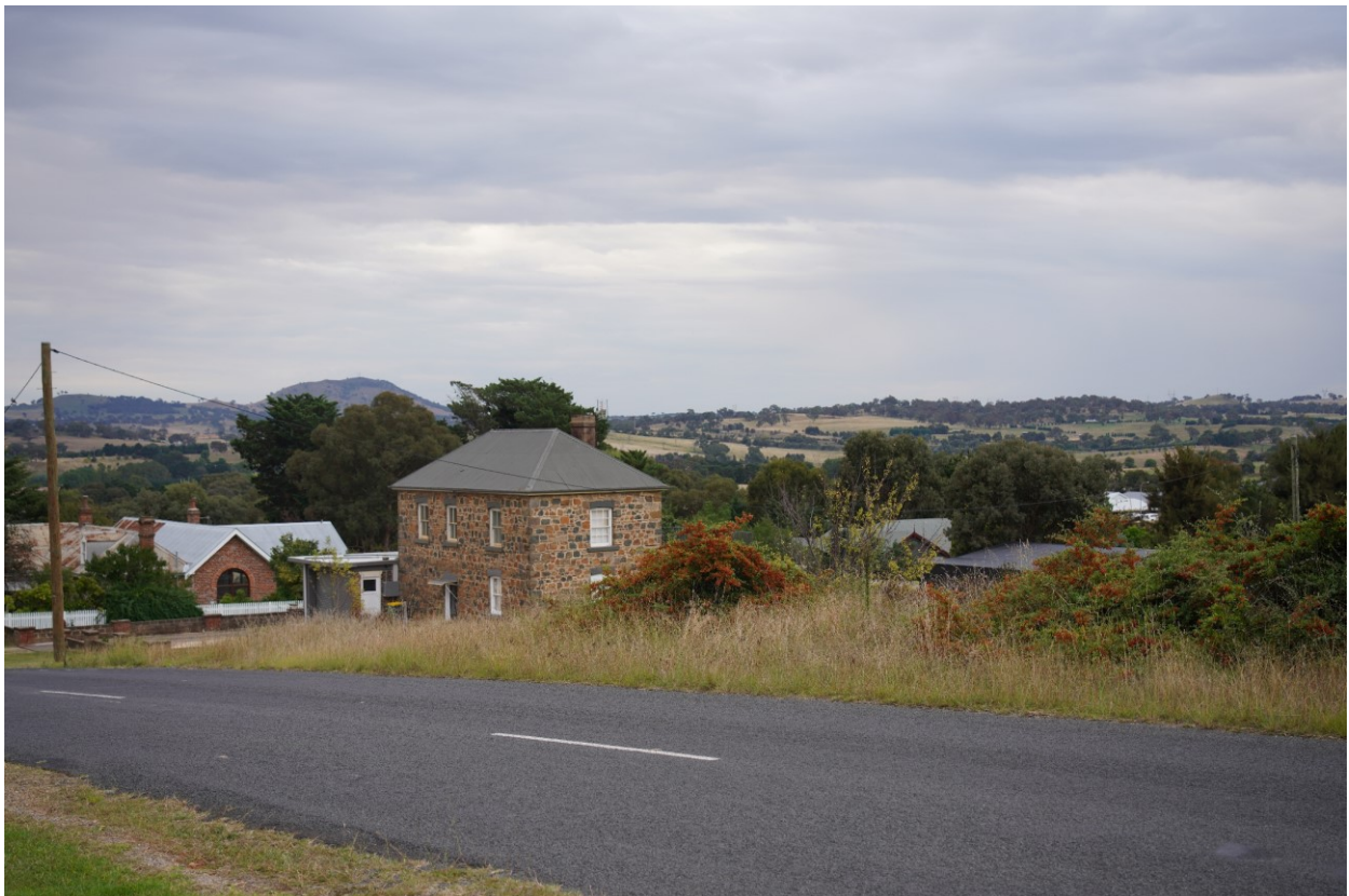
FIGURE 7-45 VIEW NORTH-WEST FROM ORION STREET, YASS
