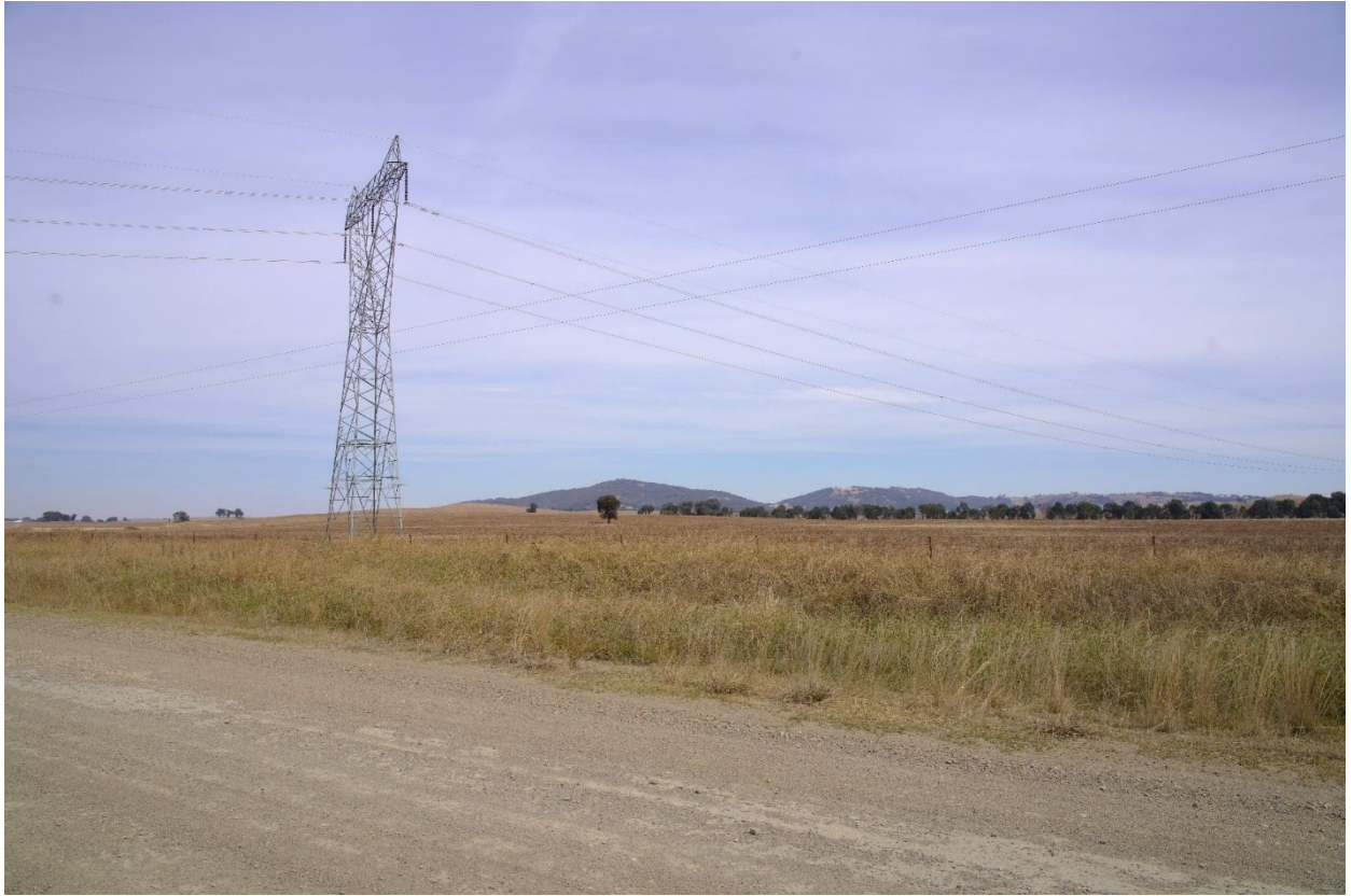
FIGURE 7-3 VIEW SOUTH FROM LIVINGSTONE GULLY ROAD
