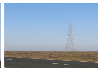
Cables extending across the view
