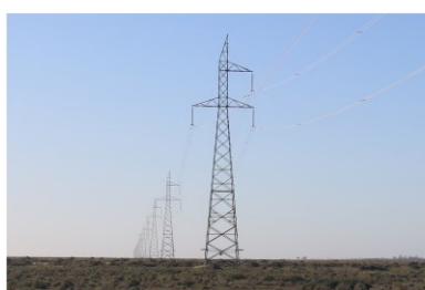
Transmission towers and overhead wires extending away from viewer
