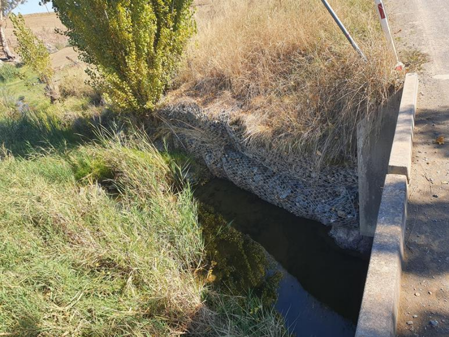
Gabion baskets on left bank of Killimicat Creek
