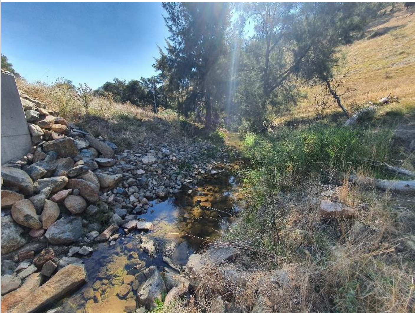
Rock wall protection of creek banks, facing downstream of Oak Creek
