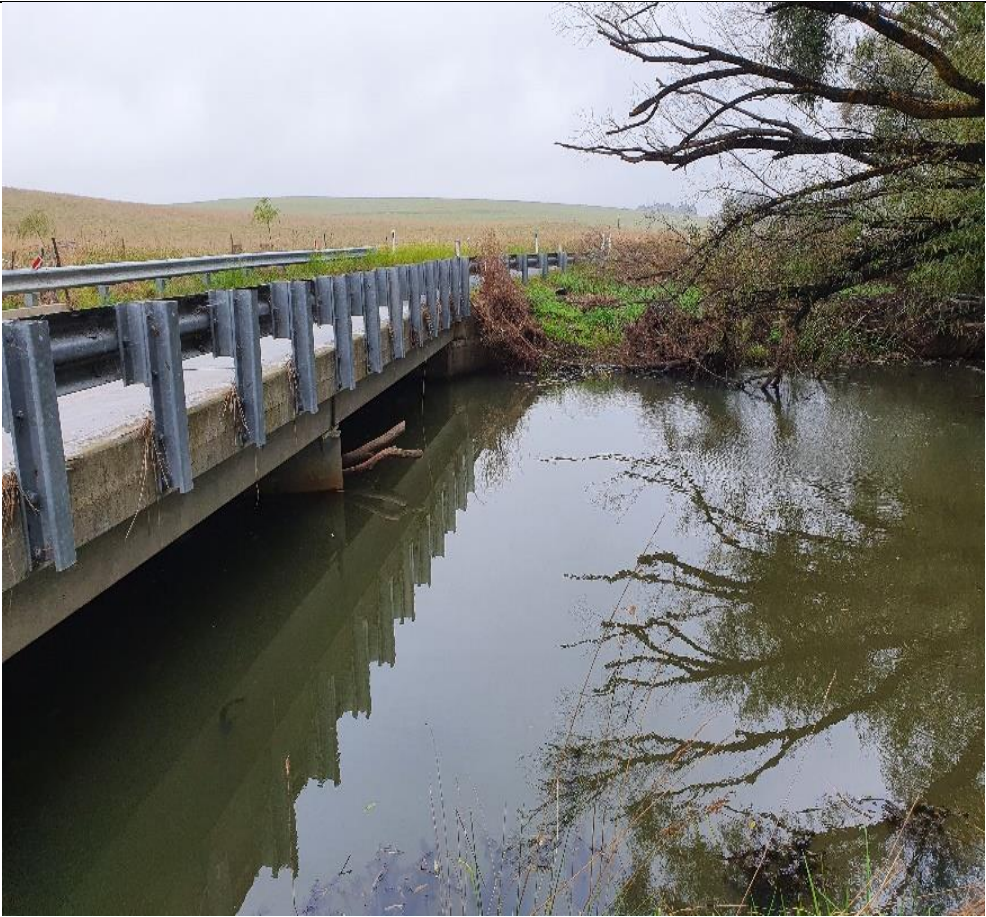
Road and bridge
