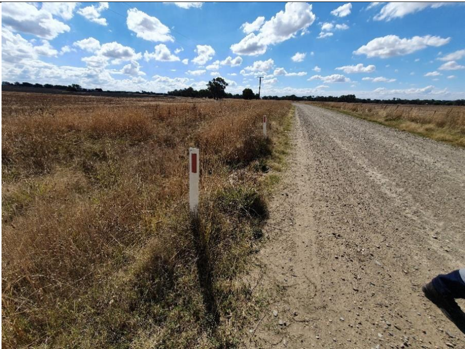
Channel running alongside road leading into culvert
