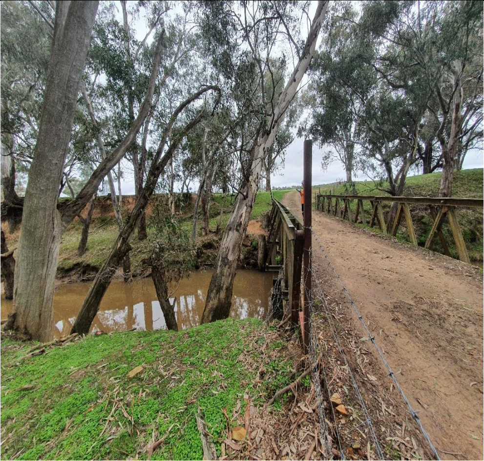
Bridge crossing O'Brien's Creek
