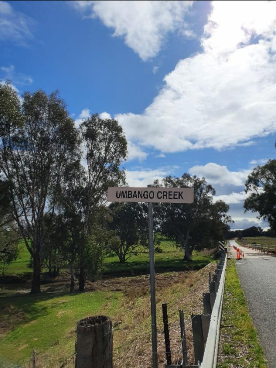
Road/bridge crossing Umbango Creek
