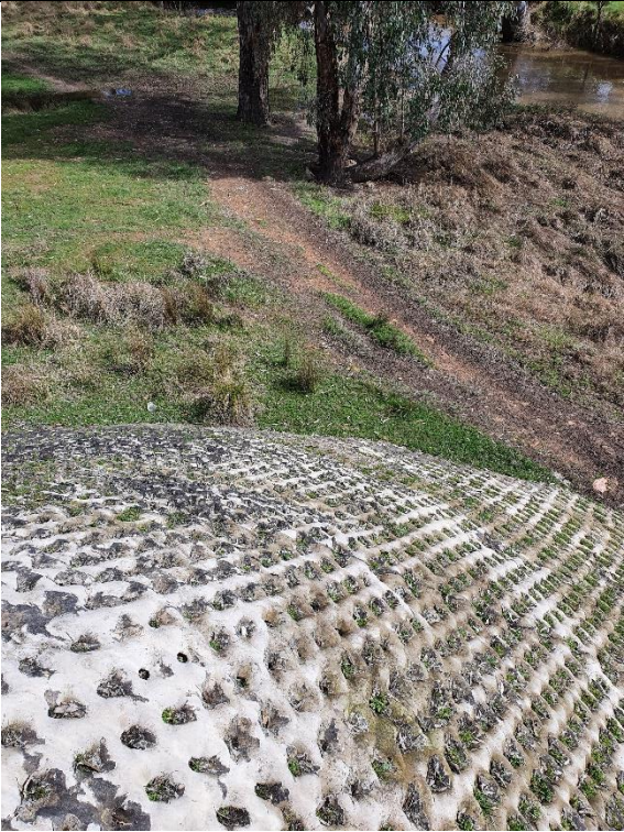
Bank protection structure underneath bridge/road
