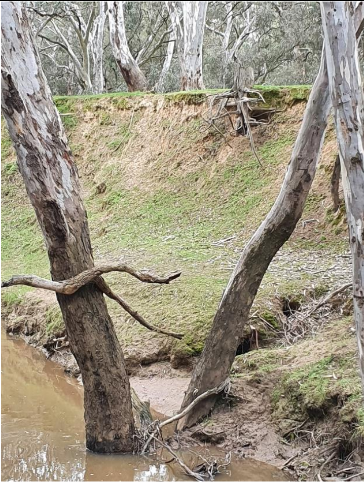
Eroded right bank
