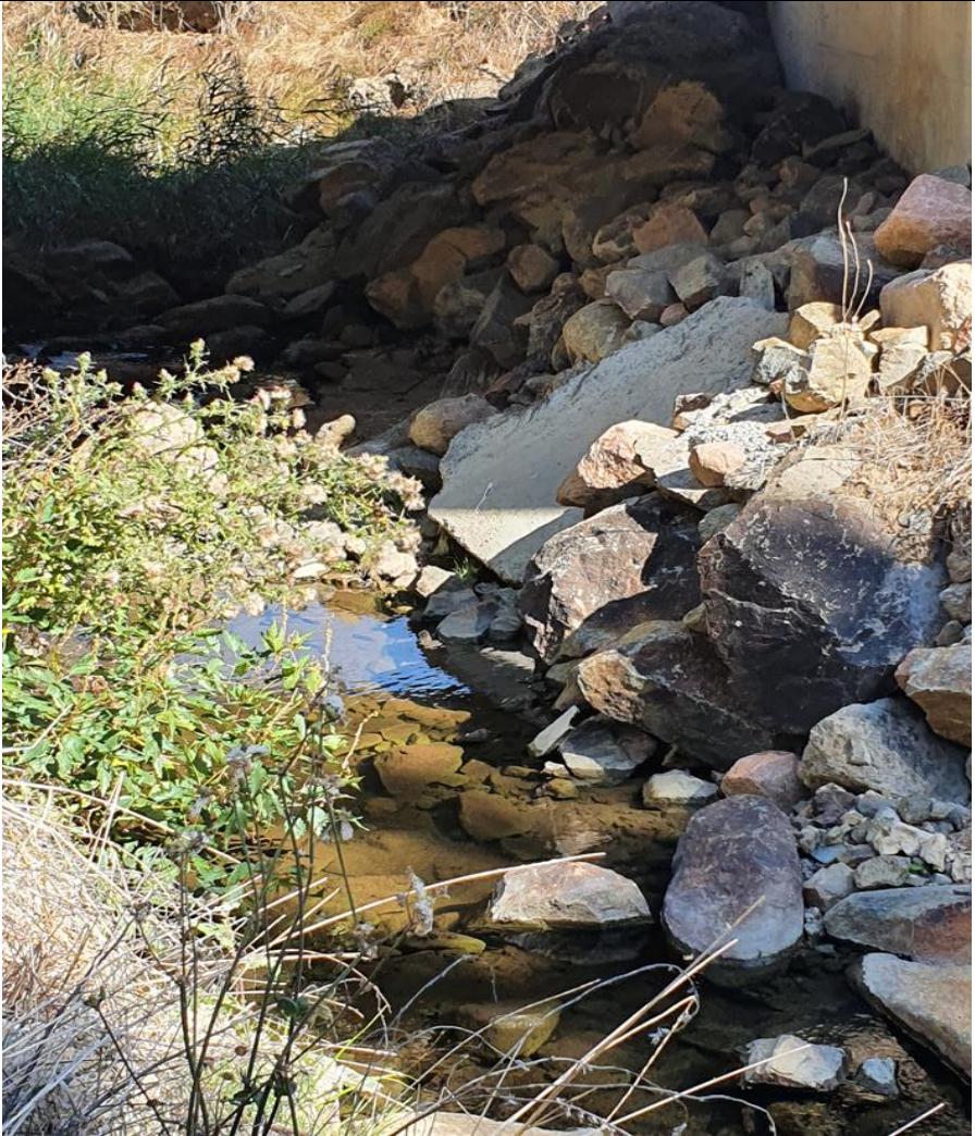
Rock wall underneath bridge crossing Oak Creek
