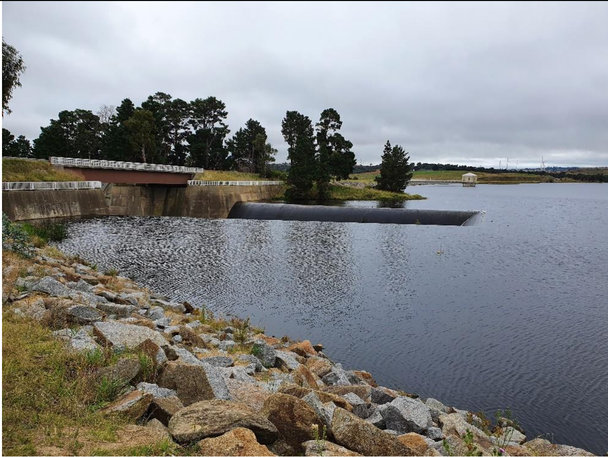
Pejar Dam spillway into Wollondilly River
