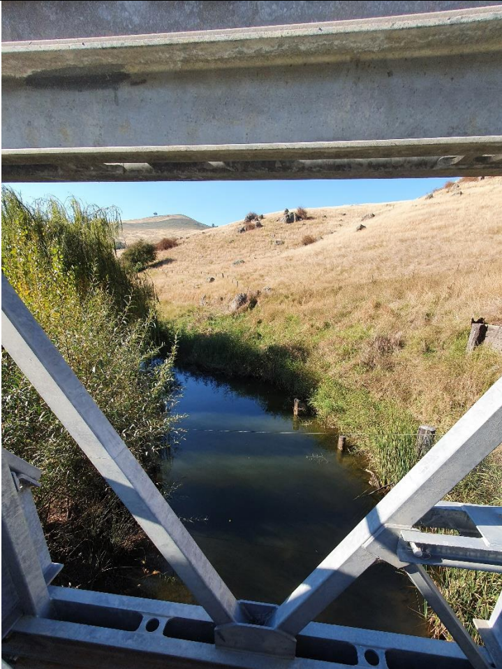
Downstream of Derringullen Creek
