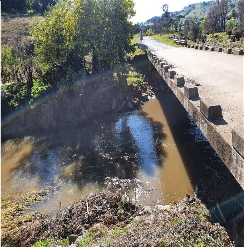
Bridge crossing Adjungbilly Creek and looking down stream
