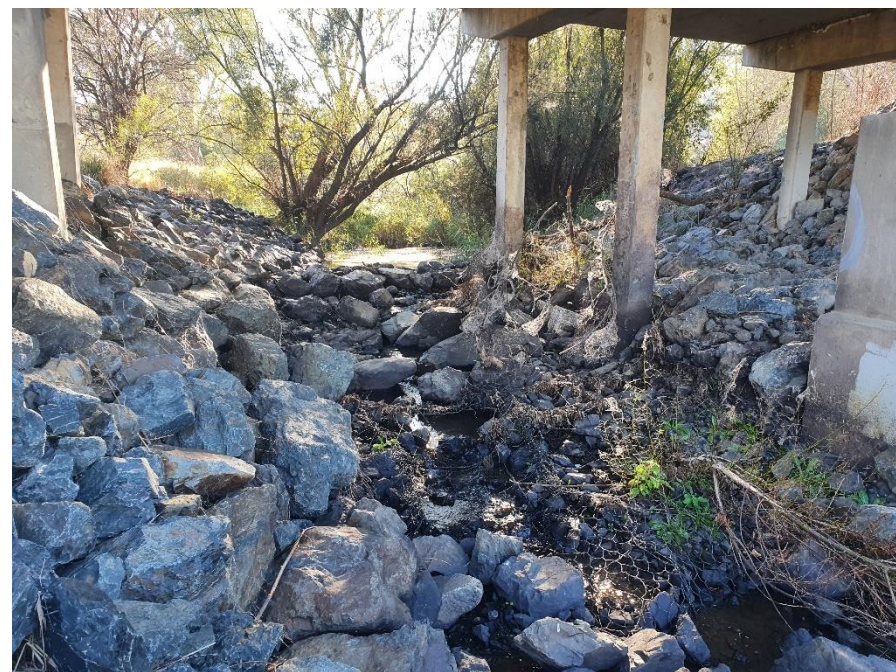
Under bridge, rock wall on both sides of creek
