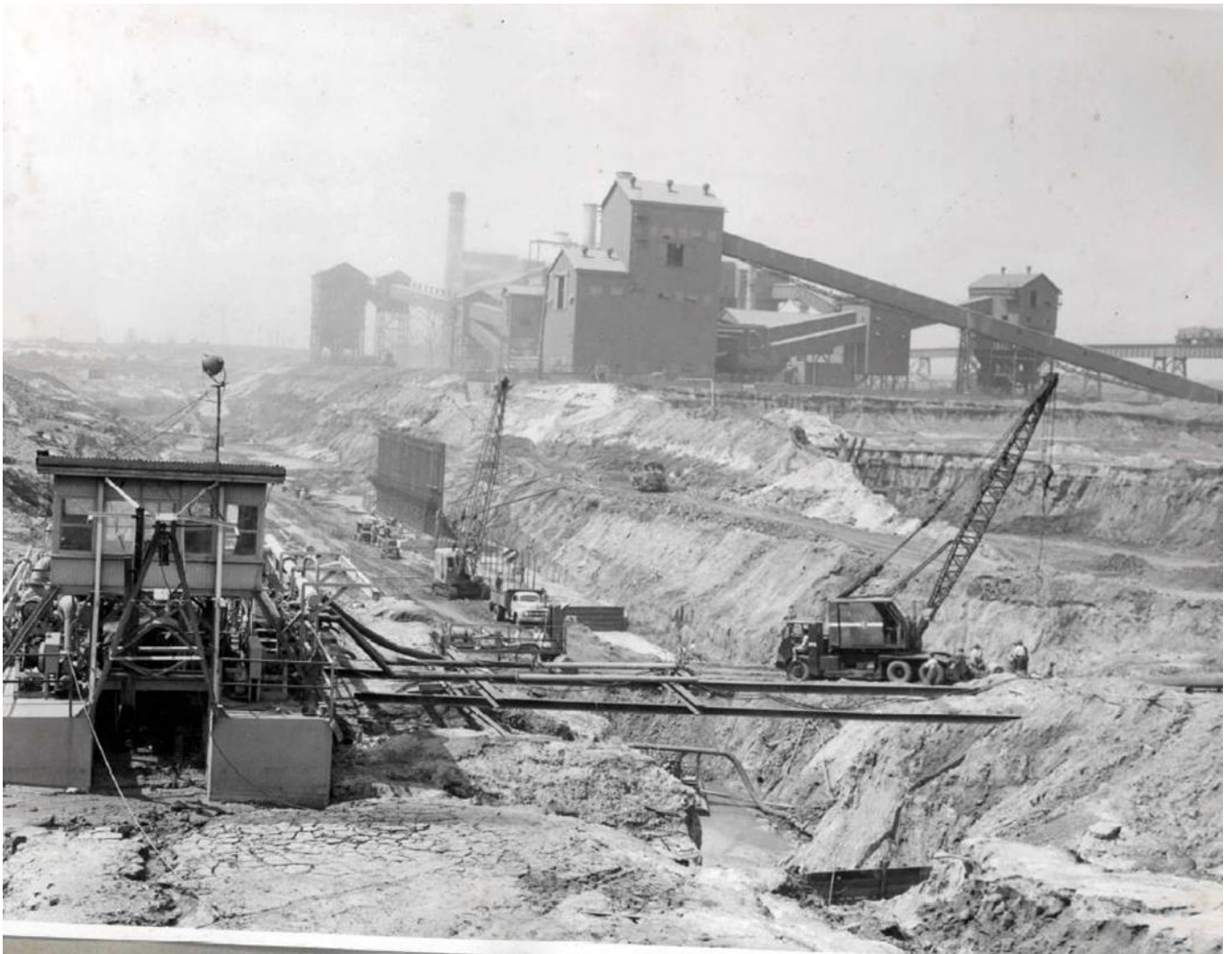
Figure 3.3 Construction of Berth 113 (source: BlueScope records)
