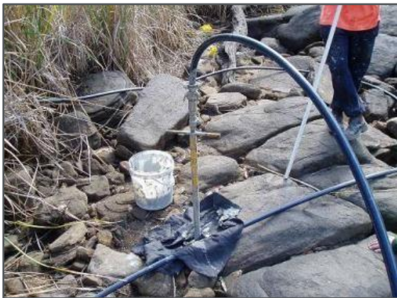
Plate A9-4 – Example of Rockbar Grouting Injection Undertaken in the Georges River
