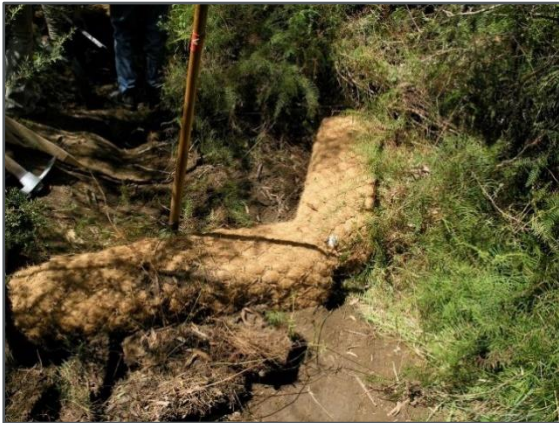
Plate A9-5 – Square Coir Logs for Knickpoint Control Source: Good et al. (2010).
