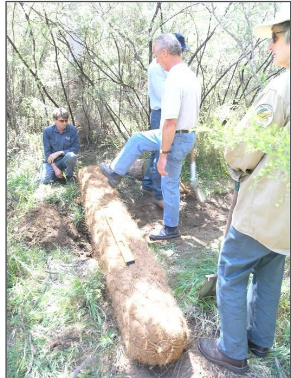
Plate A9-7 – Round Coir Logs Installed to Spread Water Source: Good et al. (2010).
