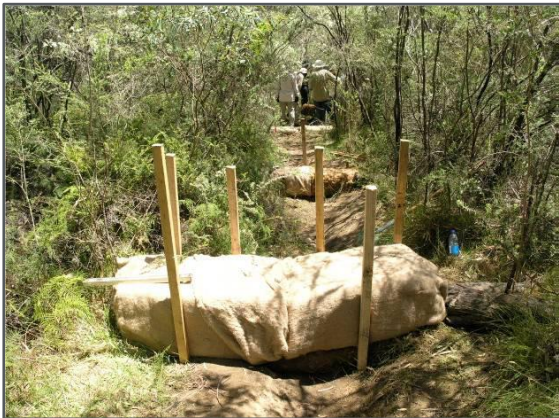
Plate A9-6 – Coir Log Dams Constructed at Intervals with Wrapping of Fibre Matting Source: Good et al. (2010).
