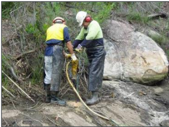
Plate A9-3 – Drilling into Bedrock to Form Grouting Holes
