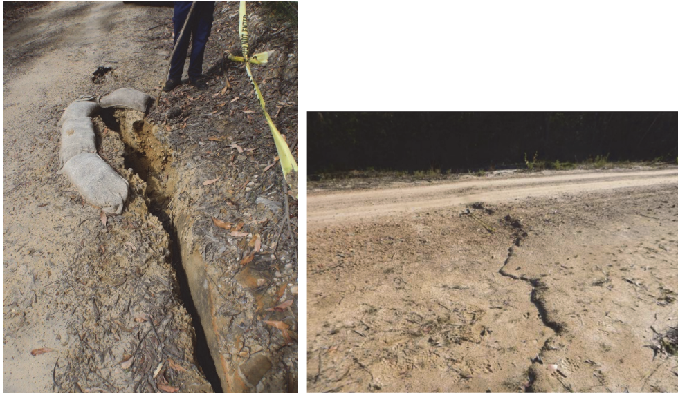
Fig. 6.5 Impacts along the unsealed roads and tracks above LW6 in Area 3A (left side) and above LW11 in Area 3B (right side) (Source: IMC)
