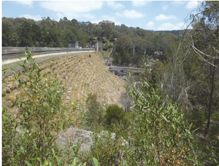
Fig. 6.8 Avon Dam Wall
