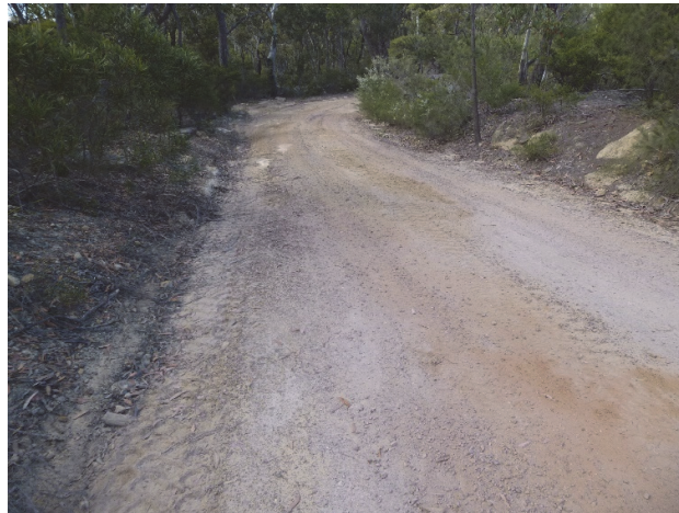
Fig. 6.4 Photograph of a typical track within the Study Area
