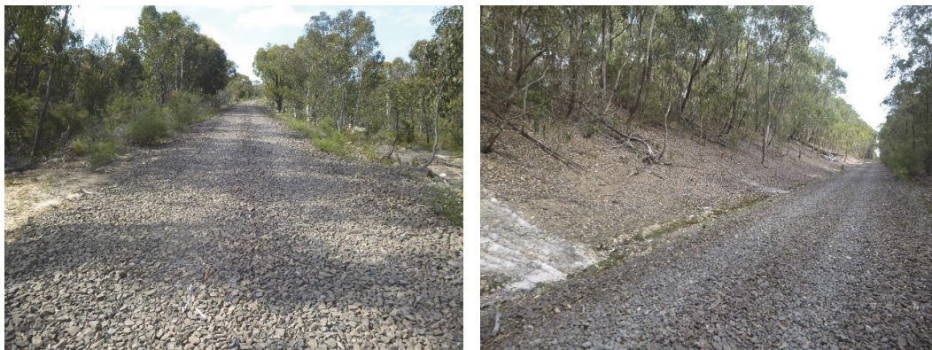
Fig. 6.1 Photographs of the disused railway corridor and cutting
