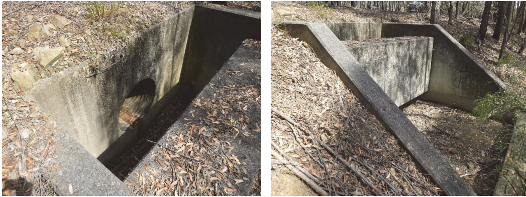
Fig. 6.3 Photographs of drainage culvert
