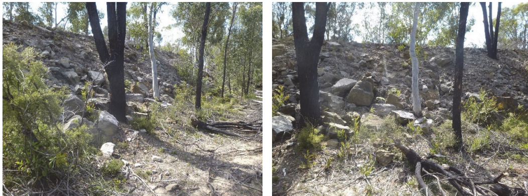
Fig. 6.2 Photographs of the embankment
