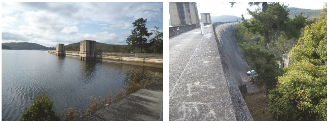
Fig. 6.12 Cordeaux Dam Wall
