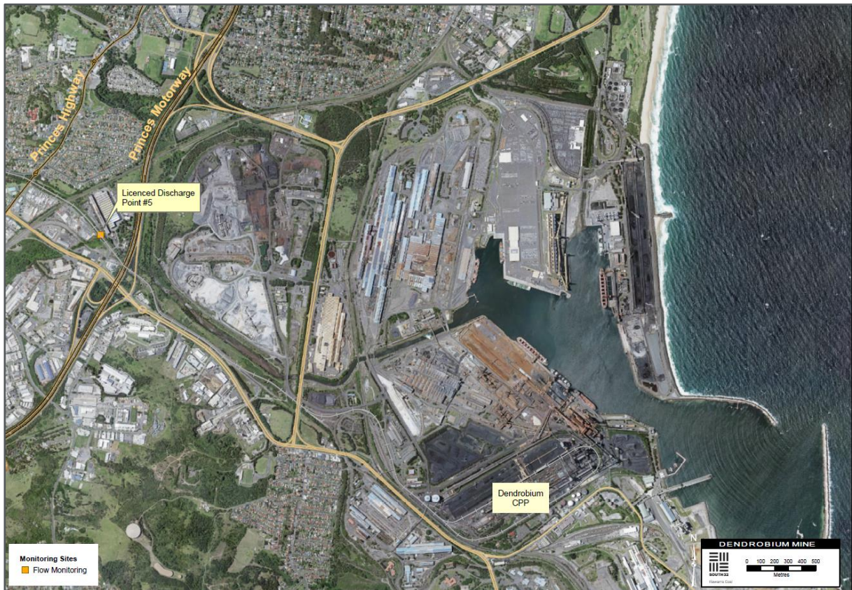
Plate 7-2 – Licensed Discharge Point 5
