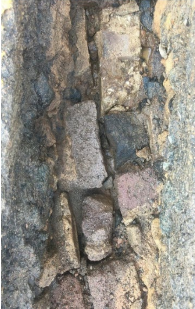
Figure 22: Buried sandstone road surface at Hassall and Priddle Street in Westmead, identified during utility investigation work for the previous Sydney Metro West planning application 29
