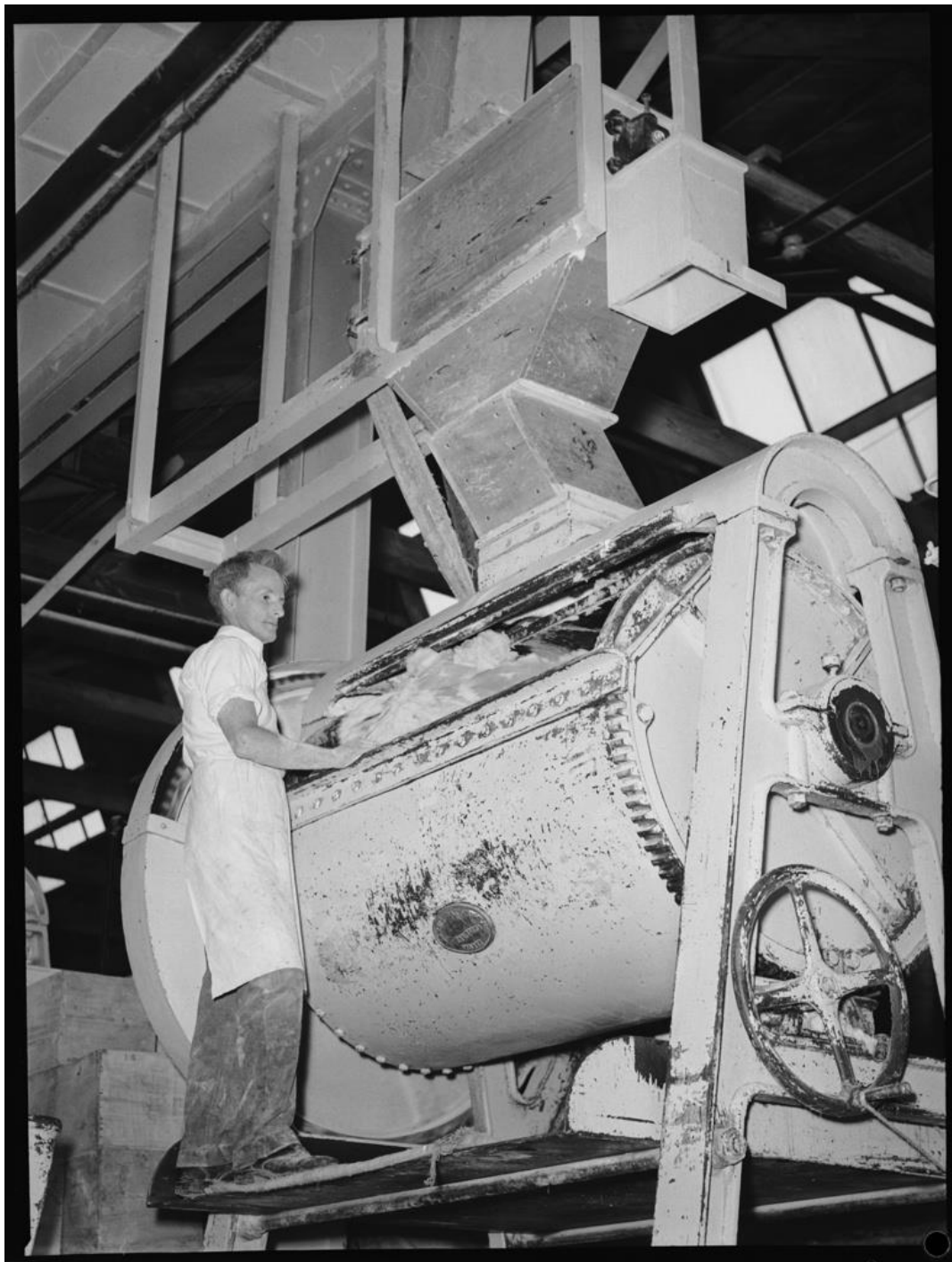
Figure 170. A male Arnott's employee operates a machine used for kneading biscuit dough. Olson, 1938. Source: SLNSW ON 388/Box 031/Item 100.
