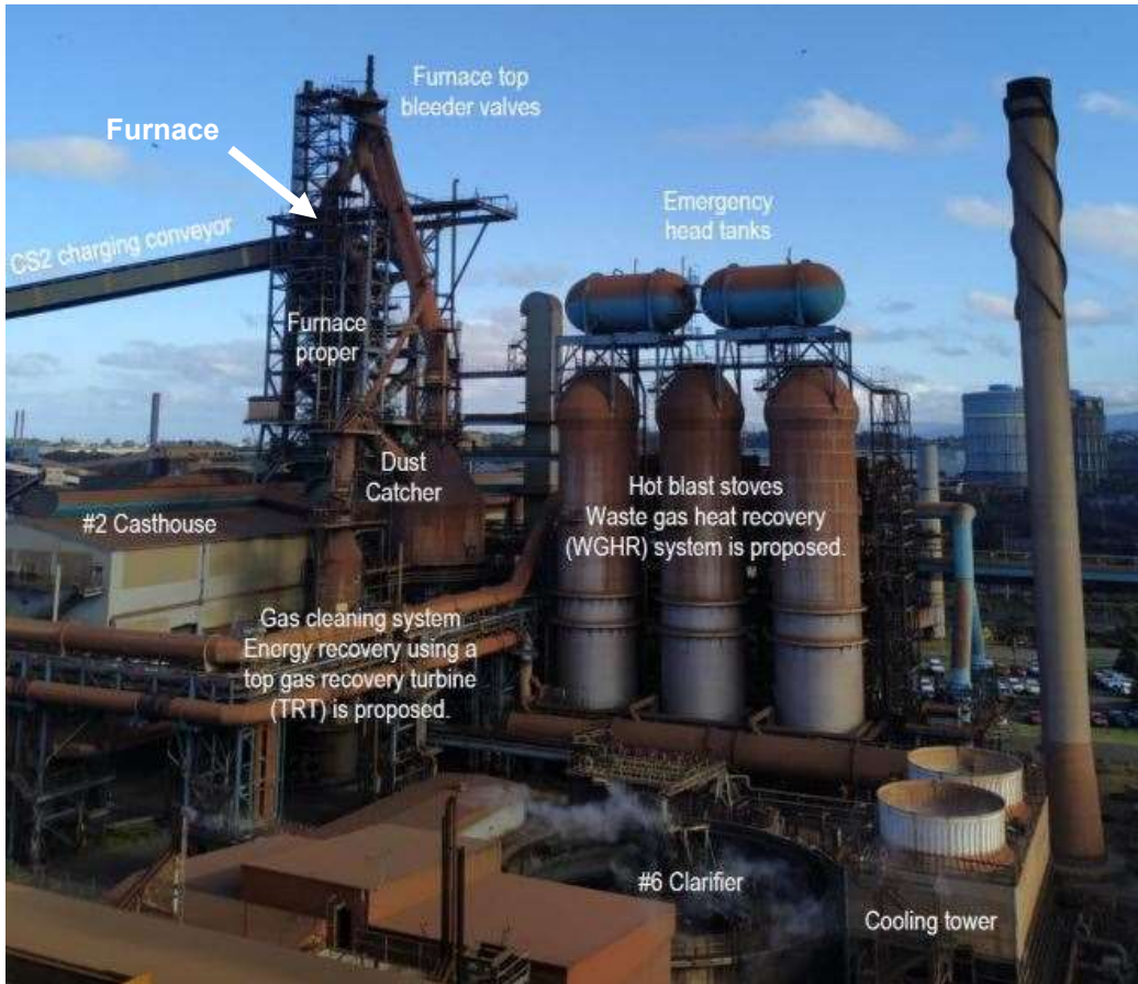
Figure 3 | Key Components of Blast Furnace No.6
