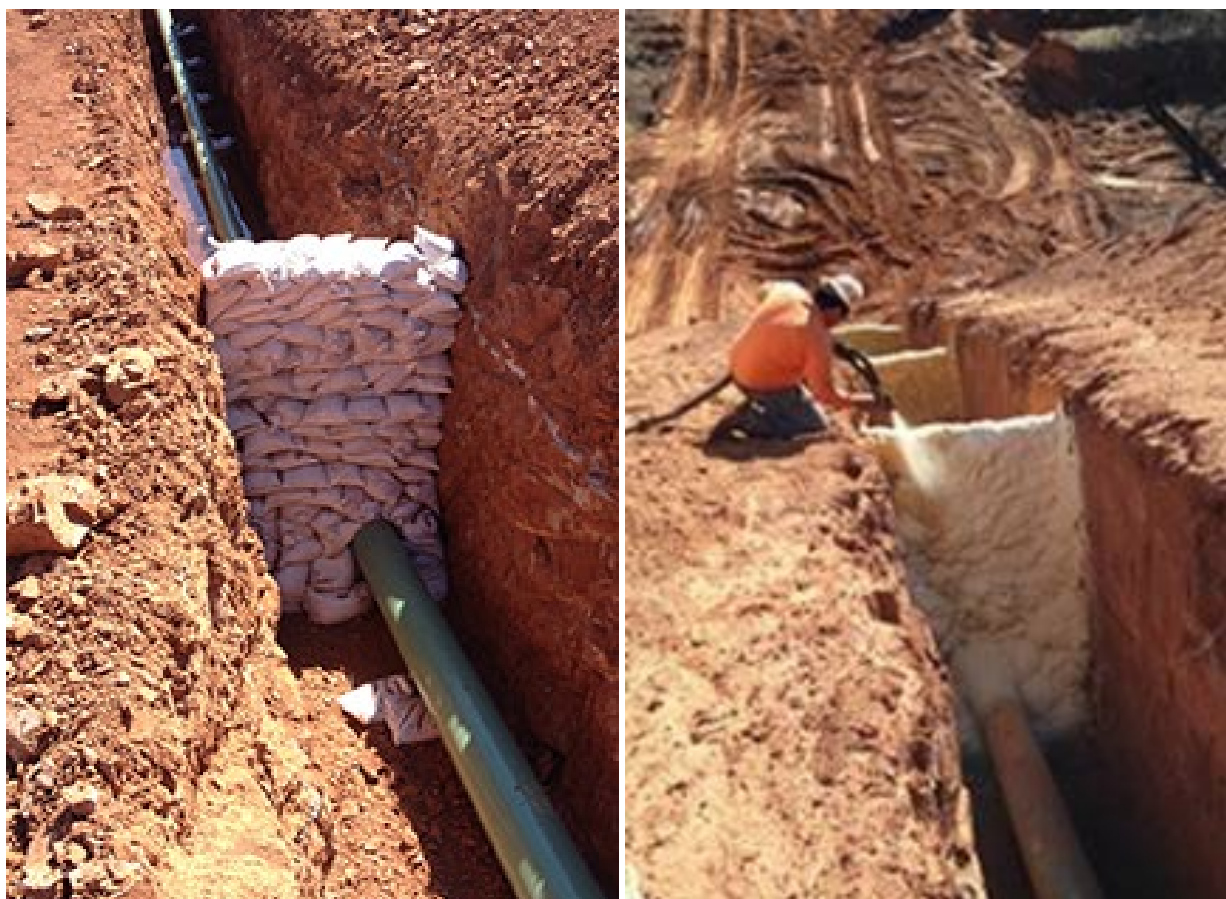
Photo 2.20 Trench breakers
