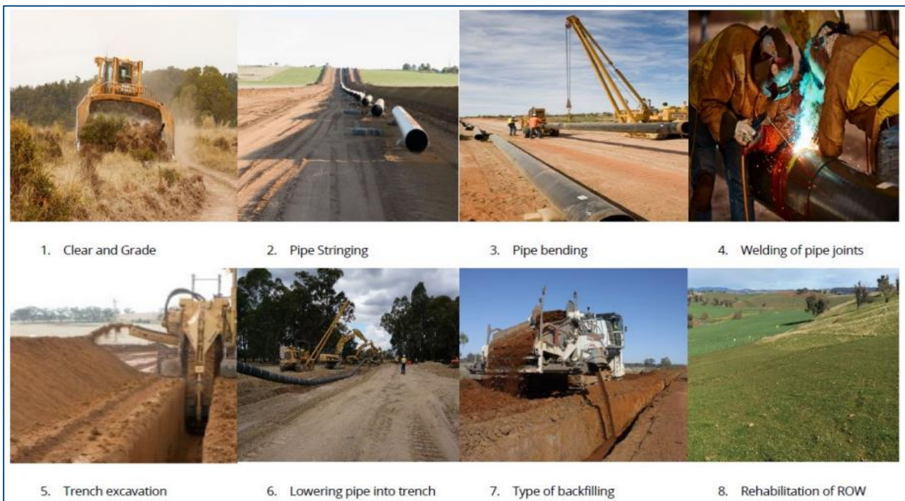
Photo 2.18 Typical construction sequence
