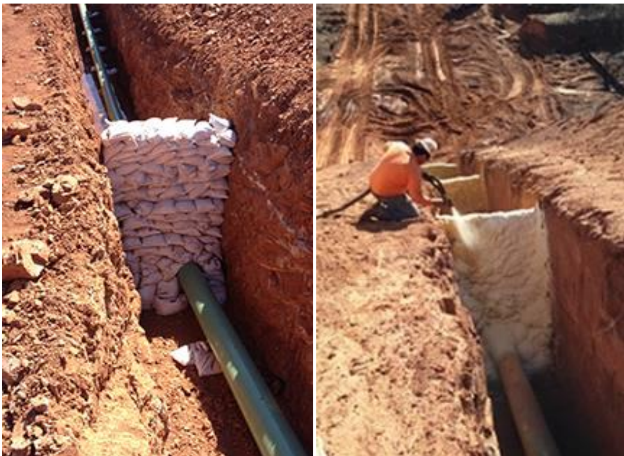
Photo 2.20 Trench breakers
