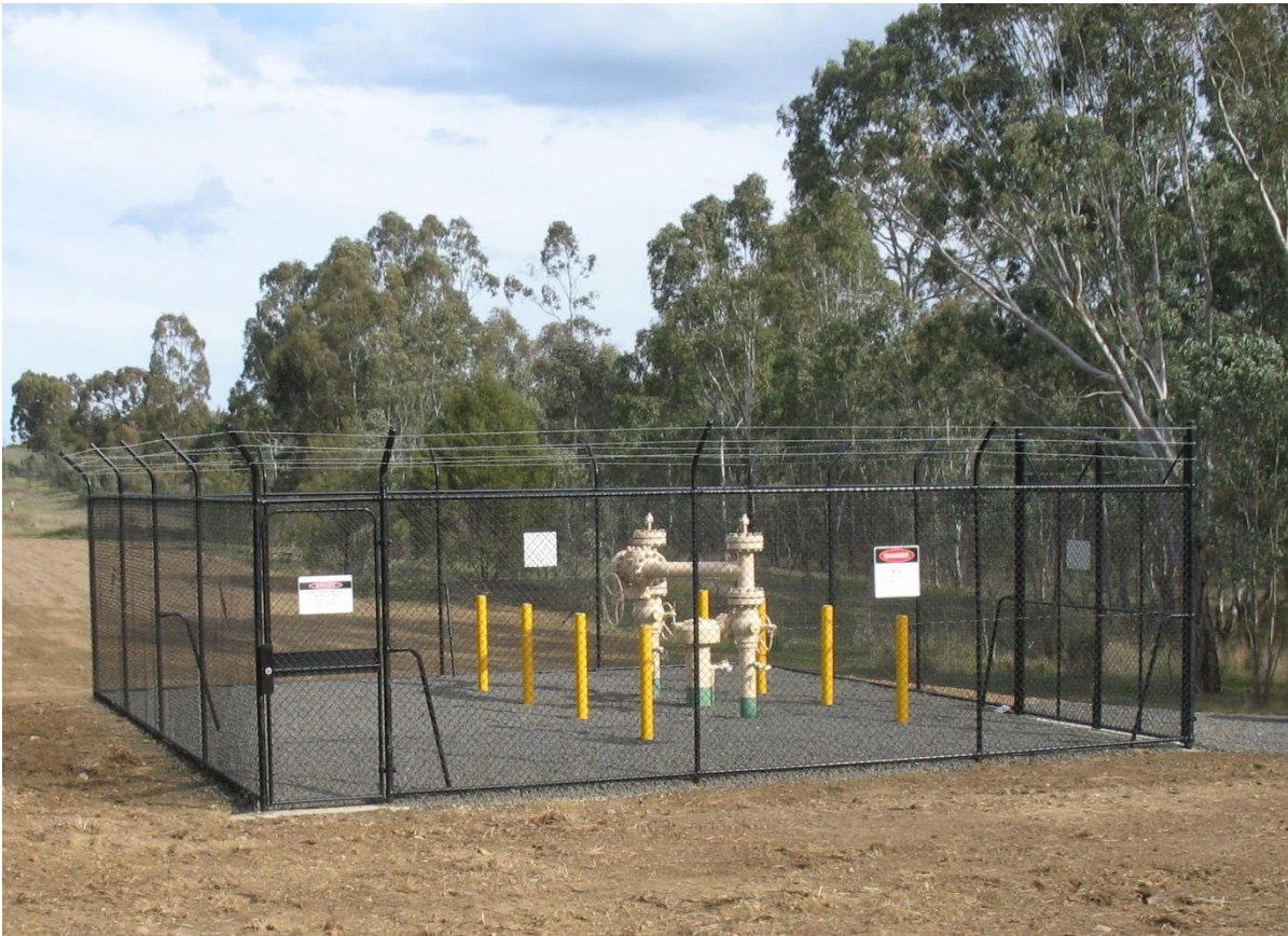
Photo 2.1 Typical Mainline Valve Compound
