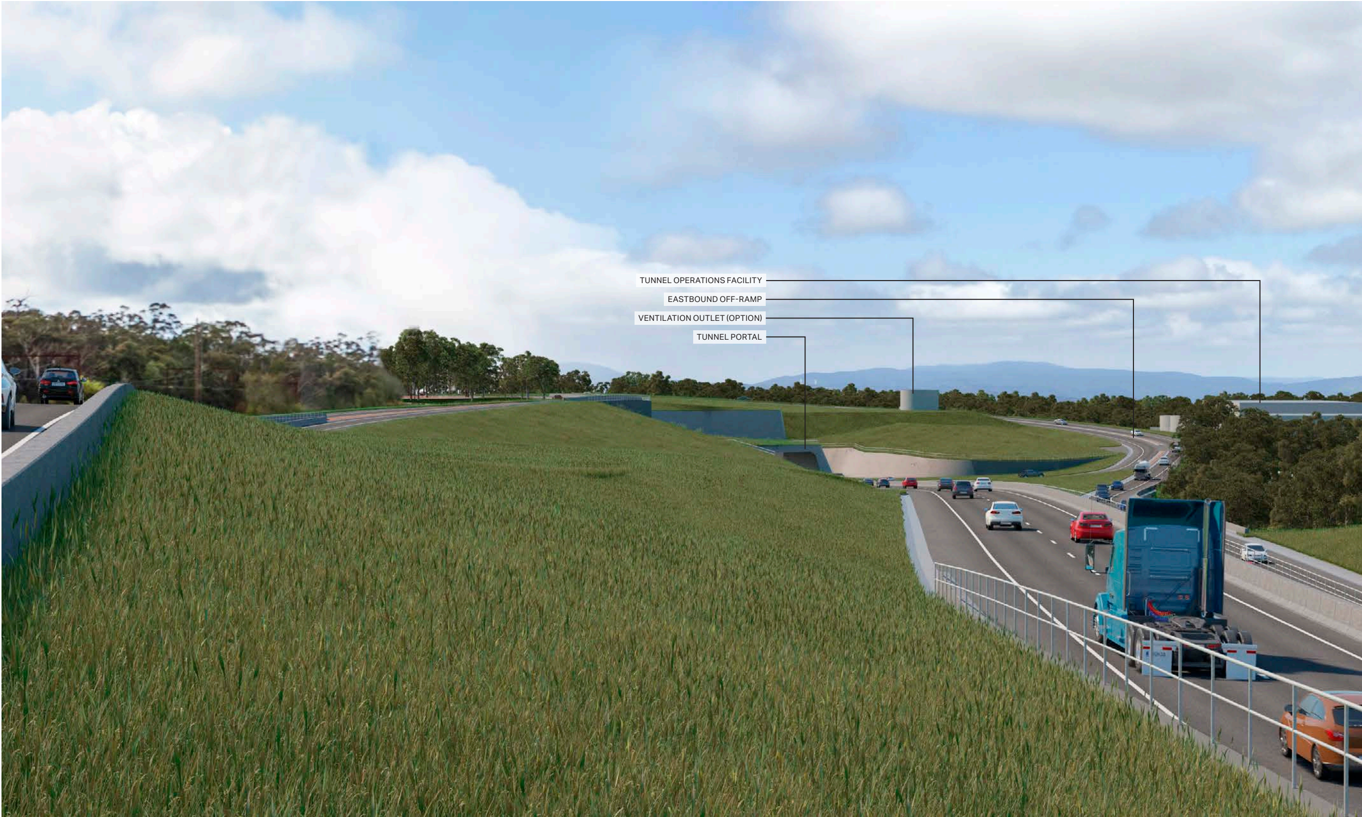
Figure 7-8: Detail of Figure 7-7 showing the project without any tree planting to clearly see infrastructure which would be potentially visible within the view
