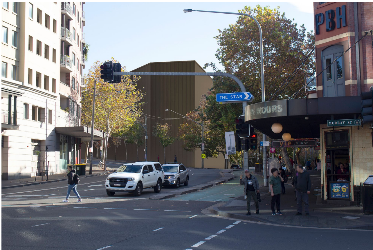
Figure 11-13 Pyrmont Station construction sites - Photomontage from viewpoint 9, west from Pyrmont Bridge, indicative extent of acoustic shed at eastern construction site
