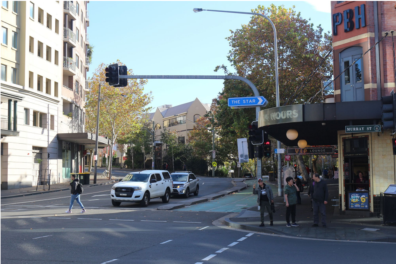
Figure 11-11 Pyrmont Station construction sites - Existing view from Viewpoint 9, west from Pyrmont Bridge
