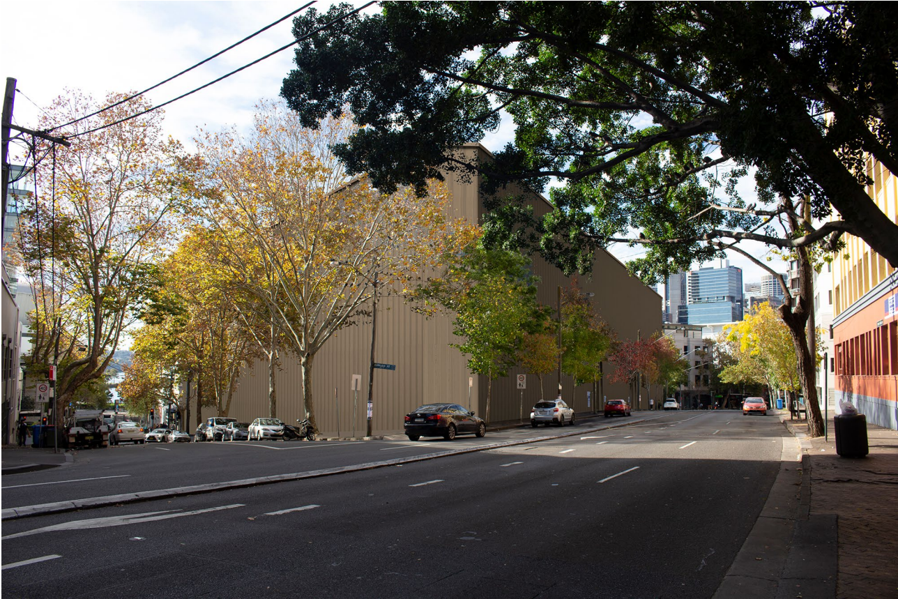
Figure 11-15 Pyrmont Station construction sites - Photomontage from Viewpoint 6, north east along Edward Street and Pyrmont Bridge Road, indicative extent of acoustic shed at eastern construction site
