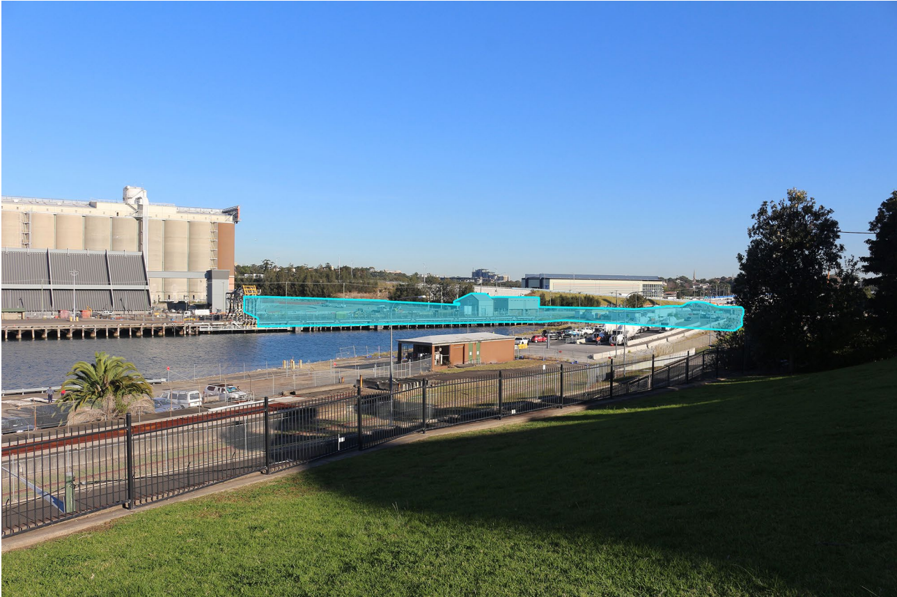
Figure 11-5 The Bays tunnel launch and support site - View from Viewpoint 3, south from Mansfield Street open space, Rozelle, indicative extent of The Bays tunnel launch and support site (shown by blue shading)
