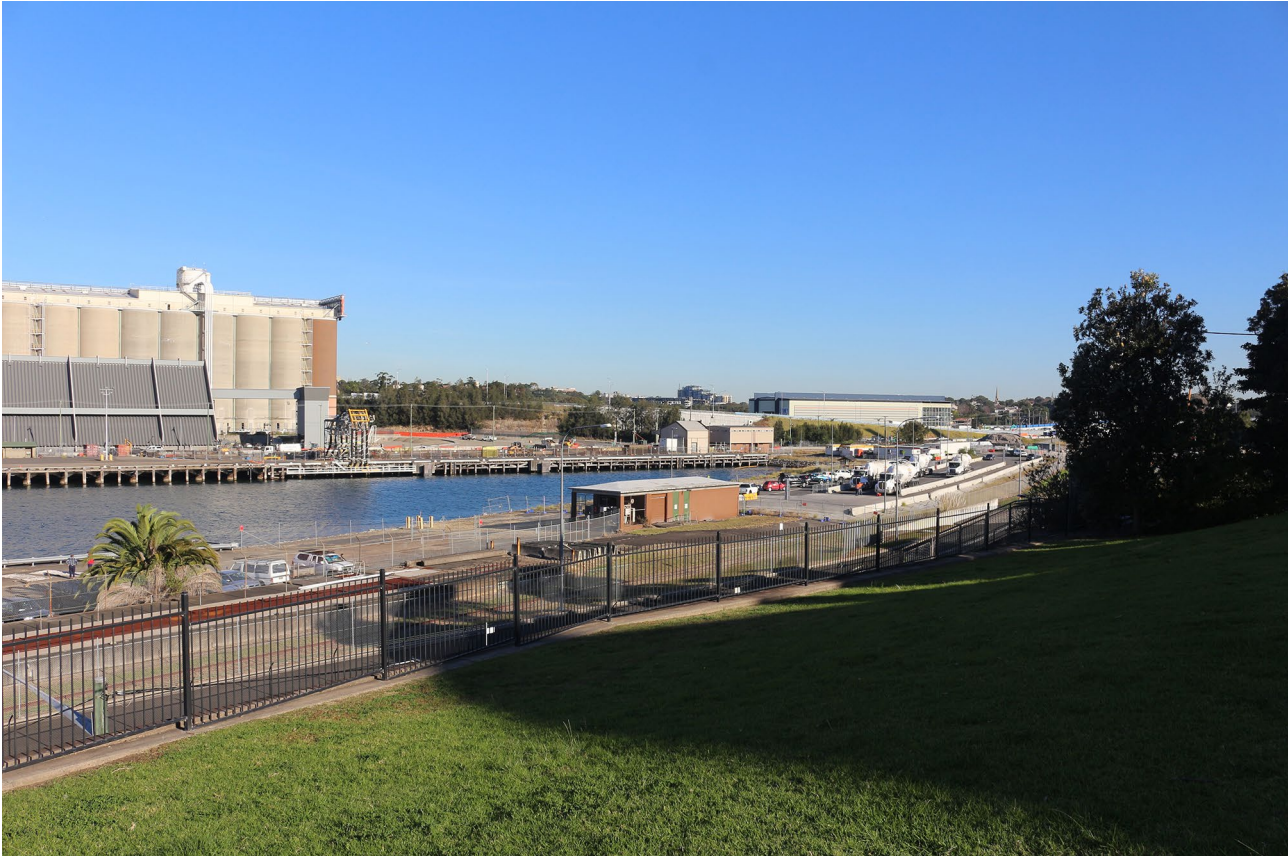
Figure 11-4 The Bays tunnel launch and support site - Existing view from Viewpoint 3, south from Mansfield Street open space, Rozelle
