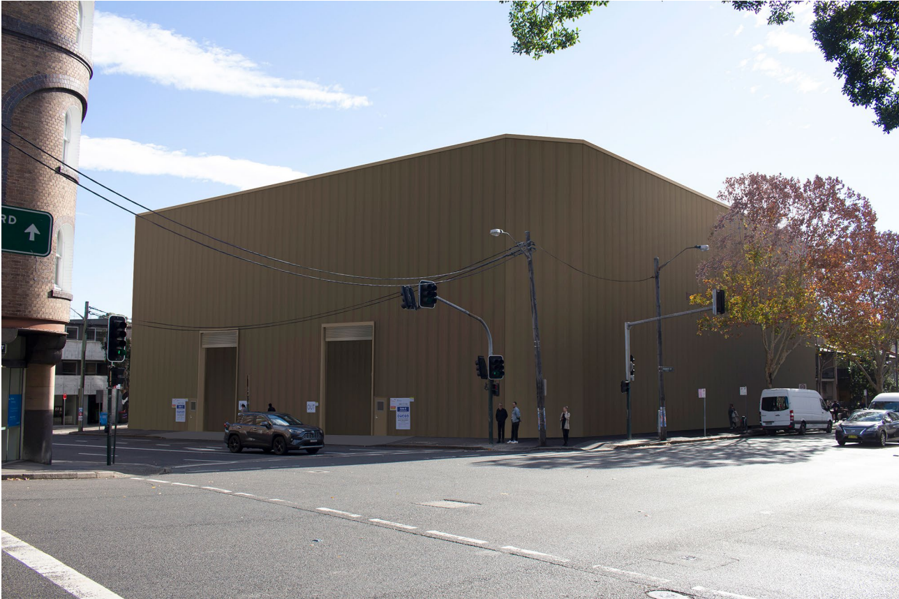
Figure 11-14 Pyrmont Station construction sites - Photomontage from Viewpoint 3, west across the Pyrmont Bridge Road and Pyrmont Street Intersection, indicative extent of acoustic shed at western construction site
