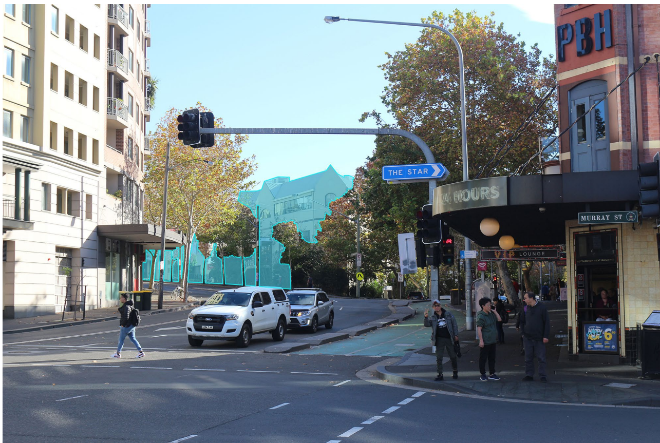
Figure 11-12 Pyrmont Station construction sites - View from Viewpoint 9, west from Pyrmont Bridge, indicative extent of demolition at Pyrmont Station eastern construction site (shown by blue shading)
