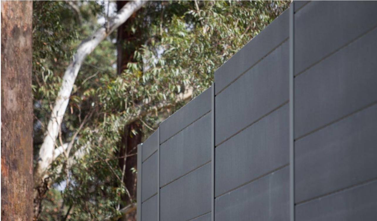
Figure 4 Hebel Wall Noise Barrier at the Cheltenham Services Facility Site
