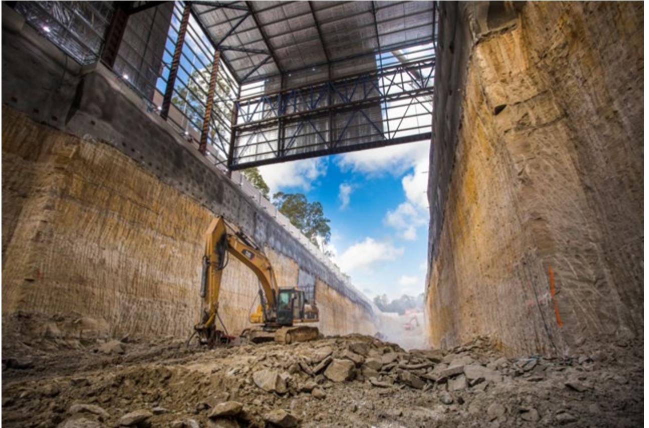
Figure 3 Spoil and Excavation Works at the Showground Site
