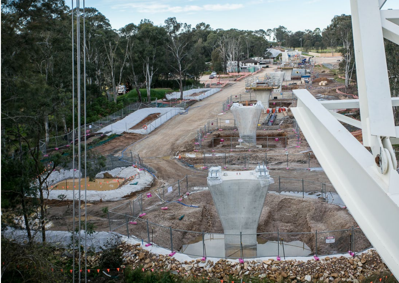
Figure 7 Erosion and Sediment Controls at the Cudgegong Road Site
