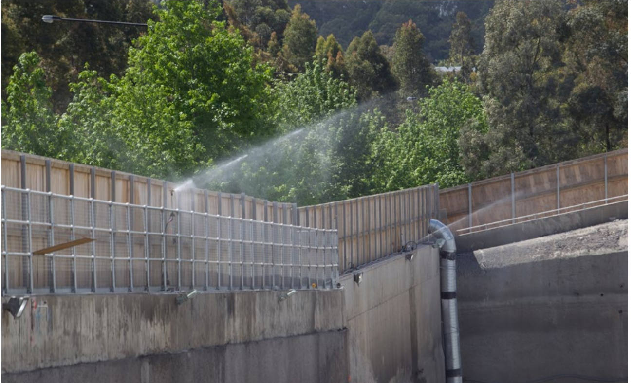
Figure 8 Dust Mitigation at Northwest Station Site
