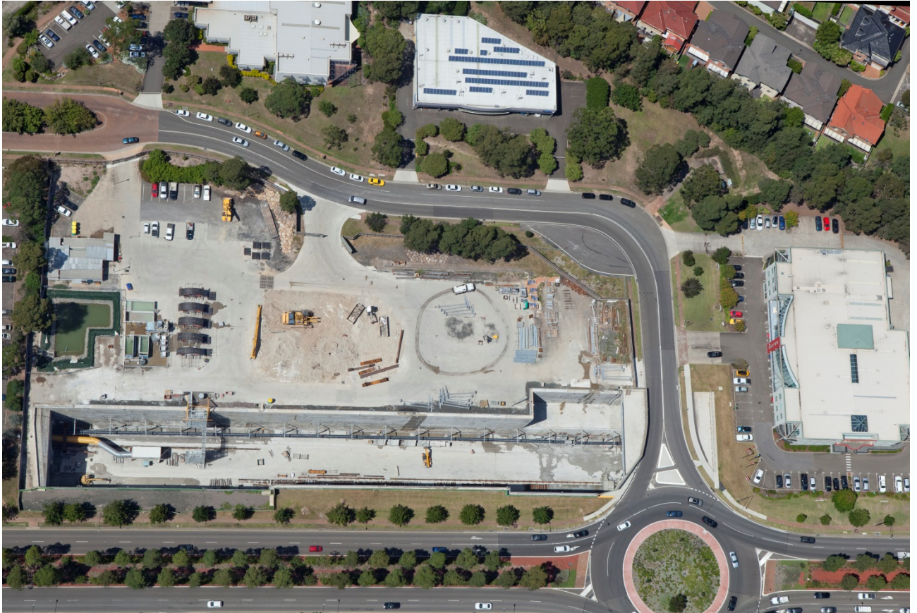
Figure 2 Aerial View of the Sydney Metro Northwest Station Site
