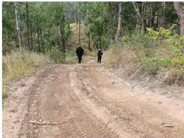
Plate 7.4 Example of the access track that runs broadly parallel with the Macleay River, view east. As demonstrated, the access track has been cut into the hillslope, and recently graded
