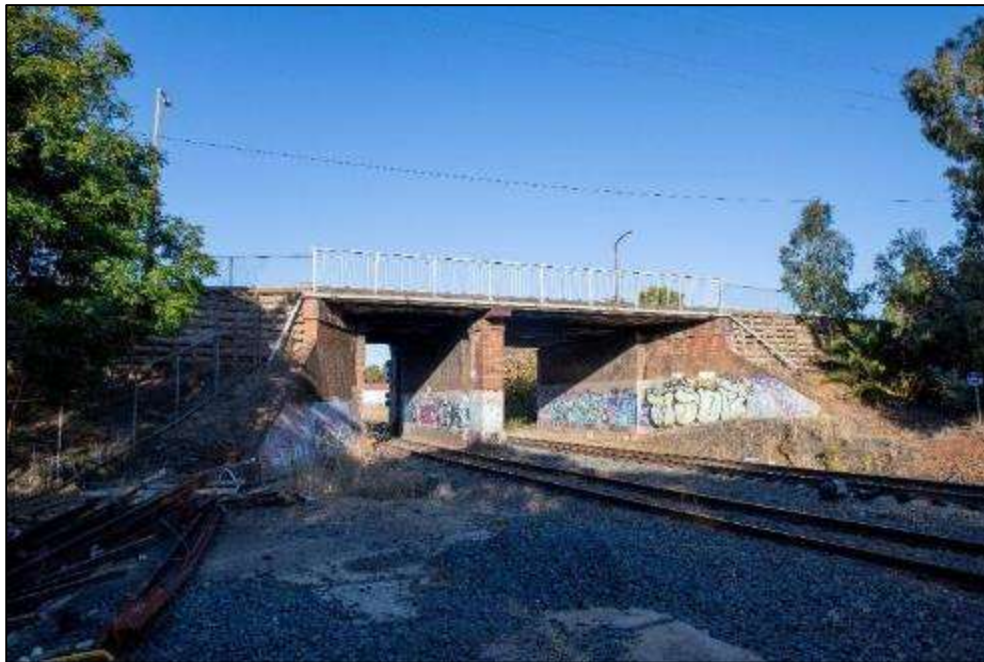
Figure 6-15: Edmondson Street Bridge brick abutments. Source: OzArk 2024.
