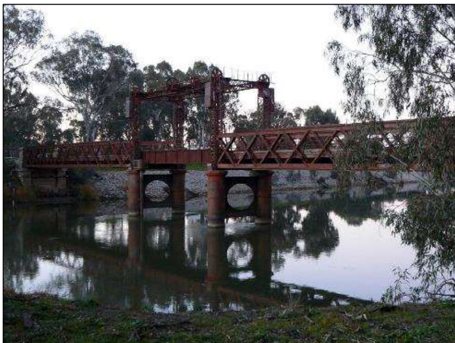
Figure 4-13: Comparative heritage rail bridge at Tocumwal featuring oval shaped perforations. Source: Wikipedia.
