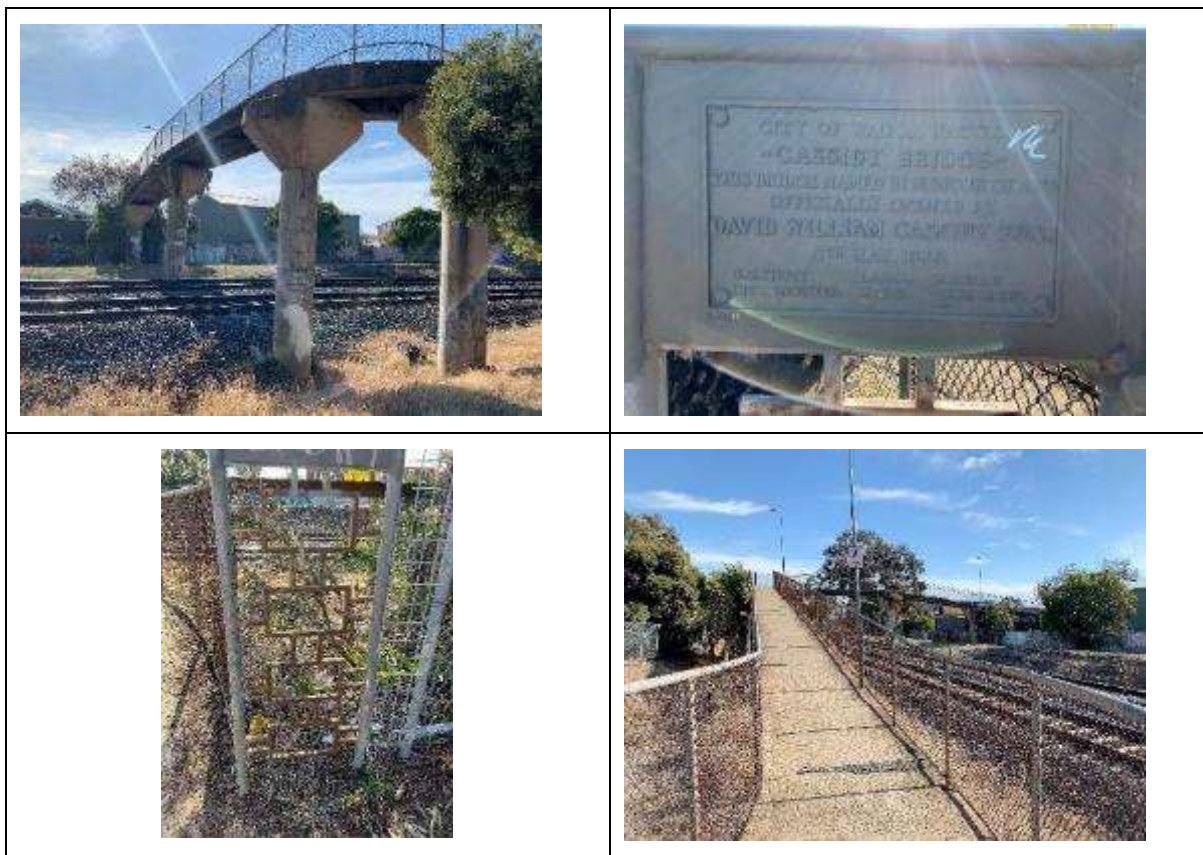
Figure 6-12: Field photos of Cassidy Bridge. Source: OzArk2024.
