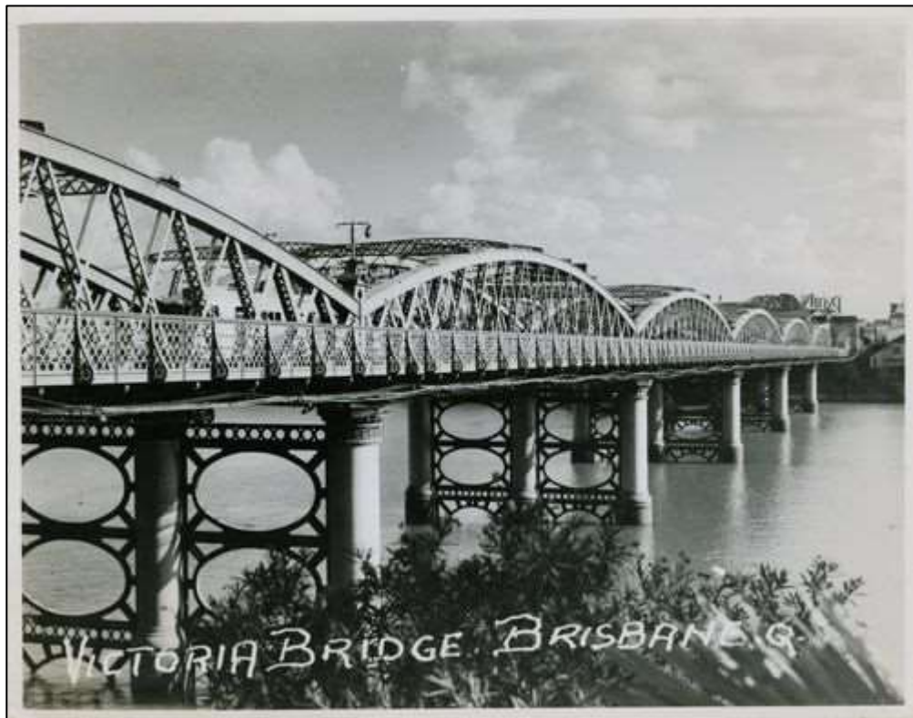
Figure 4-14: Comparative heritage rail bridge with oval and circle perforations. Victoria Bridge, Brisbane. Source: The University of Queensland.
