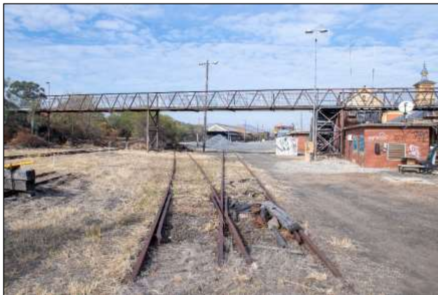
Figure 4-30: Existing Warren Truss pedestrian bridge. Source: OzArk 2024.
