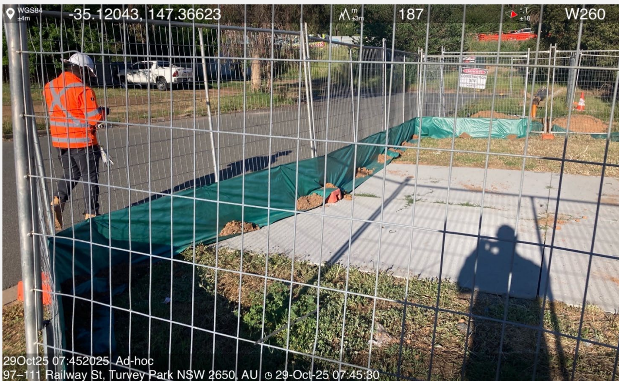
Site compound – OBS 02
