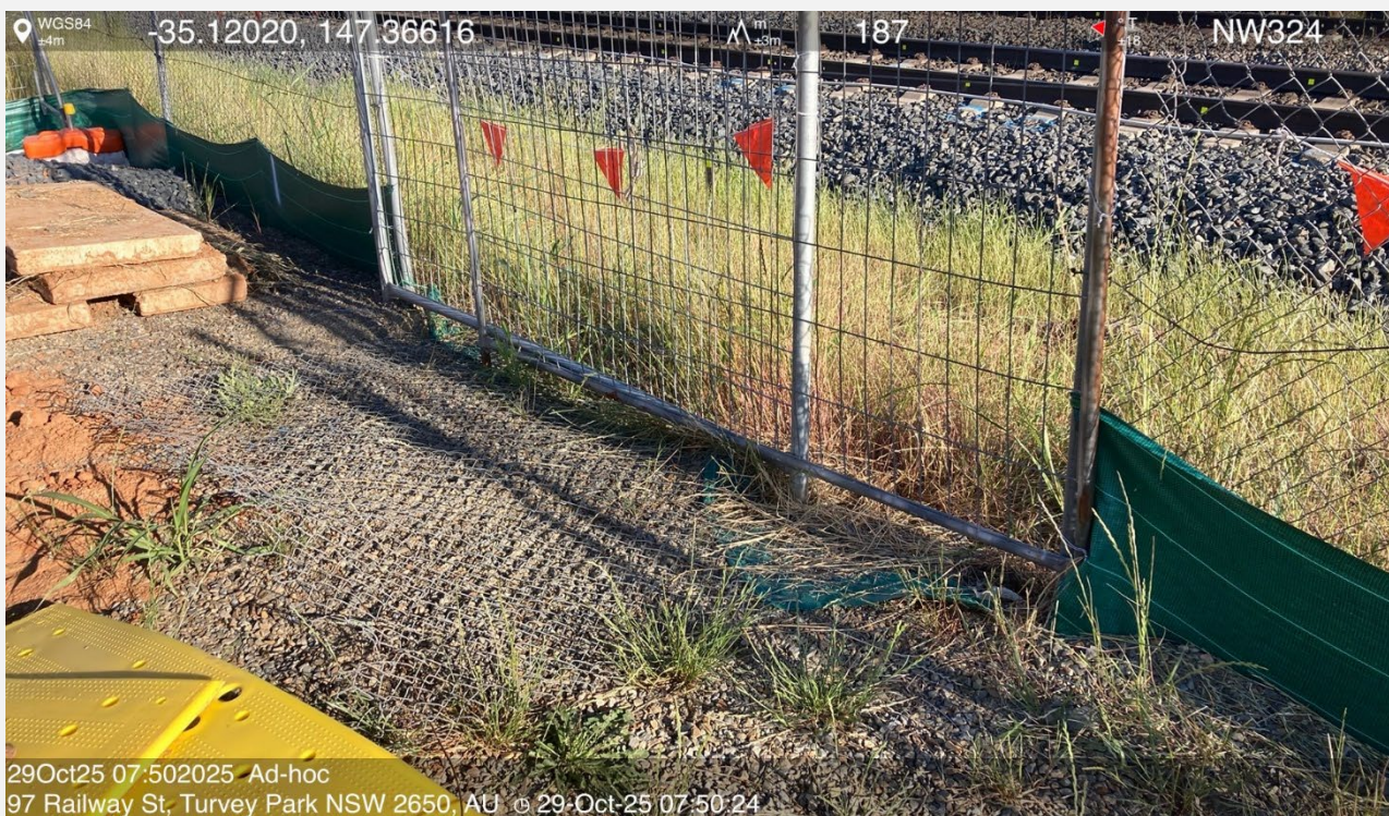
Site compound access to the corridor – OBS 02
