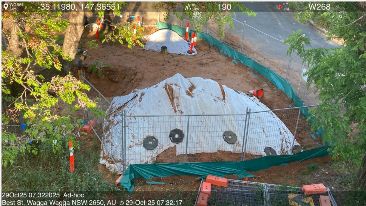
Gas main works compound, Edmonson Bridge – OBS 01
