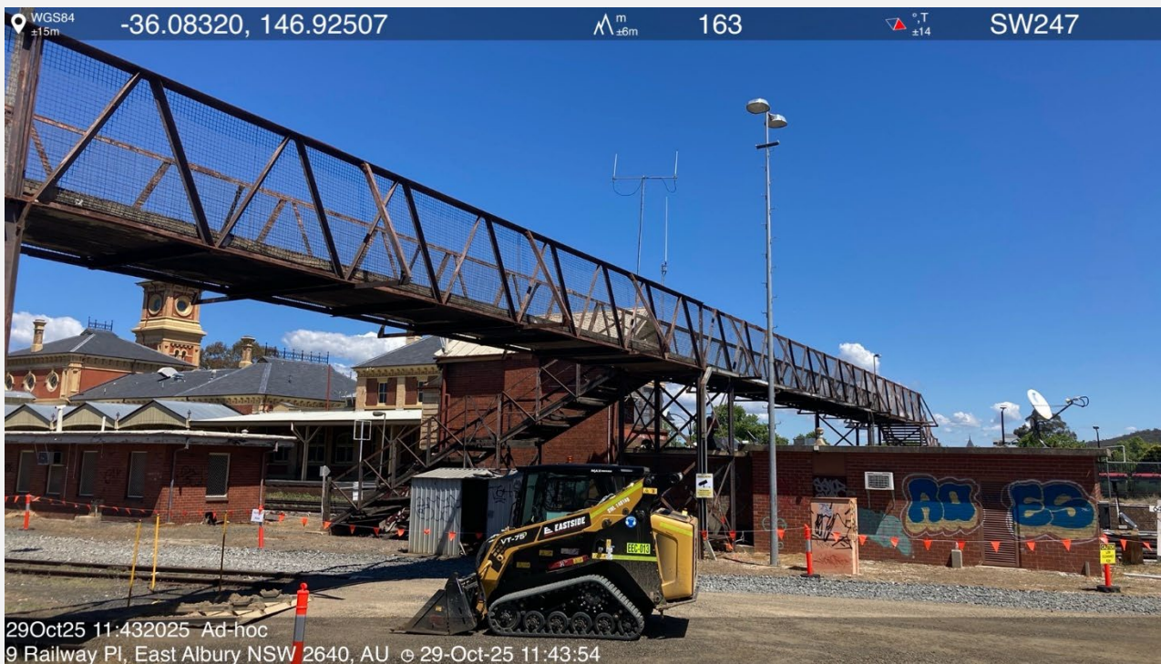
Heritage pedestrian bridge
