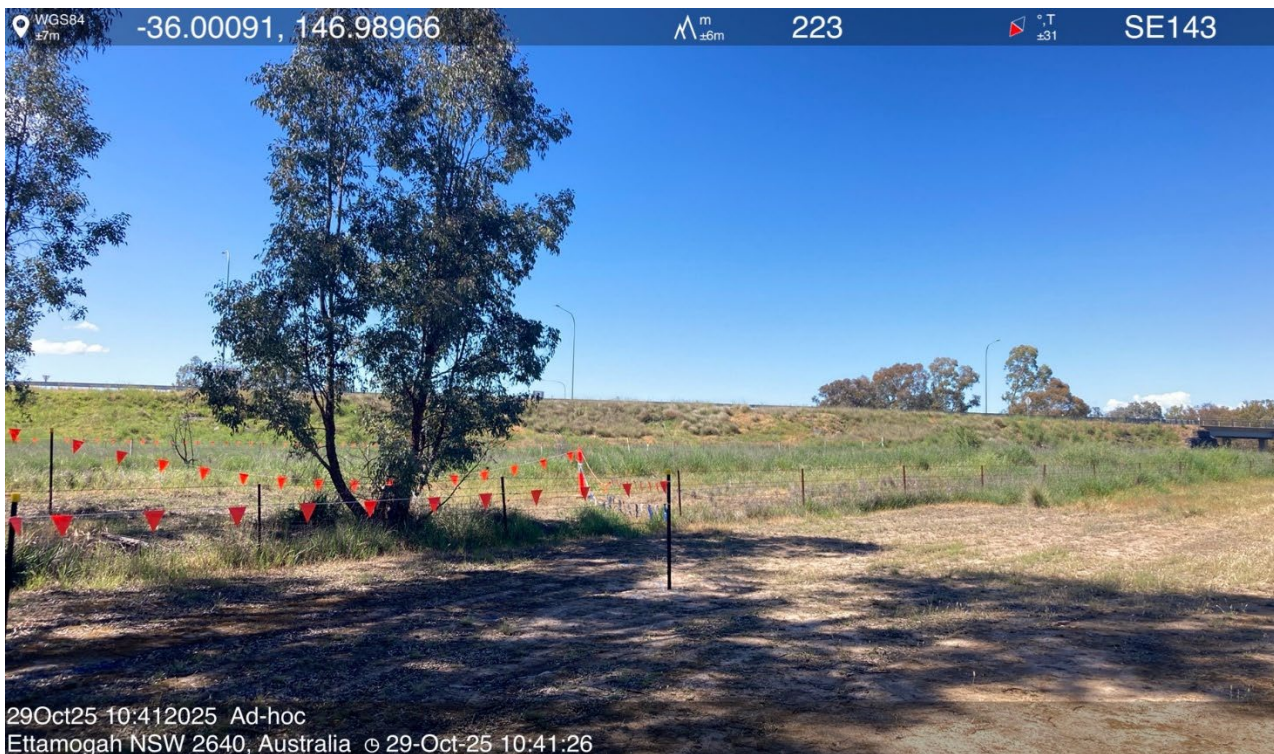
Clearing and CIZ flagging demarcation
