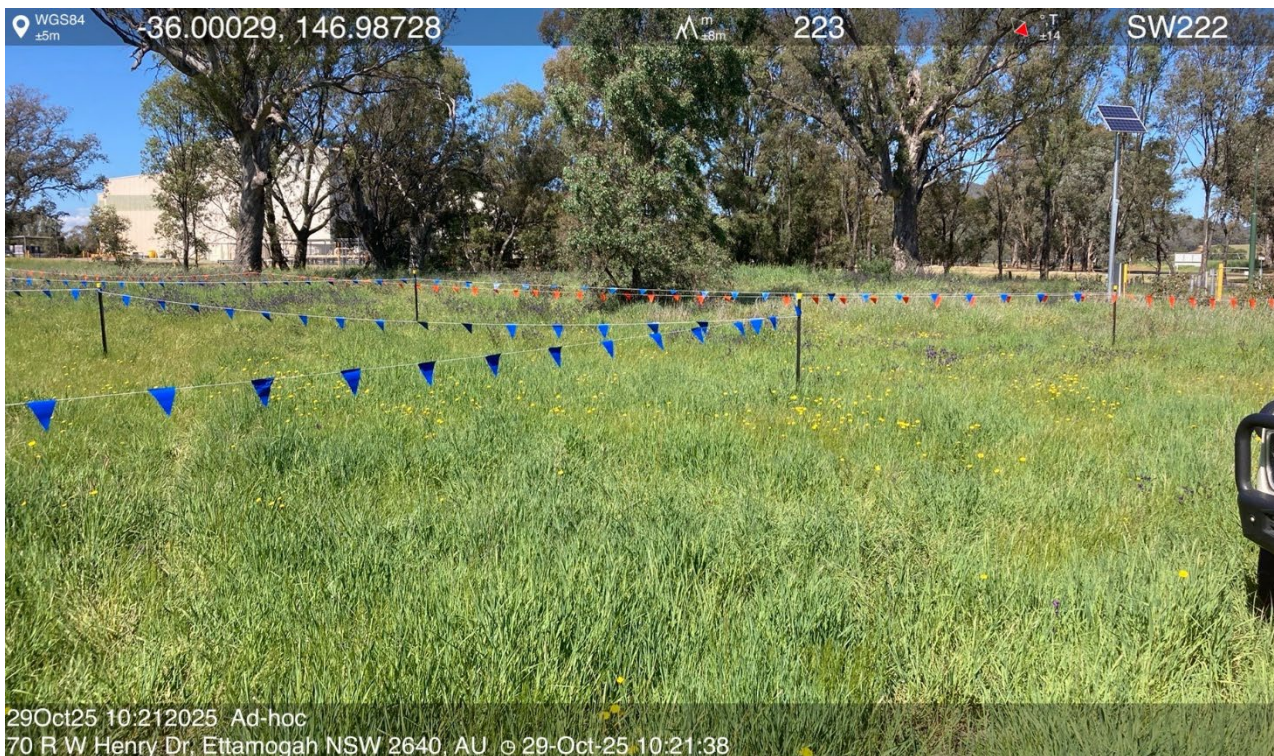
Clearing and CIZ flagging demarcation
