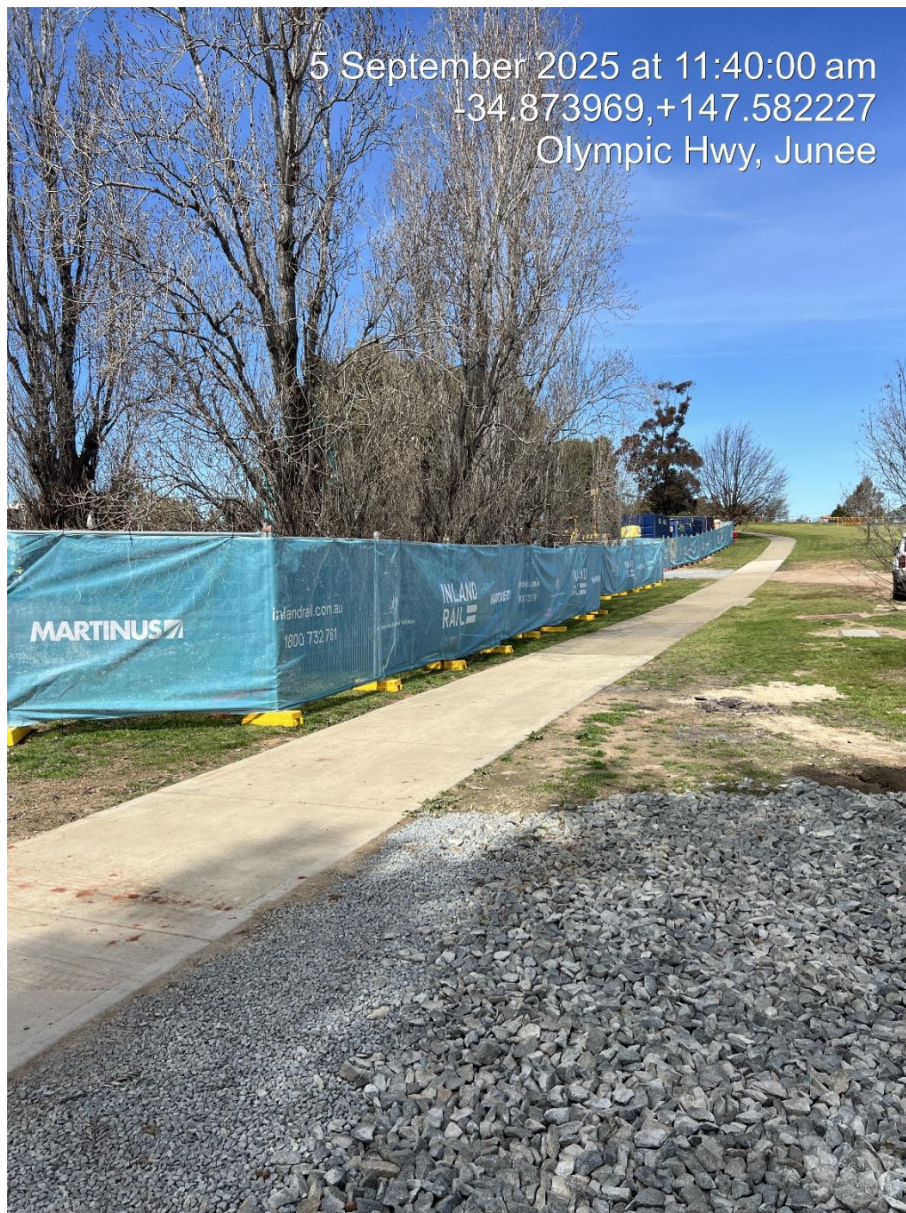
FIGURE 7 Rail exclusion fencing in place on the western side of the rail corridor looking south from the existing boundary fencing along Seignior Street
