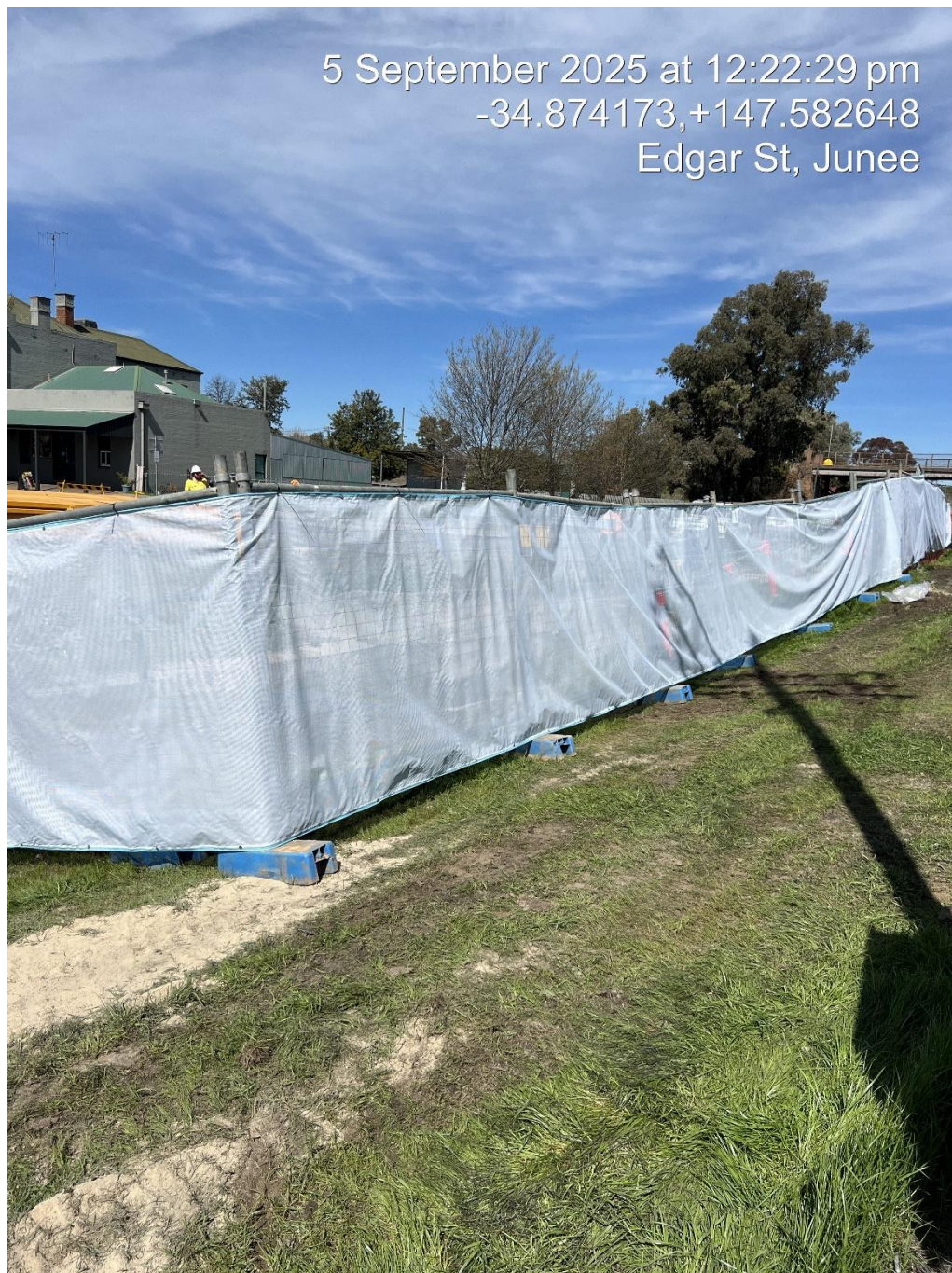
FIGURE 6 RAIL EXCLUSION FENCING IN PLACE ON THE EASTERN SIDE OF THE RAIL CORRIDOR LOOKING SOUTH FROM THE REAR BOUNDARY OF THE AQUATIC CENTRE
