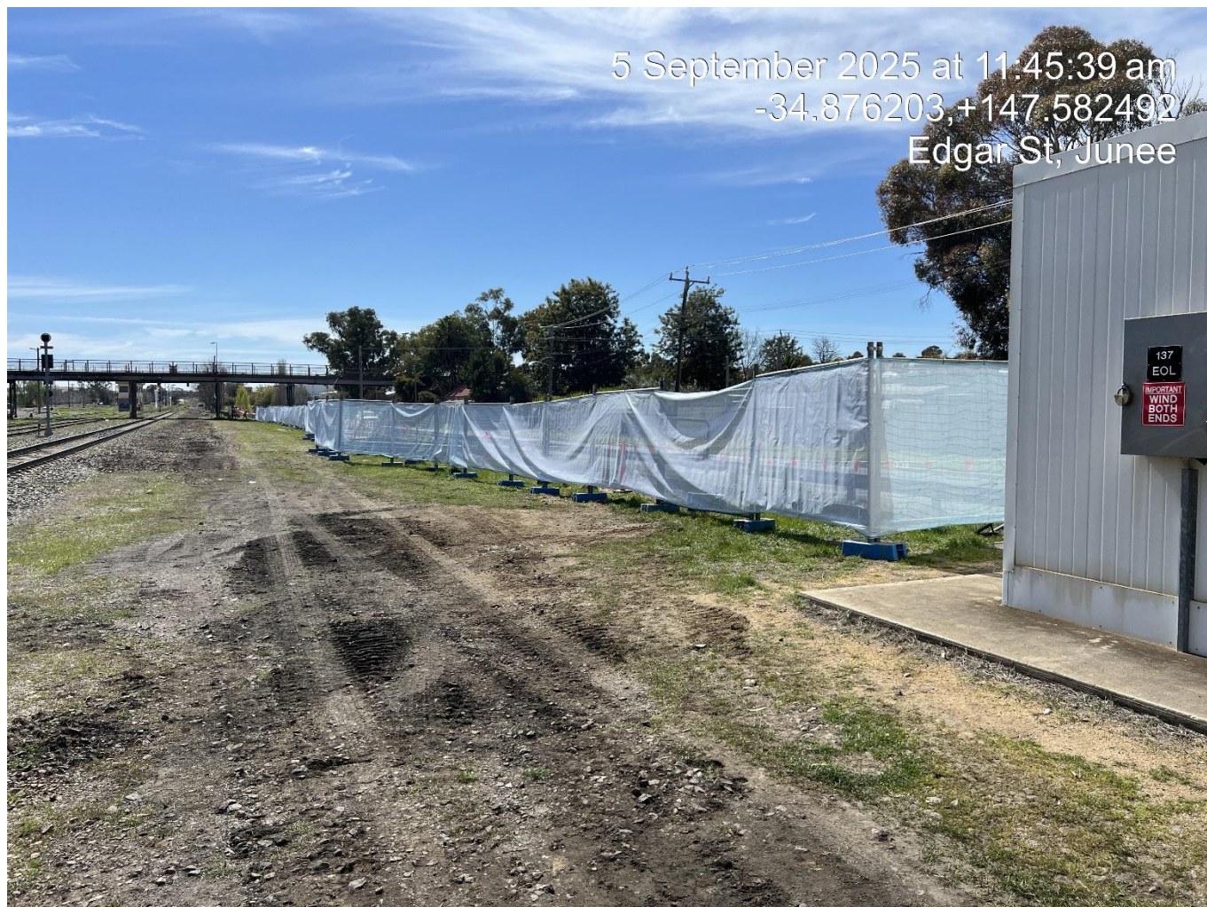
FIGURE 5 Rail exclusion fencing in place on the eastern side of the rail corridor extending north from William Street along Edgar Street
