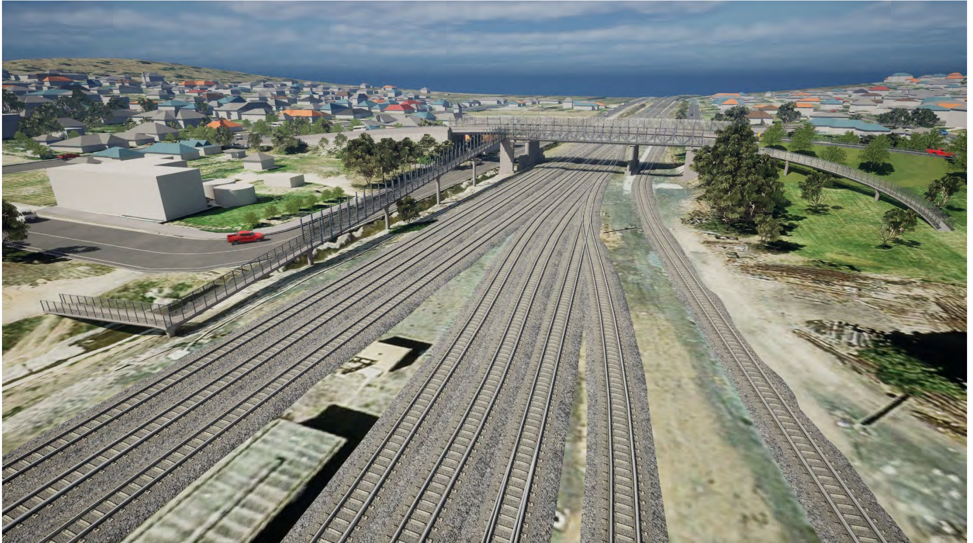
FIGURE 3-5 KEMP STREET BRIDGE (FACING SOUTH)
