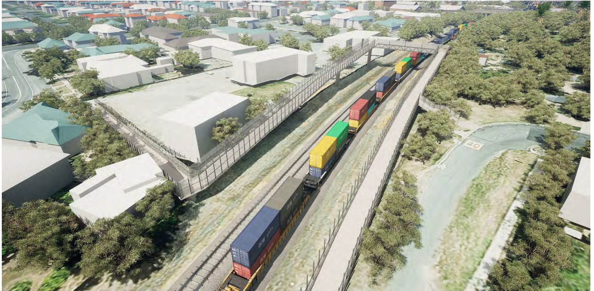
FIGURE 3-2 CASSIDY PARADE PEDESTRIAN BRIDGE (FACING NORTH-EAST)
