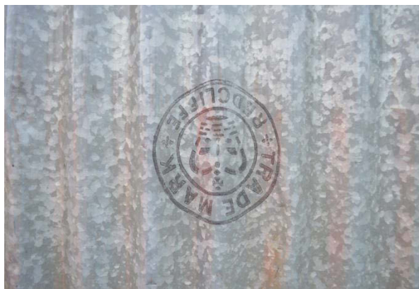
Figure 25 The original corrugated iron sheets have been stamped with a trademark.
