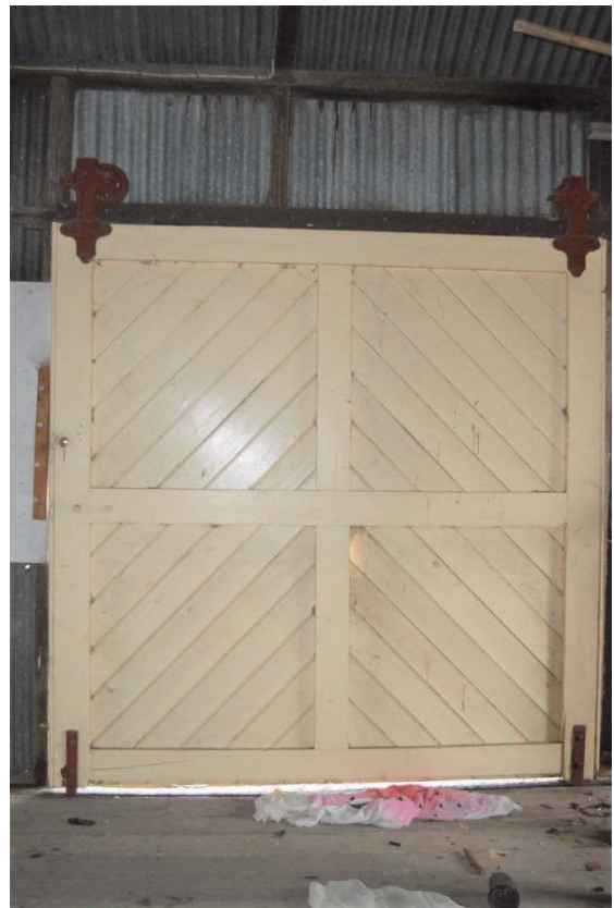
Figure 23 Two of the four sliding doors. Note the slight difference in construction and castors.
