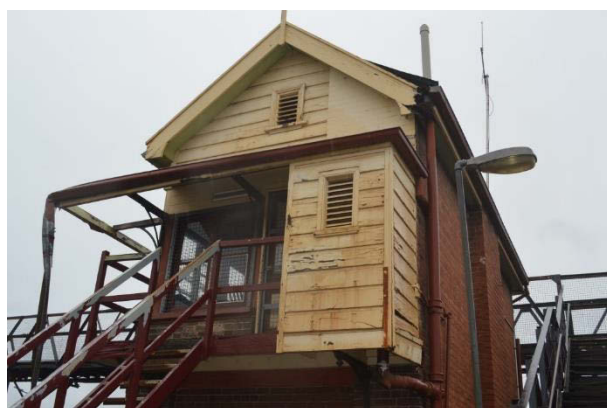
Figure 5 The timber work shows signs of deterioration.
