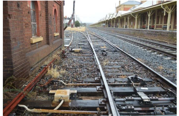
Figure 6 The switching gear housed in the operating level and its external connection to the railway tracks appears to be intact.
