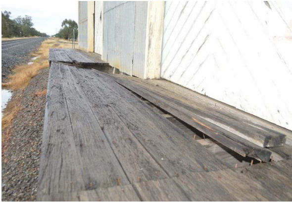
Figure 19 The track side platform has deteriorated.
