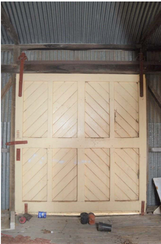
Figure 23 Two of the four sliding doors. Note the slight difference in construction and castors.
