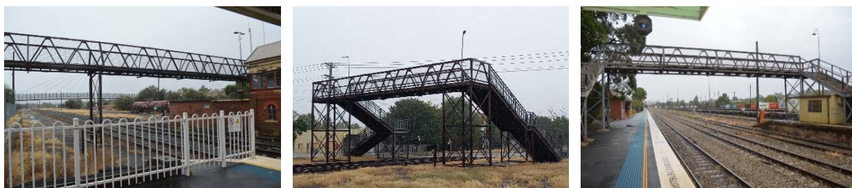
Figure 4.29 The Warren truss footbridges at Albury (1910, left), Culcairn (1920, centre) and Junee (1919, right).
