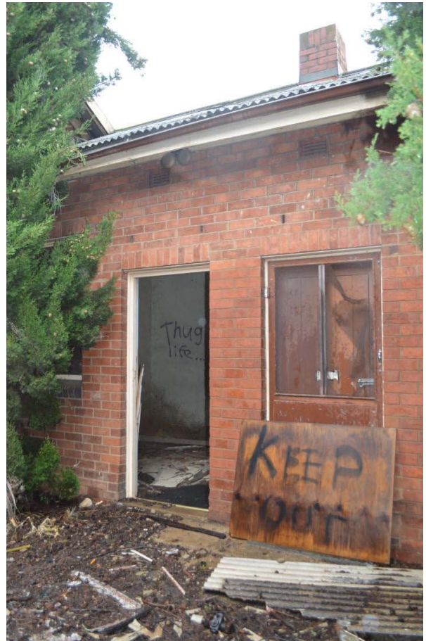
Figure 50 Both buildings are in poor condition, with evidence of vandalism and squatting.
