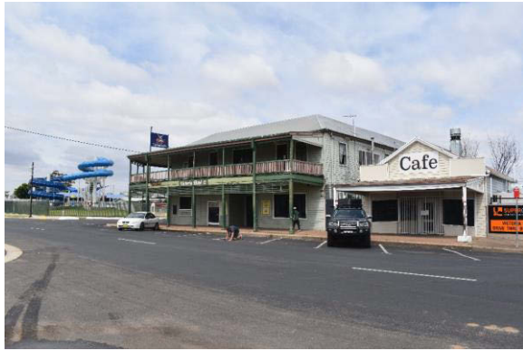
Figure 4-33: The locally listed heritage item of Victoria Hotel at 339 Gosport Street, Moree
