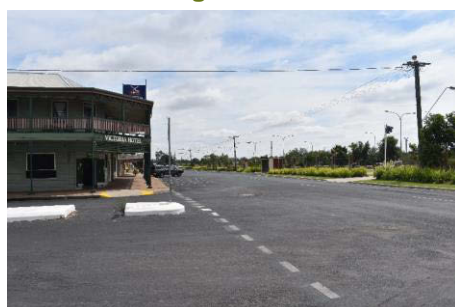
Figure 5-7: View of the southern elevation of Victoria Hotel with the CIZ in the background. Source: Artefact Heritage
