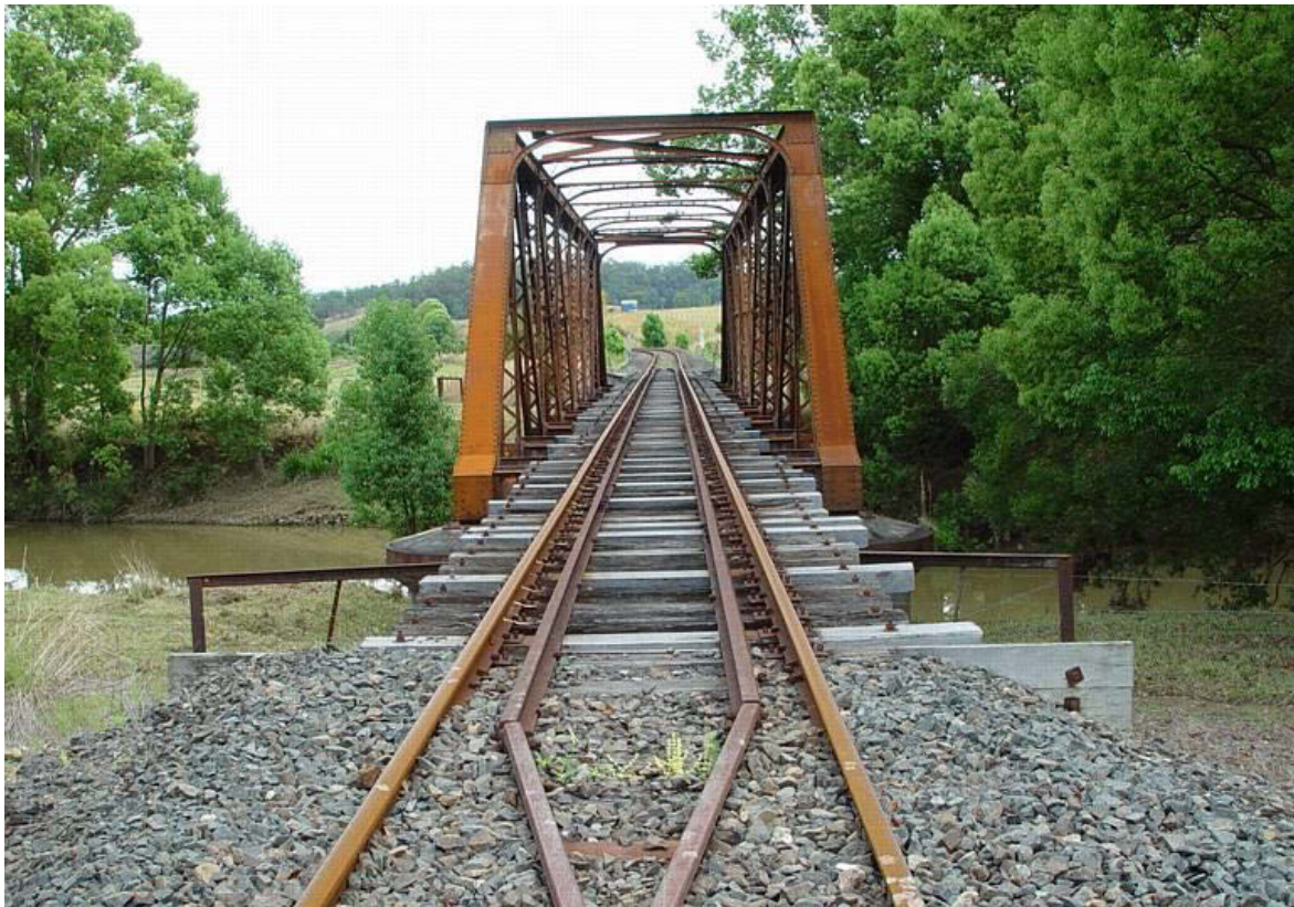
Figure 3-12: The 1894 steel Pratt truss bridge over Dunbible Creek design (CRIA, n.d. in Heritage NSW, DPC 2005)
