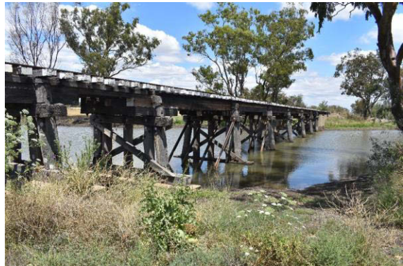
Figure 4-14: The 13 span timber and concrete constructed underbridge over Duffy's Creek at Chainage 667.21
