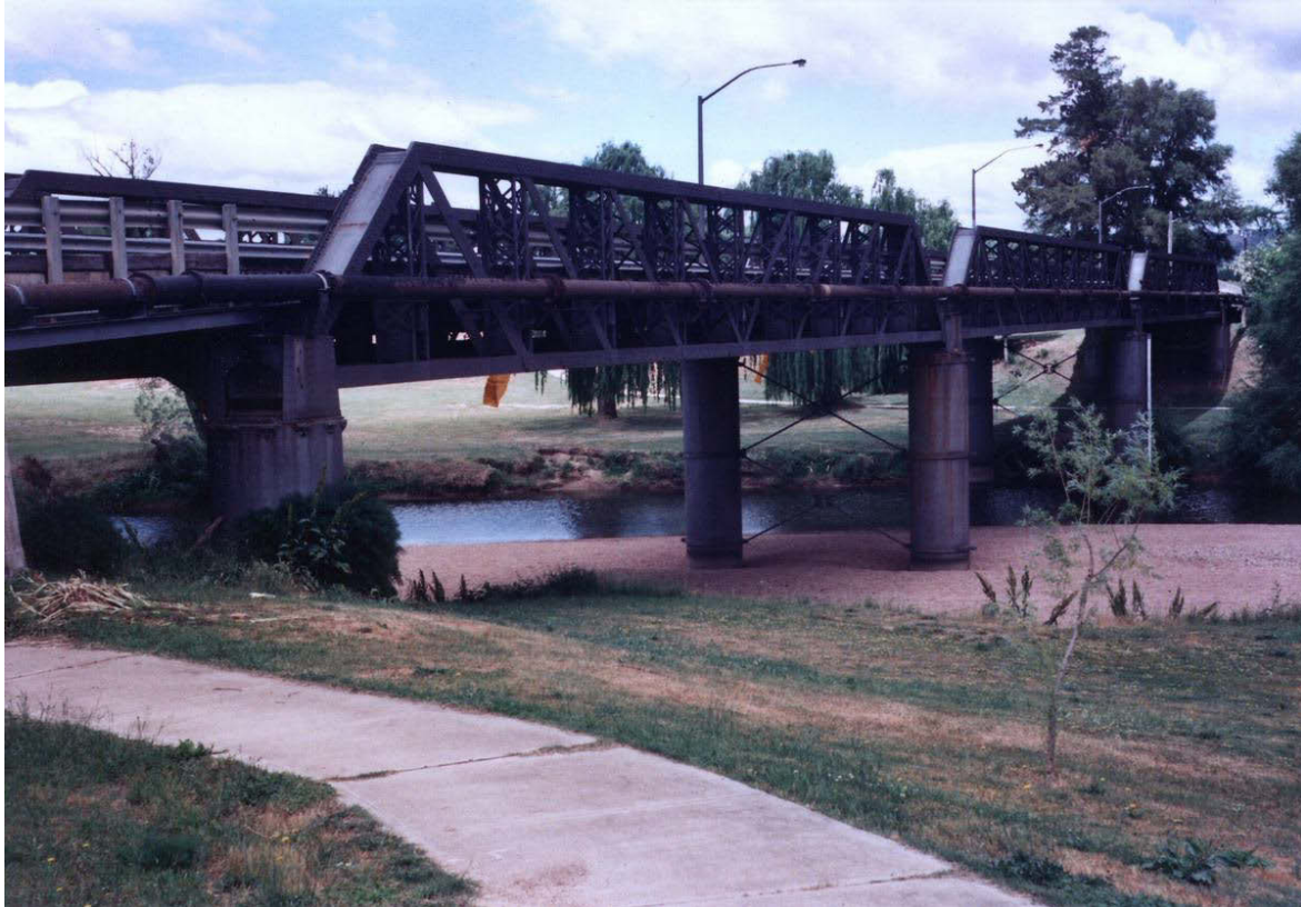
Figure 3-12: The 1894 steel Pratt truss bridge over Dunbible Creek design (CRIA, n.d. in Heritage NSW, DPC 2005)
