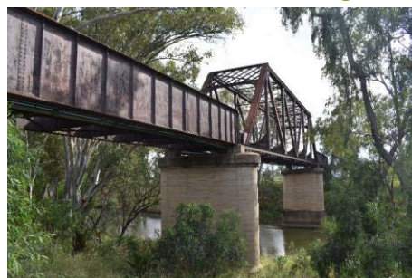
Figure 5-1: Mehi River Bridge, view north. Source: Artefact Heritage
