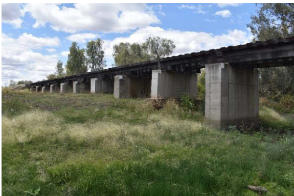
Figure 4-13: The 12 span timber and concrete constructed underbridge over Duffy's Creek at Chainage 667.37
