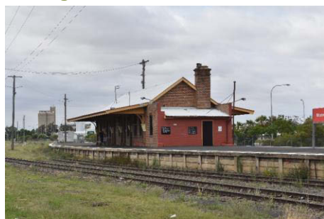
Figure 5-5: Moree Railway Station, view south. Source: Artefact Heritage
