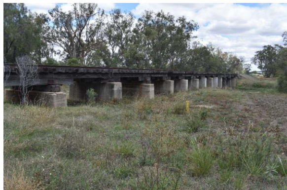
Figure 4-14: The 13 span timber and concrete constructed underbridge over Duffy's Creek at Chainage 667.21
