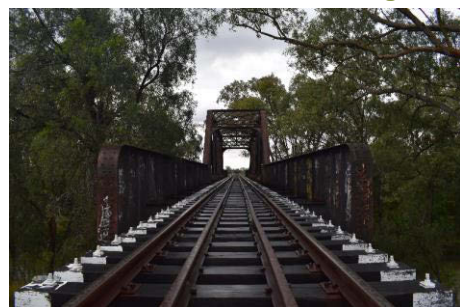
Figure 5-2: Mehi River Bridge, view north. Source: Artefact Heritage
