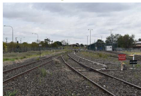
Figure 5-6: View north from Moree Railway Station to the CIZ. Source: Artefact Heritage
