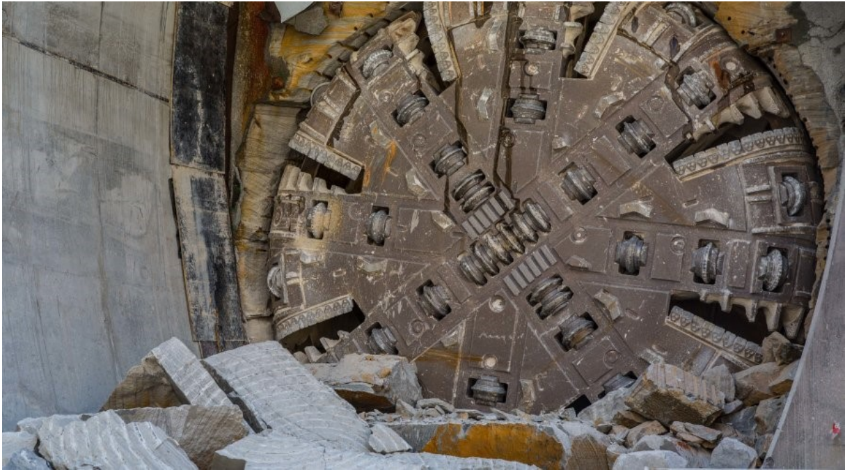
Figure 8-3 Photo of a tunnel boring machine at Epping Station on the Metro North West Line
