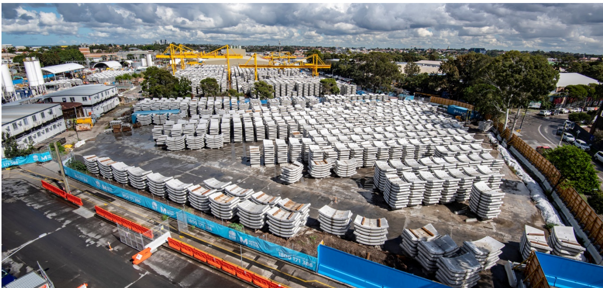
Figure 8-4 Photo of the tunnel segment storage area at Marrickville for the Sydney Metro City & Southwest project
