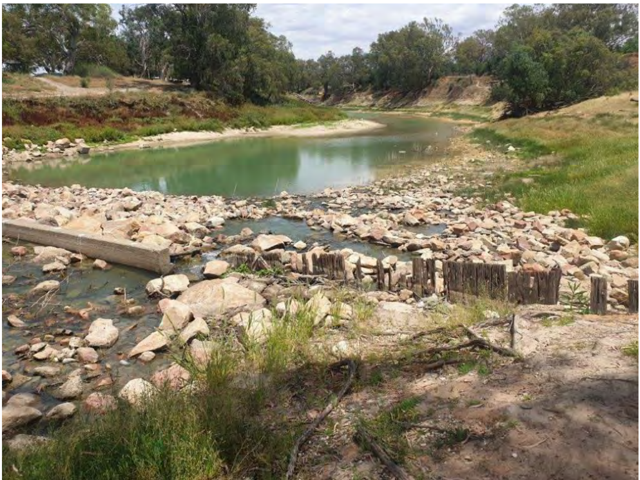
Photo 2-1 Erosion of the river channel and degradation of the right abutment of the existing weir structure
