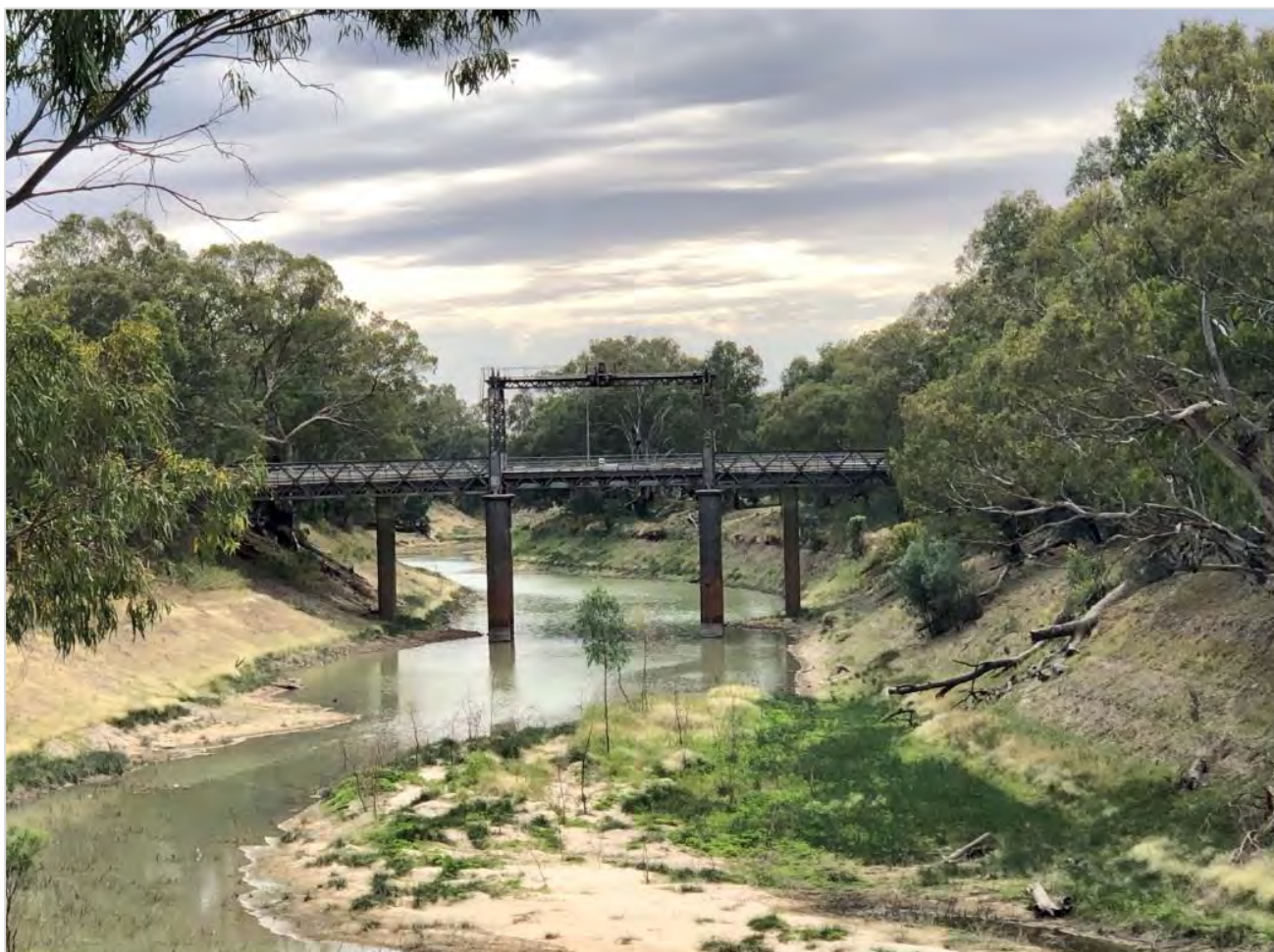
Photo 15-1 Wilcannia Bridge and central lift span, facing north-east from left riverbank downstream
