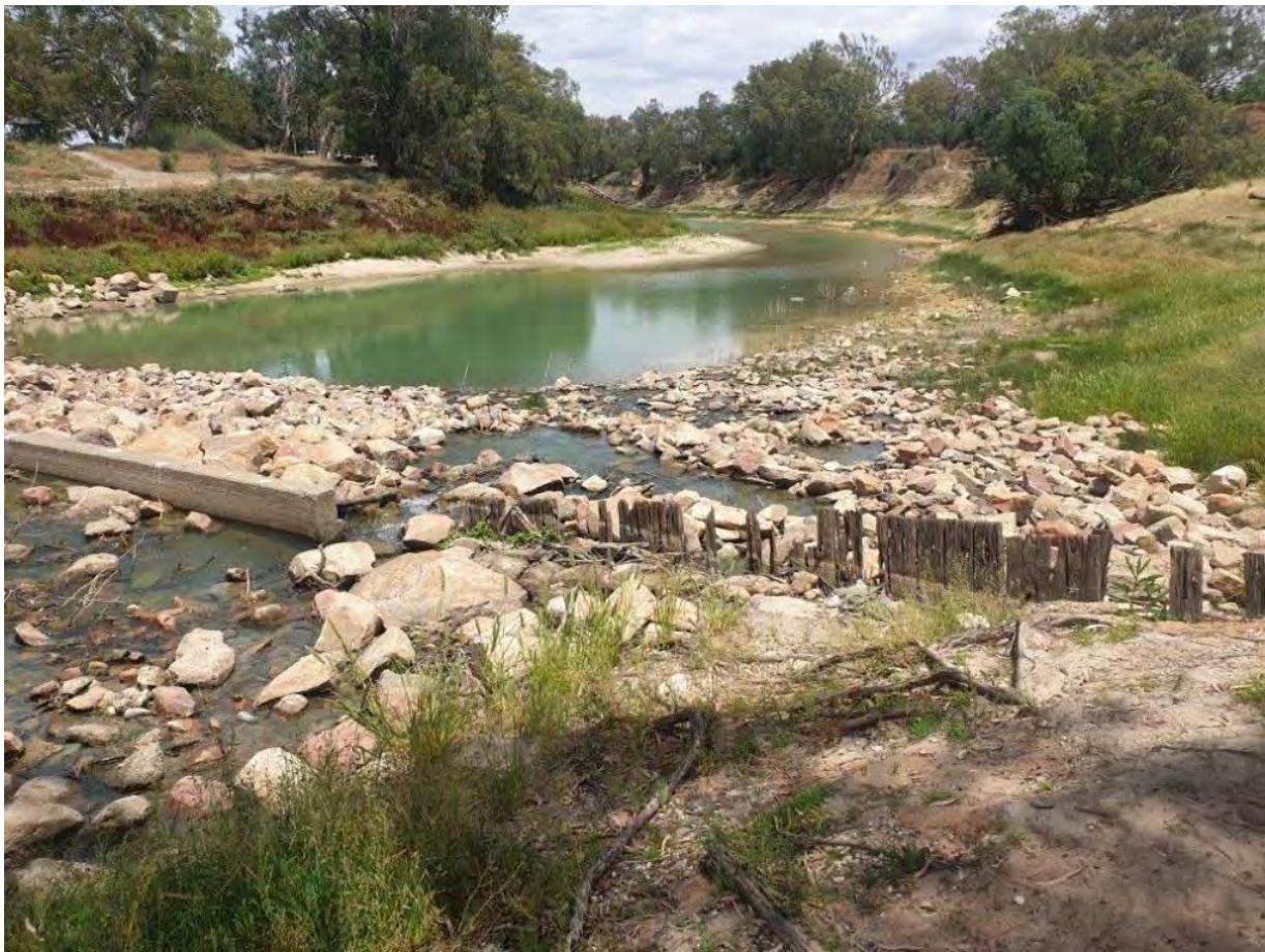
Photo 4-1 Erosion of the river channel and degradation of the right abutment of the existing weir structure
