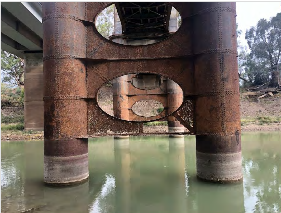
Figure 5-4 Lower pier cross ties with significant deterioration below the elliptical frame; facing southeast (Jacobs 2020)
