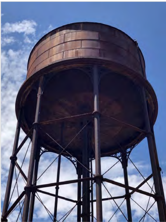
Figure 5-39 Cast-iron tank, riveted plate iron and decorative brackets; facing east from base of tank (Jacobs 2020)
