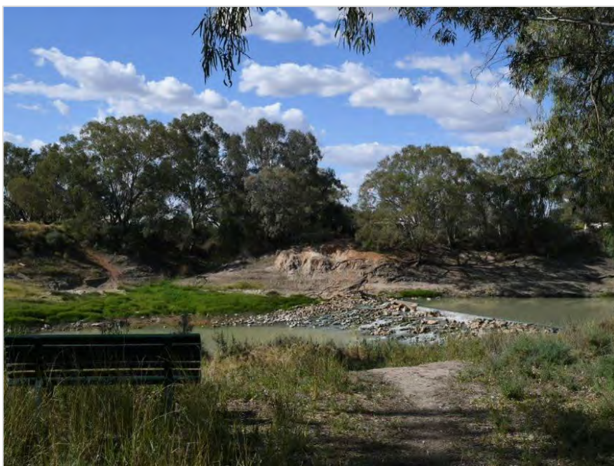
Figure 5-43 Current weir showing extensive bank erosion on the northern bank; facing northeast (Jacobs 2020)
