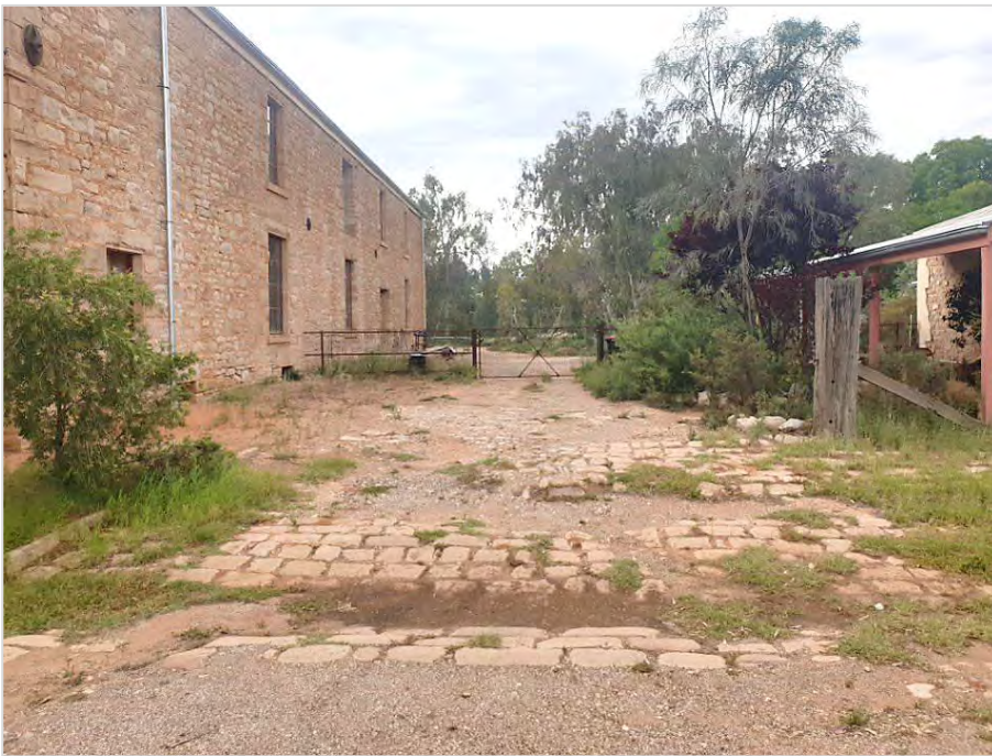
Figure 5-24 Sandstone flagged surface and guttering; facing southeast from Reid Street (Jacobs 2020)
