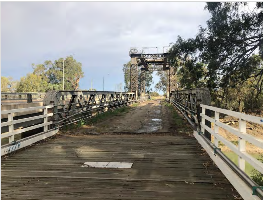
Figure 5-3 Timber approach on the Wilcannia township side of the bridge, remnant asphalt wearing surface; facing southeast (Jacobs 2020)
