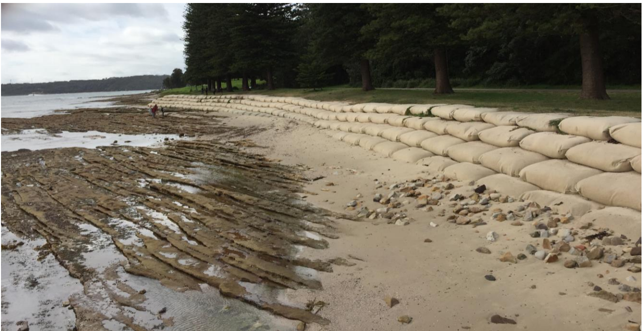
Figure 1-5 GSC Sandbags protecting the Norfolk Island Pines
