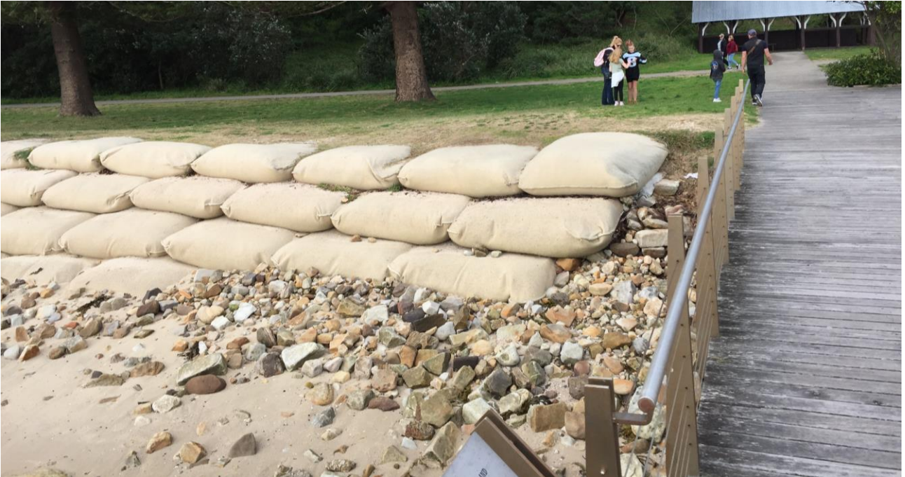
Figure 1-6 GSC wall Termination adjacent to the Jetty
