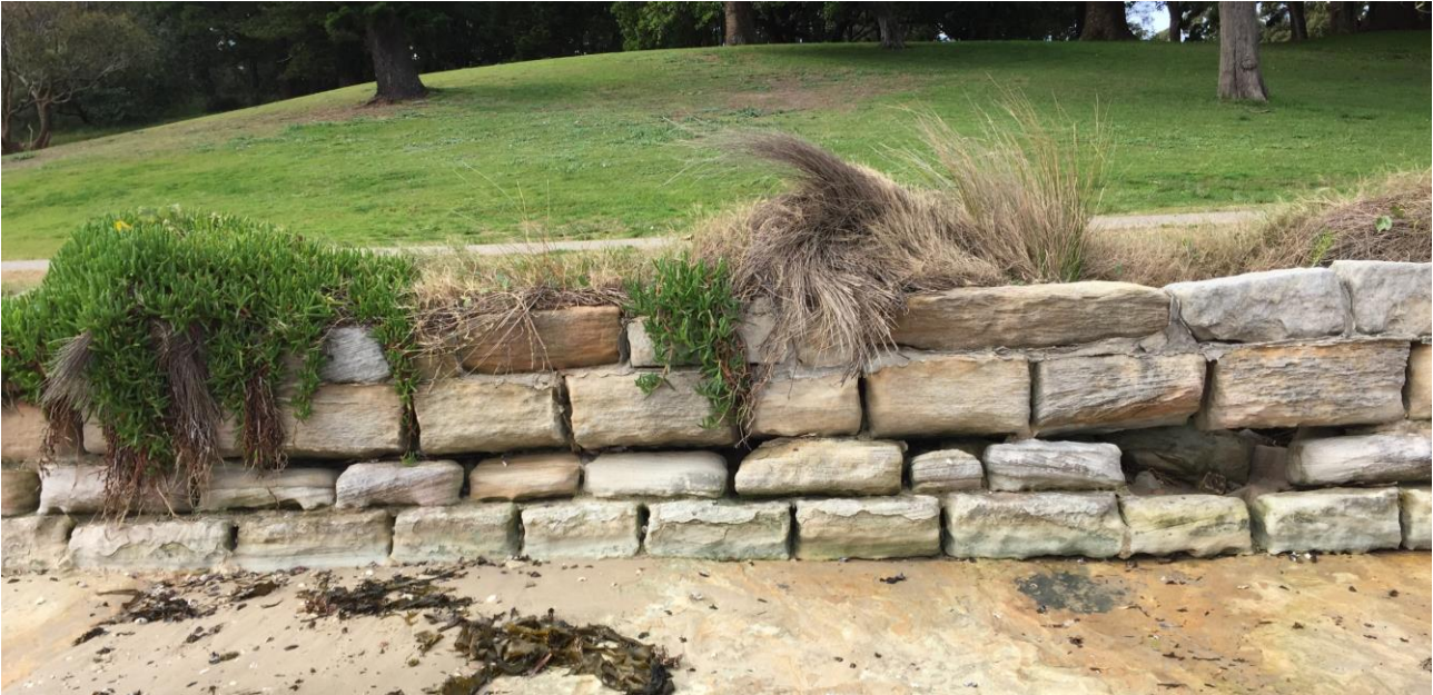
Figure 1-8 Example of Missing Blocks from the Sandstone Wall
