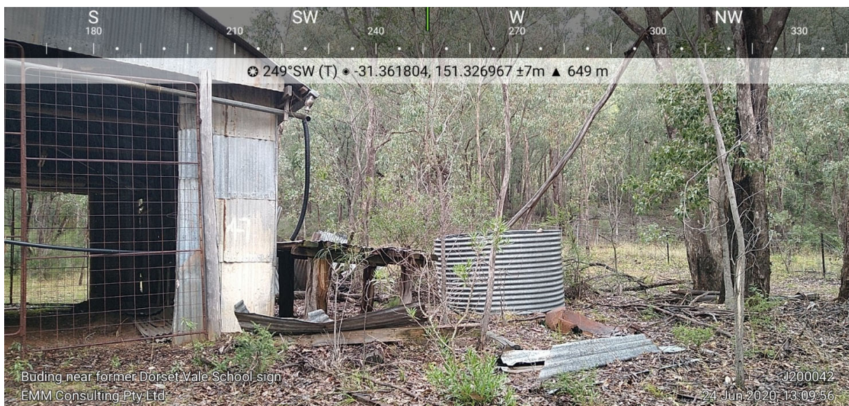
Plate 8 Building near former Dorset Vale School sign
