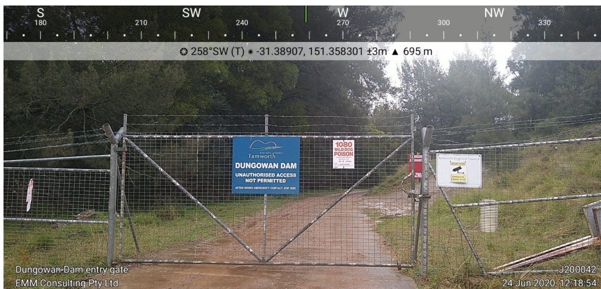
Plate 1 Existing Dungowan Dam entry gate
