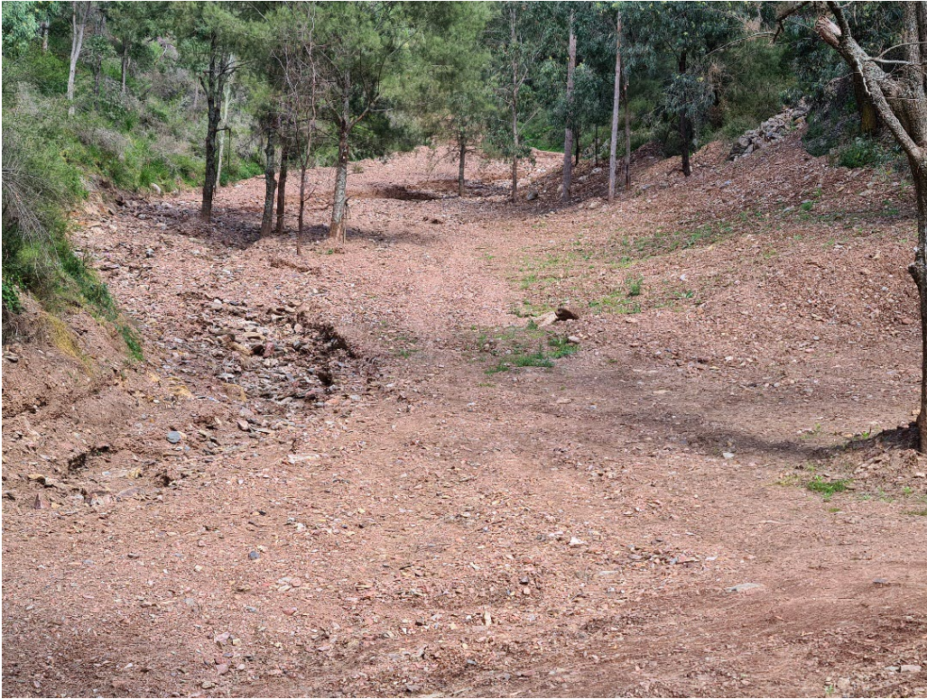
Photograph 4.2 Eroded sediments in a lateral gully that feeds Dungowan Creek
