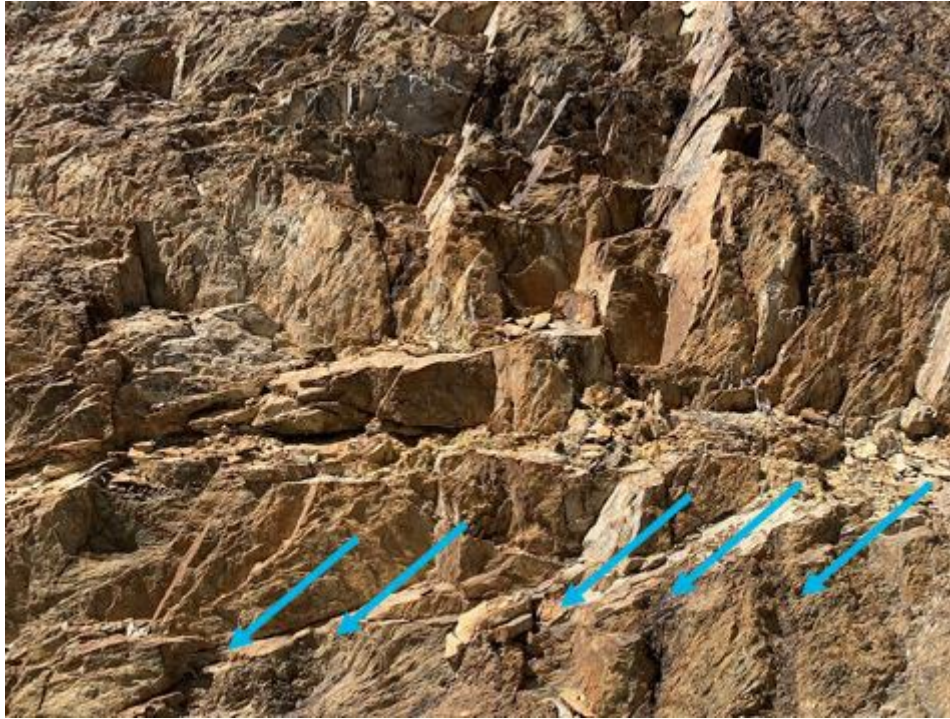
Plate A.82 Detail of the cutting face showing the natural breakage of the shale as well as possible tamping scars (indicated). View south-east.
