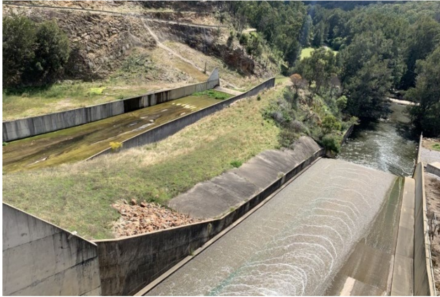
Plate A.13 Primary and secondary spillways; view north-west.
