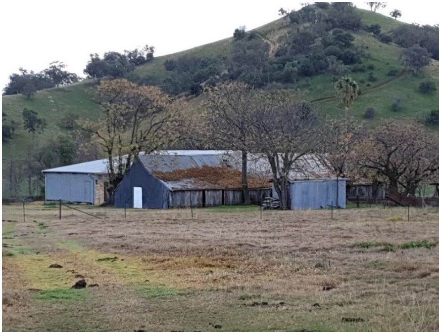
Plate A.91 Sheds on Dungowan Station; view north. The shed with the ogee roofline has timber slab walls.
