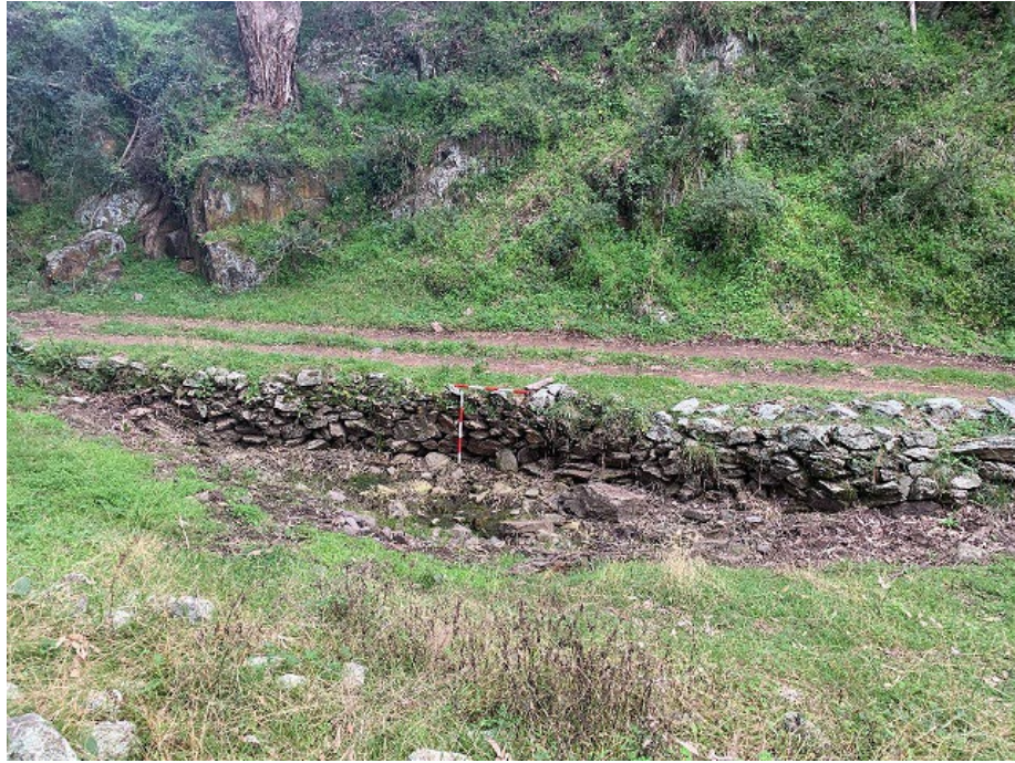
Plate A.42 View north to a random rubble retaining wall along a track. (September 2020).
