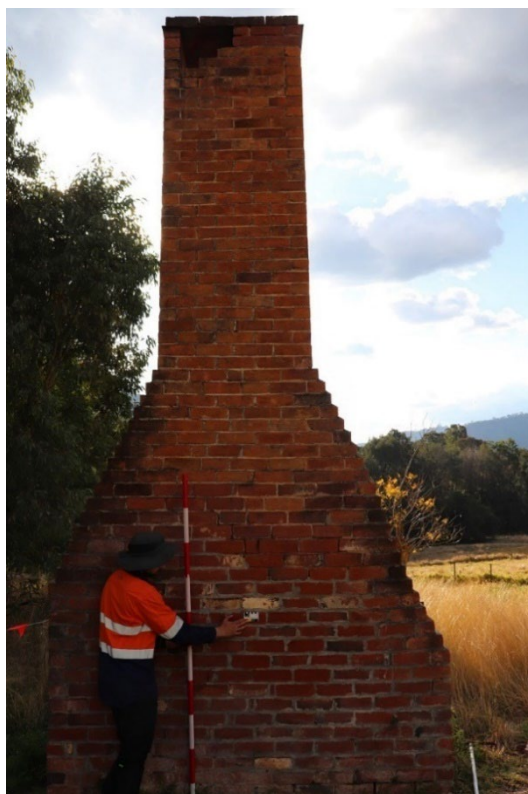
Plate A.64 The external elevation of the chimney stack at Hillcrest showing reused brick, repointing, and scale. View north-west; scale = 2 m.
