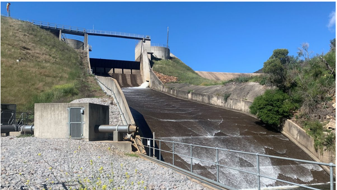
Photograph 6.2 Existing Dungowan Dam spillway chute and downstream face of embankment
