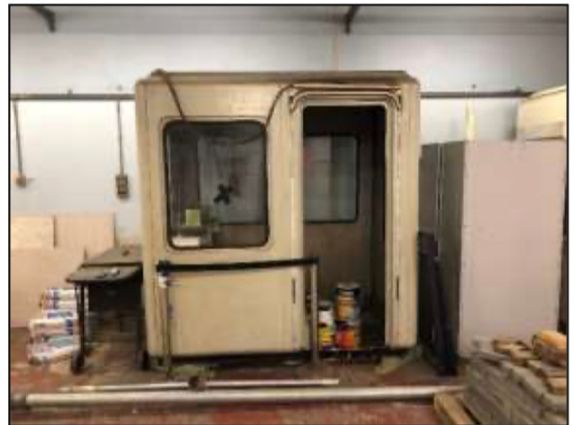
Figure 4: Guard Booth located in the mezzanine level.
