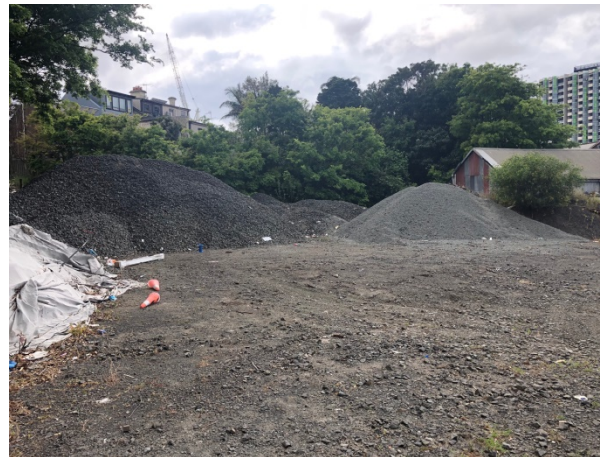
Figure 10 Eveleigh Railyard area, view to gravel stockpiles, looking north (Image source: AECOM, 2019).
