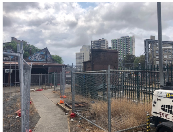
Figure 12 View to train line and Redfern Station beyond, right of image (Image source: AECOM, 2019).
