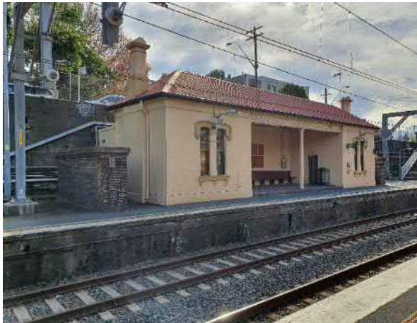
Figure 42 Waiting room on Platform 1
