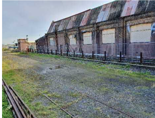
Figure 76 Telecommunication's Equipment Centre
