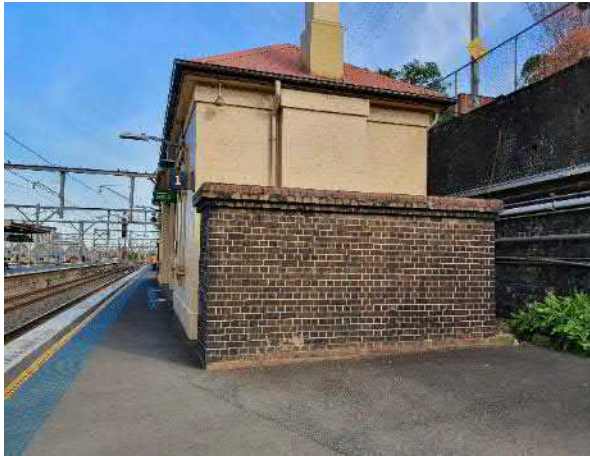
Figure 40 Engine Dive Ventilation Shaft on Platform 1 adjacent to Waiting Room
