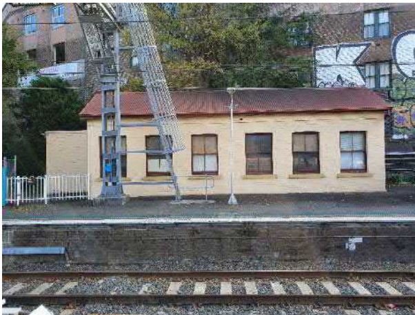
Figure 44 East elevation of Office building showing Victorian styles station building with typical colour scheme
