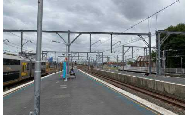
Figure 115 View from Platform 4/5 looking south towards Eveleigh Railyards in approximate location of proposed footbridge showing the visual clutter of overhead wiring system
