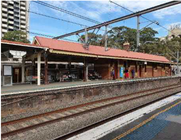
Figure 67 Eastern elevation of Platform 8/9 building
