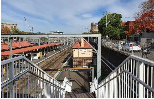
Figure 114 View 1 from the top of Platform 1 and existing Concourse looking south. View to Eveleigh Railway Workshops is obscured by the overhead wiring system
