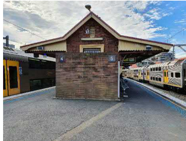
Figure 58 Southern elevation of Platform 4/5 building showing timber valance and low height privacy masonry wall
