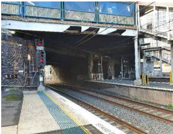
Figure 34 Platform 2/3 showing masonry wall with concrete facing
