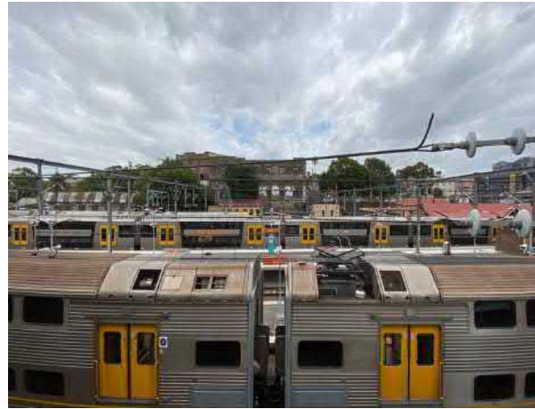
Figure 118 View from current Marian Street entrance across platforms approximating alignment of proposed footbridge
