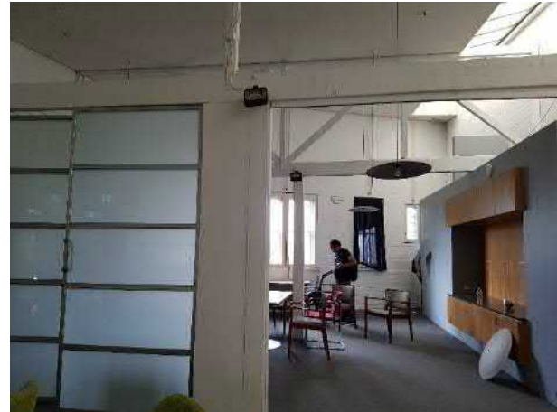
Figure 107 Upper level showing light weight partitions, exposed timber trusses and skylight
