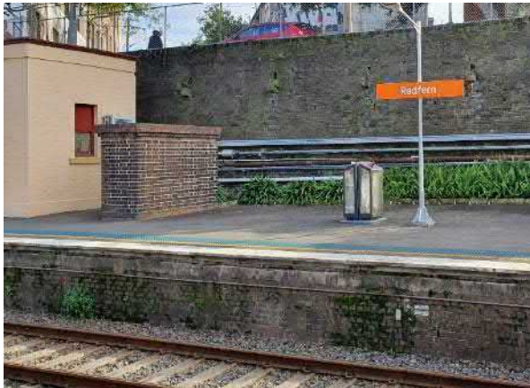
Figure 32 Platform 1 walls show typical masonry wall with a battered profile
