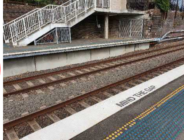
Figure 72 Southern end of Retaining wall showing entry stair to Marian Street
