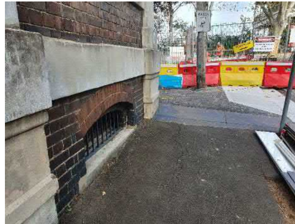
Figure 112 Intersection of Ivy and Lawson Street showing basement windows adjacent to the footpath
