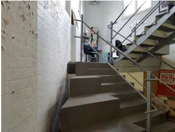
Figure 100 View of Mezzanine and stair
