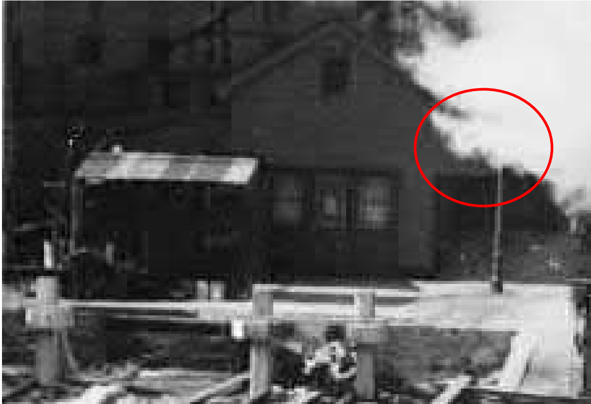
Figure 174 c.1930 photograph in detail showing Platform 1 Office Building with annex and timber and glass doors/windows to southern elevation
