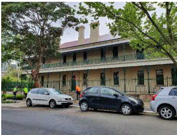
Figure 85 View of Chief Mechanical Engineer's Office building from Wilson Street
