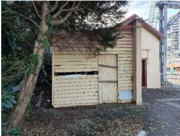
Figure 46 Brick wall on southern elevation with timber clad room
