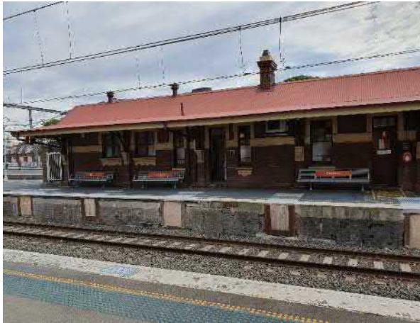
Figure 61 Eastern elevation of Platform 6/7 building
