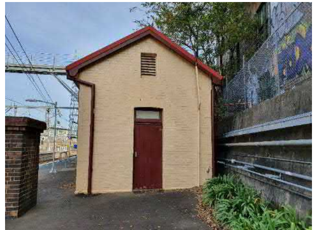
Figure 49 Entry door on the northern elevation
