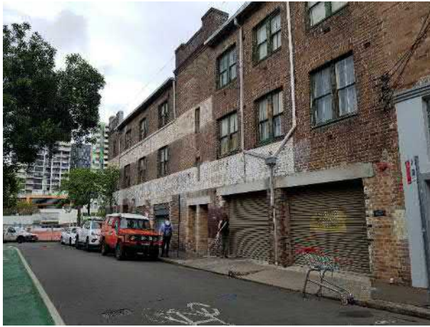
Figure 94 Northern elevation (No127 end of the building)
