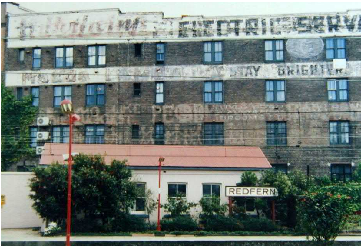
Figure 178 View of Platform 1 Office Building showing former garden (Source: Sydney Trains Virtual Plan Room)
