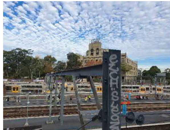
Figure 74 OHW structure SWI+304
