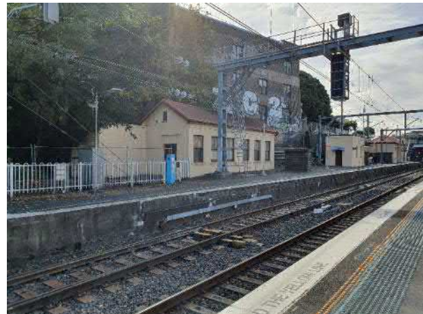
Figure 45 South easterly view of Office building along with Store Building and Waiting room beyond
