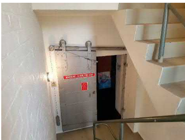
Figure 104 Fire stair with early warehouse door
