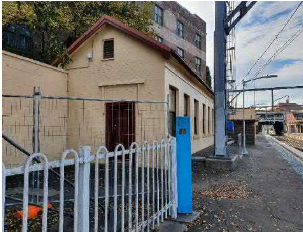
Figure 176 Southern elevation of Platform 1 Office Building showing modification to doors
