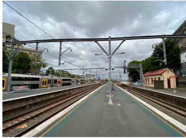
Figure 123 View 7 from Platform 2/3 looking north
