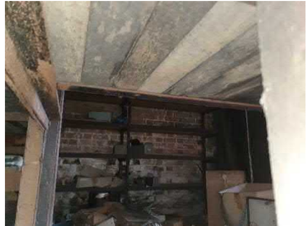
Figure 53 Interior of timber-clad building showing masonry wall to rear and timber panelled roof
