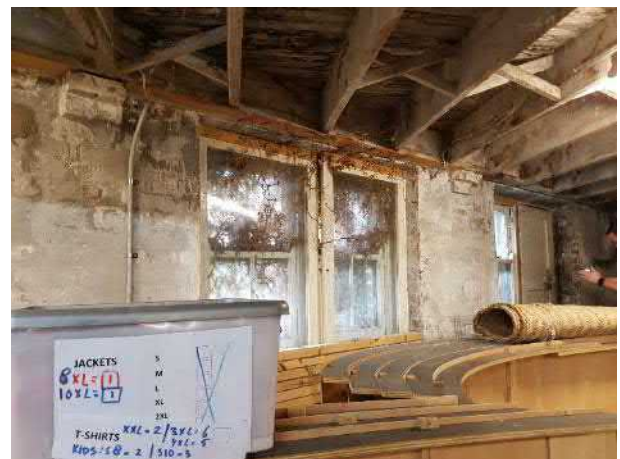
Figure 99 Basement level showing internal timber windows
