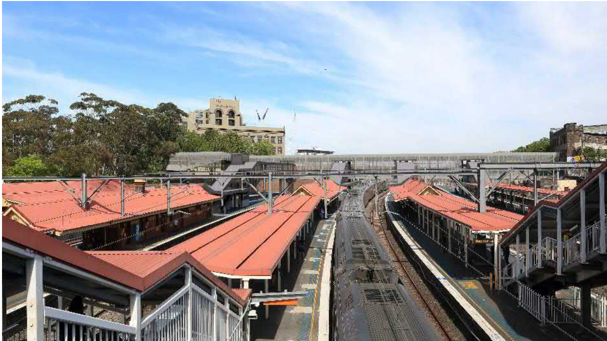
Figure 151 View of the proposed concourse from existing concourse (identified significant view)
