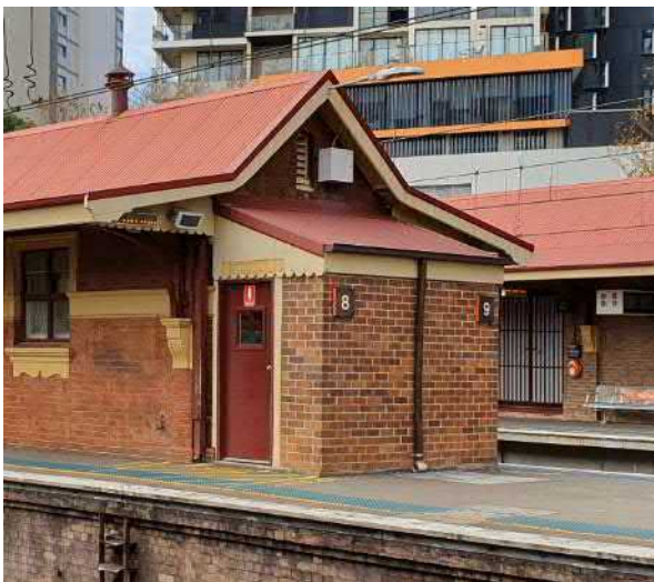
Figure 69 Lean-to structure with a corrugated roof over
