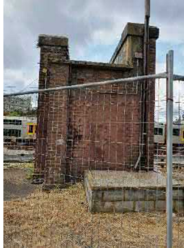
Figure 78 Extant footbridge brick piers
