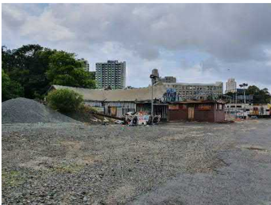
Figure 79 Outbuildings including Interlocking Store, Southern Store, Northern Store and Brick Toilet
