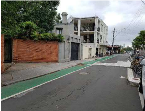
Figure 88 Western side of Little Eveleigh Street (northern portion)
