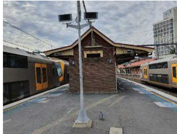
Figure 62 Southern elevation of Platform 6/7 building showing timber valance and low height privacy masonry wall
