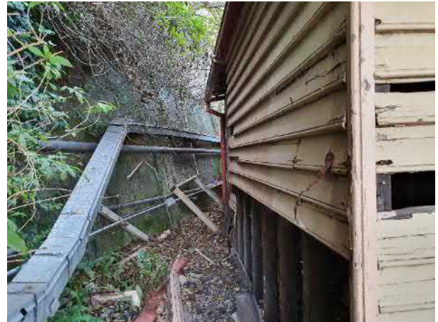
Figure 47 Western elevation of lean-to
