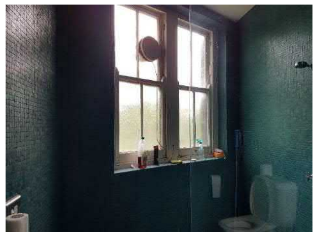
Figure 105 Typical wet area
