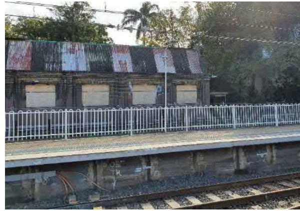
Figure 33 Southern end of Platform 1 showing pre-cast pressed concrete paving slabs
