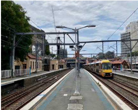
Figure 122 View 6 from Platform 2/3 looking south (AECOM 2020)
