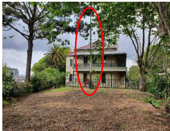
Figure 86 Northern elevation of Chief Mechanical Engineer's Office building showing garden, fence and flagpole (circled)
