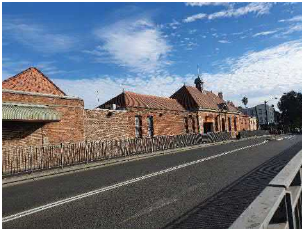
Figure 21 Lawson Street overbridge with primary entrance to Redfern Station
