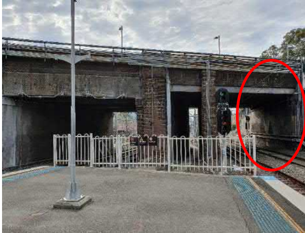
Figure 71 Northern end of Retaining wall
