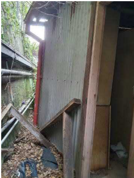
Figure 48 Lean-to with corrugated iron wall cladding and roof on western elevation
