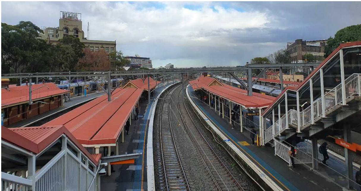
Figure 25 View from the existing concourse looking towards Eveleigh Railway Workshops are impeded by the overhead wiring structures
