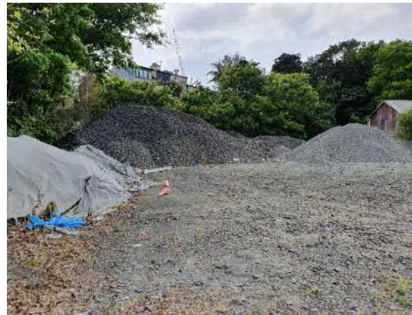
Figure 81 Area used as material storage and overgrown (background)
