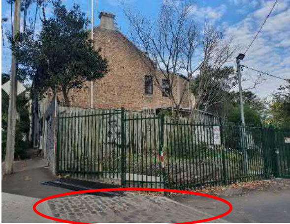
Figure 77 Current gated entry accessing the Eveleigh Railway Workshops where the former footbridge entry was located showing brick paving at driveway
