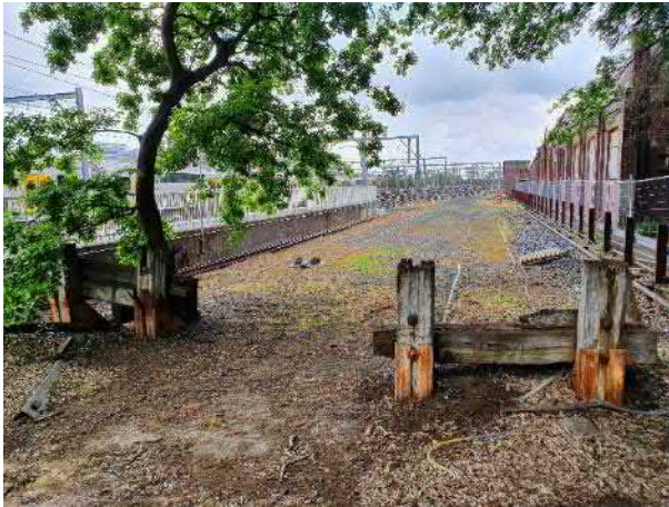
Figure 56 Buffer stops at the termination of Elston's Sidings and Telecommunications Building (right)
