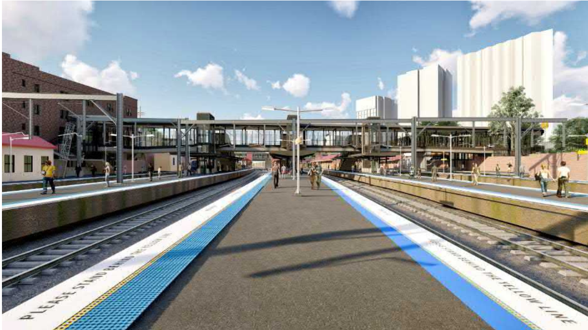
Figure 140 Option 1 – Showing concourse with glass panels to three metres above finished floor level and open over with dark coloured structural and framing elements
