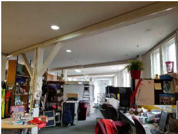
Figure 102 Ground floor showing contemporary insertions (columns, beams and ceiling)
