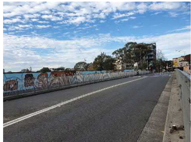
Figure 22 Lawson Street overbridge with NUAA Wall
