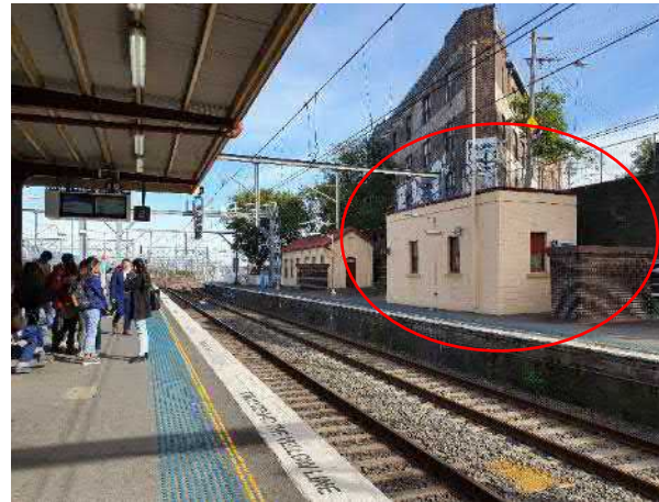
Figure 43 The Store Building on Platform 1 (circled red) with Platform 1 Office Building beyond
