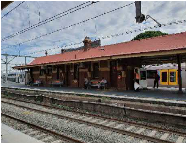
Figure 57 Eastern elevation of Platform 4/5 building
