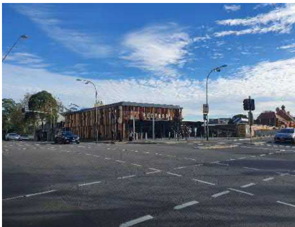
Figure 28 Secondary entrance at the intersection of Gibbons and Lawson Streets
