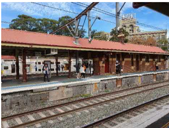
Figure 36 The substructure on Platforms 6/7 has been repaired
