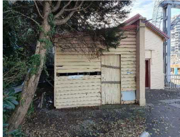
Figure 177 Southern addition is not the annex shown on 1930 photograph. Brick wall appears taller and skillion roof to annex pitches in the different direction
