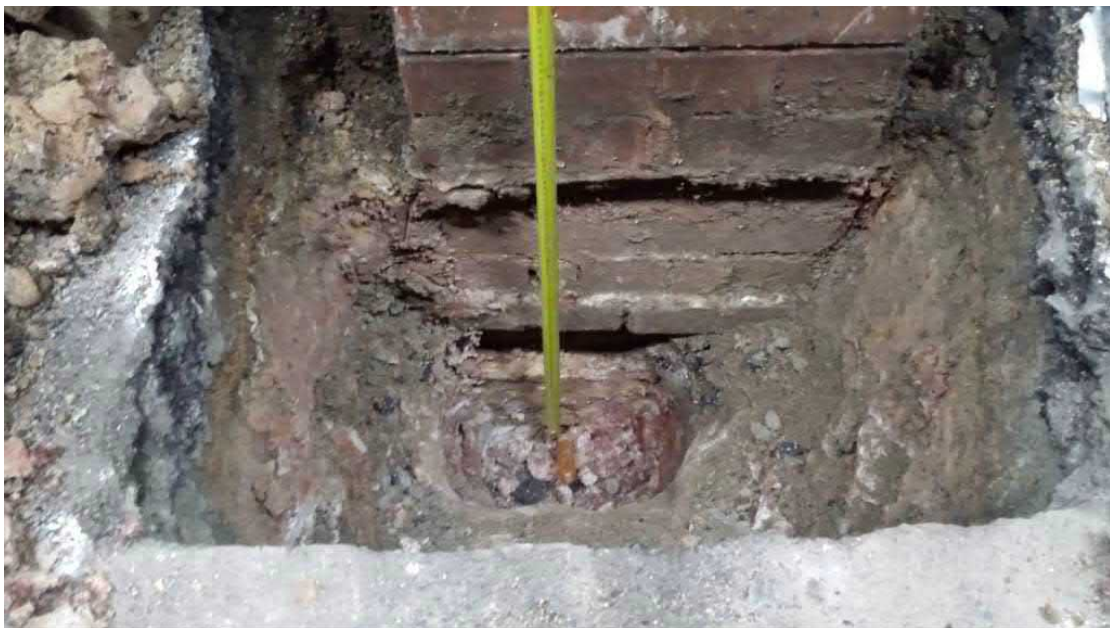
Photo 3: Concrete footing at the base of the test pit,
