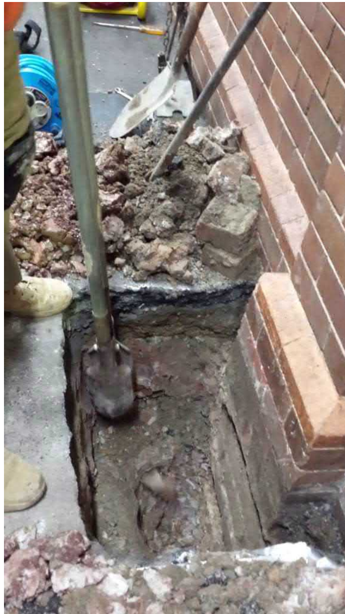
Photo 1: Footing excavation for Station Building
