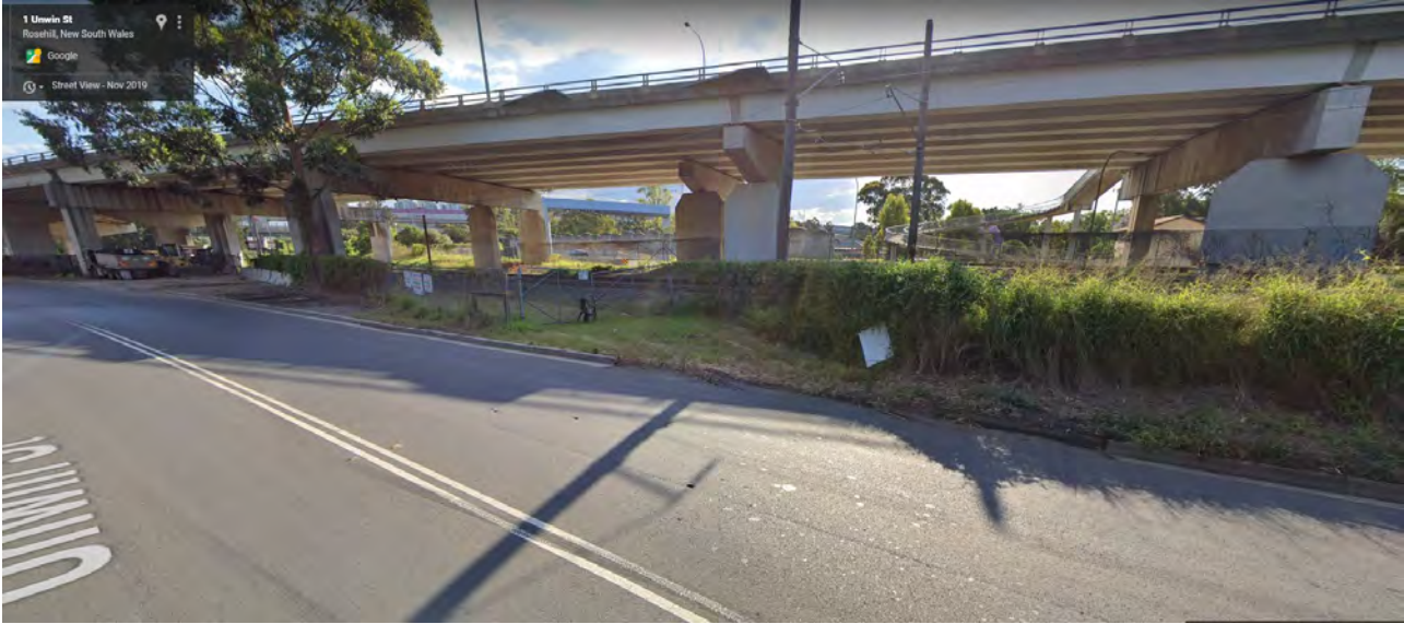
Figure 3-16: Unwin Street heavy vehicle access/ egress into-from the Rosehill site
