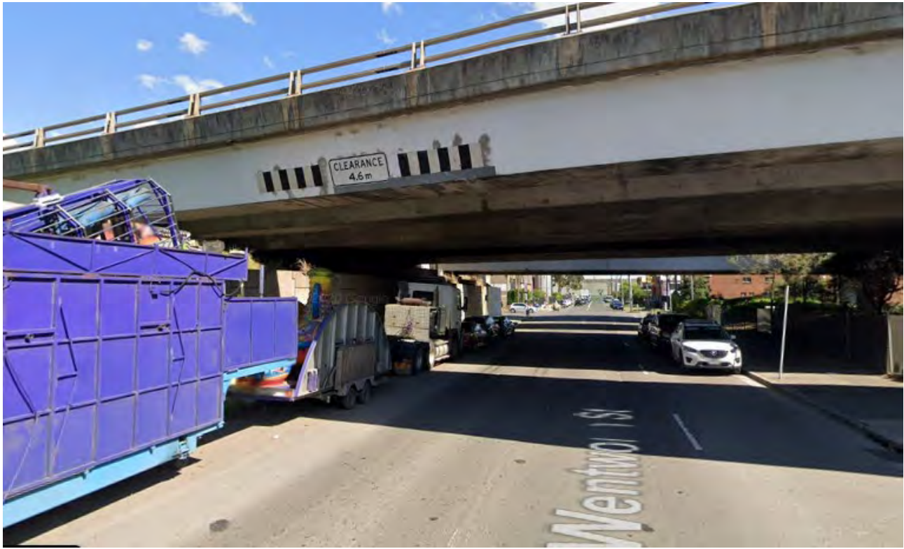
Figure 3-26: M4 Overpass on Wentworth Street
