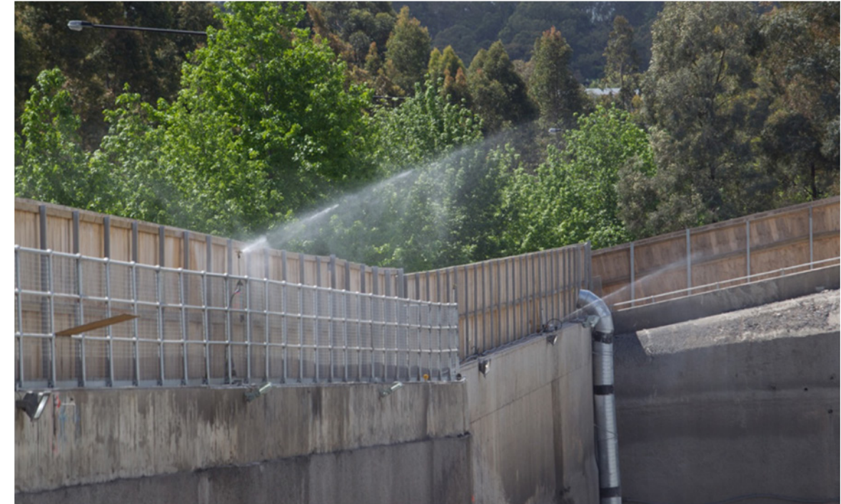
Figure 11 - Dust Mitigation at Norwest Station Site
