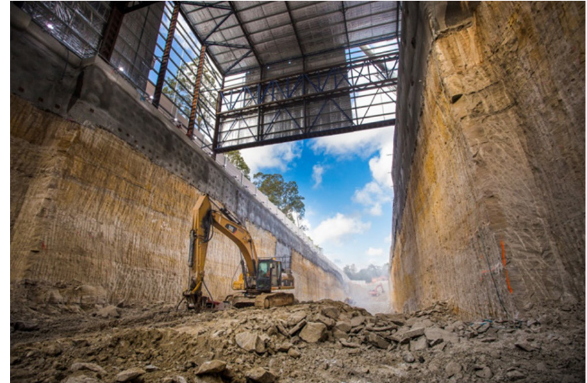
Figure 4 - Spoil and Excavation Works at the Showground Station Site
