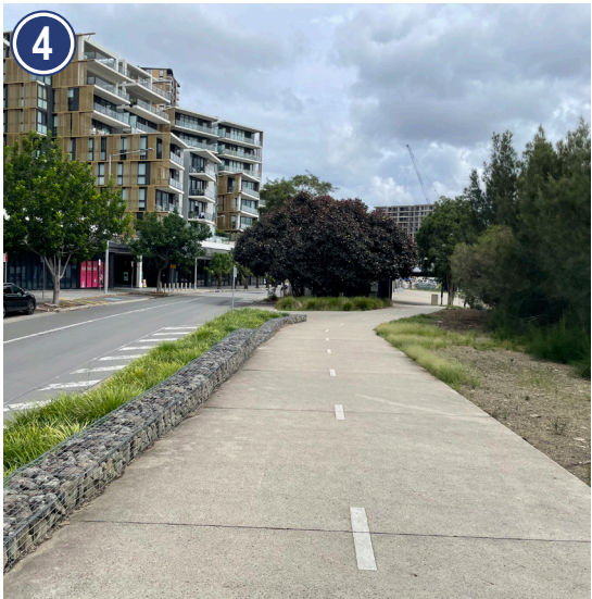
Figure 19: River Walk between Sydney Olympic Park Wharf and Peninsula Park - Shared Path - 4.0m
