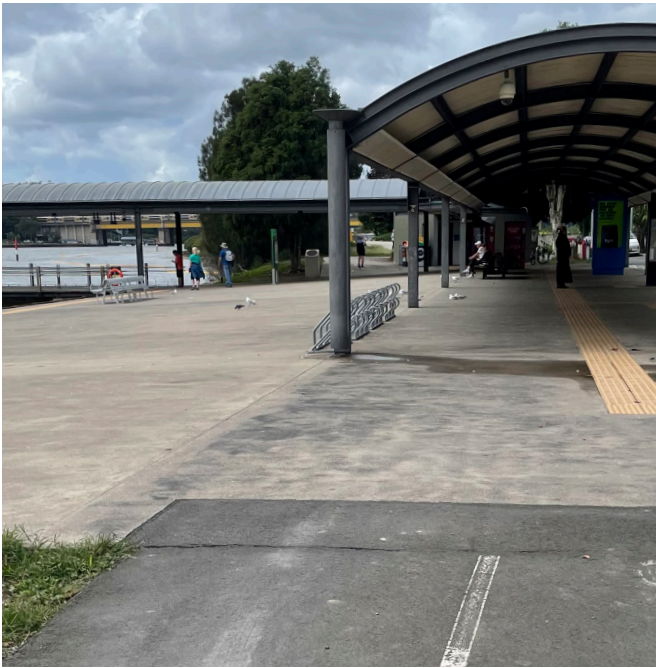
▶ CCTV Camera at Sydney Olympic Park Wharf
