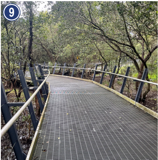
Figure 24: Parramatta Valley Cycleway - Boardwalk - Shared Path - 3.1m
