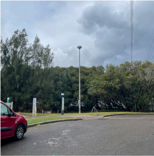
■ Lighting along Pedestrian/Cyclist Infrastructure - North foreshore car park
