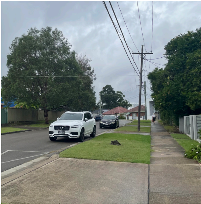
— Typical Street Lighting
