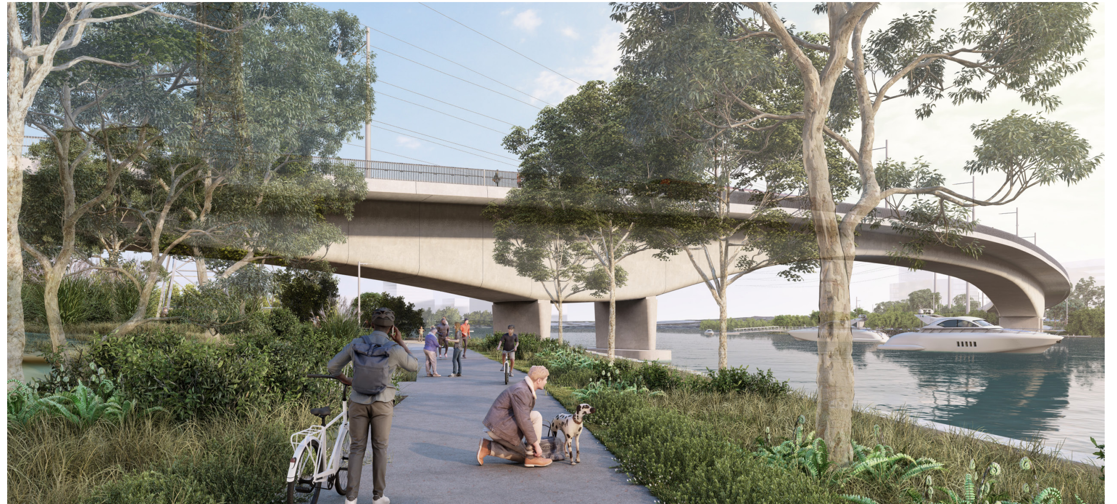
Figure 46: Looking West along the Upgraded River Walk
