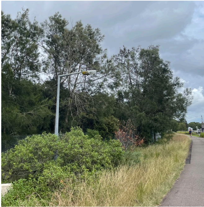
■ Lighting along Pedestrian/Cyclist Infrastructure - River Walk
