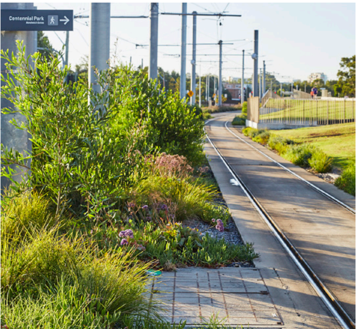
Figure 19: Light rail track separated from road with buffer planting, Randwick, Australia (credit: ASPECT Studios).
