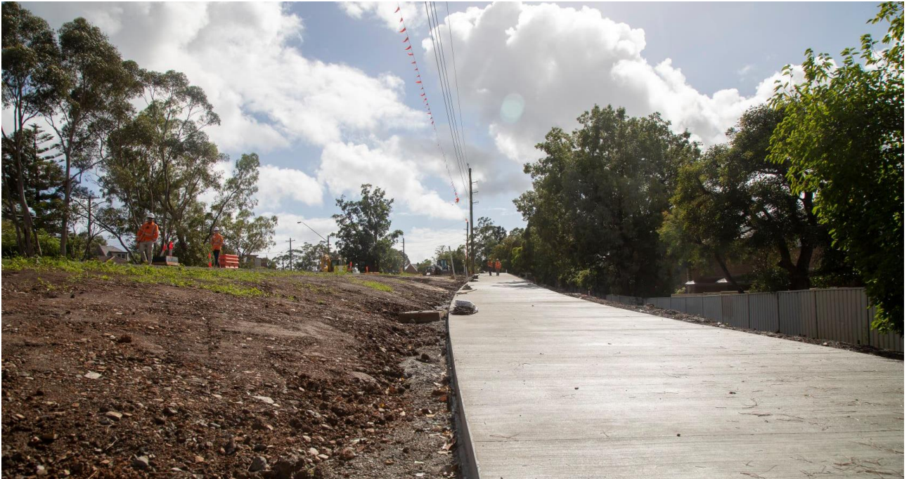
Figure 4.2: Construction of ATL as part of Parramatta Light Rail Stage 1 (TfNSW, 2022)
