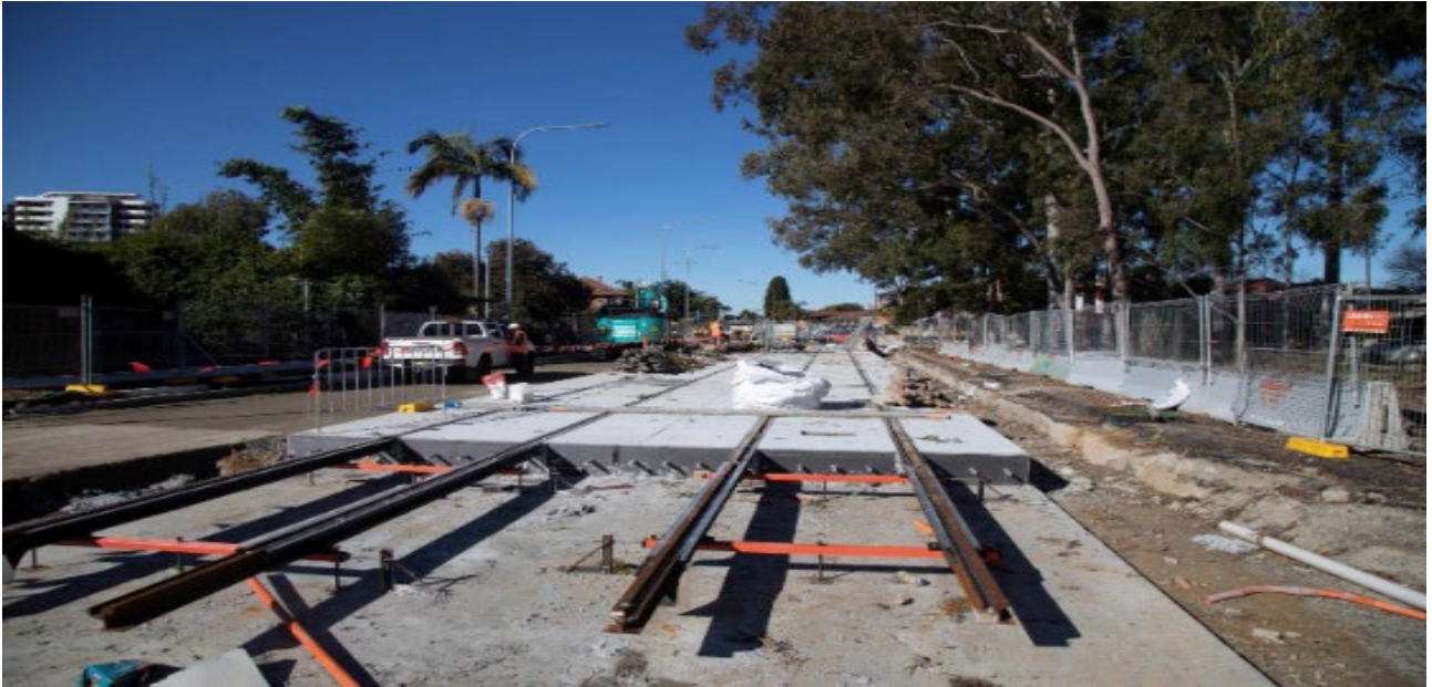
Figure 4.1: Track installation works during construction of Parramatta Light Rail Stage 1 (TfNSW, 2022)
