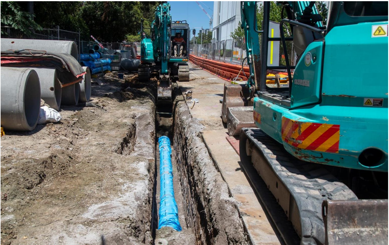
Figure 7.15 Image showing the laying of a small diameter water main in Westmead (Parramatta Light Rail Stage 1)
