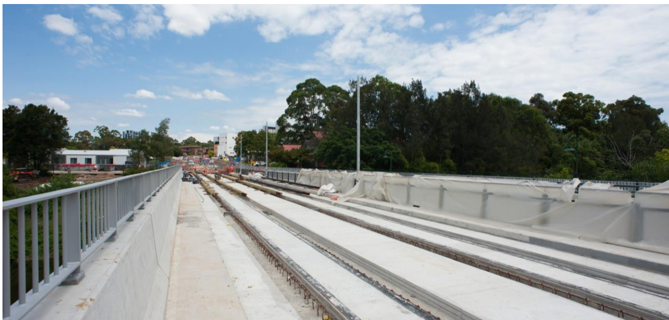
Figure 7.4 Image showing light rail track form for a Parramatta Light Rail Stage 1 bridge
