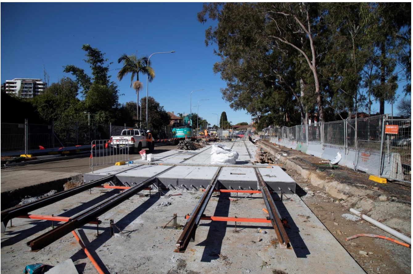
Figure 7.3 Image showing track installation works for Parramatta Light Rail Stage 1
