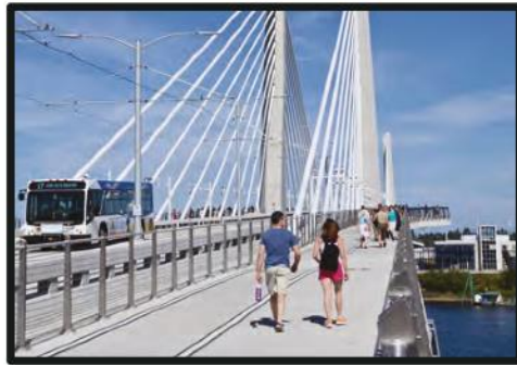
Separated facility over bridge
