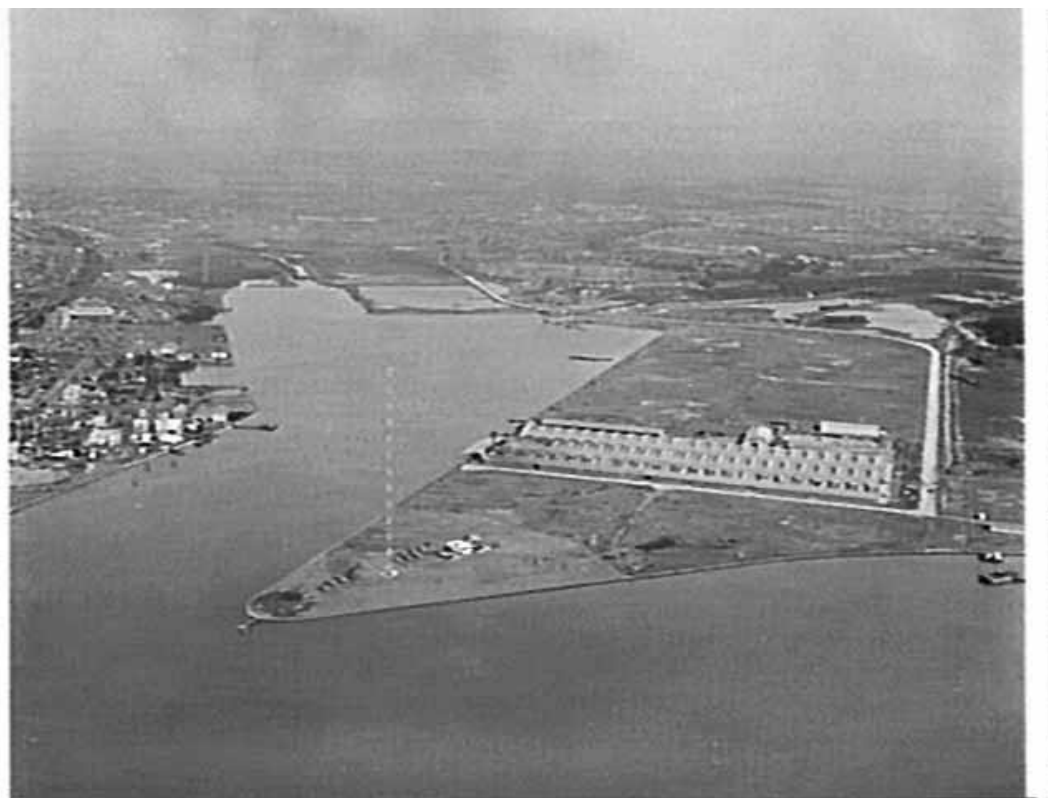
Plate 3.16: Aerial photographs of Ralph Symonds plywood factory, with unusual timber arch clerestory roof designed by Symonds, Homebush Bay, 1964 (State Library of NSW)
