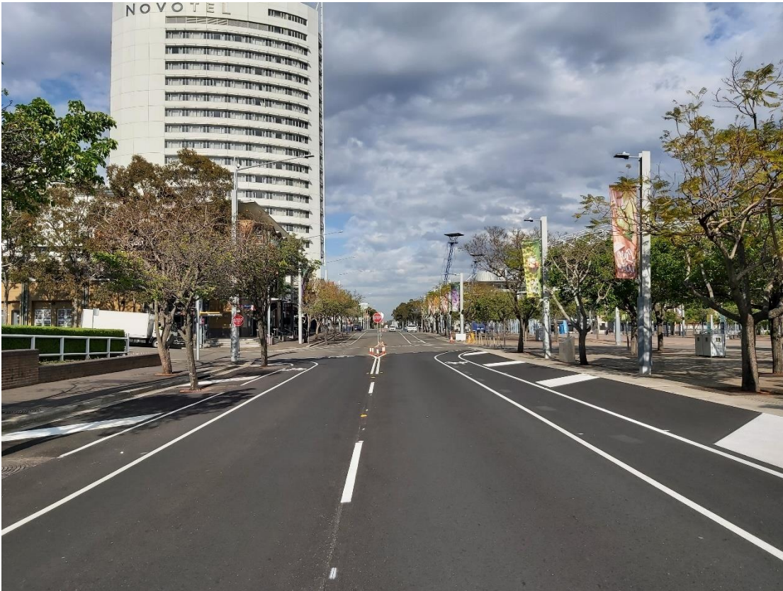
Plate 4.46: View west along Dawn Fraser Avenue (RPS 2021)
