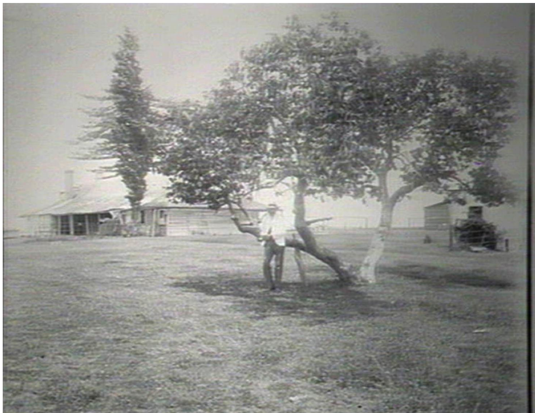
Plate 3.19: D’Arcy Wentworth’s homestead, back view, n.d. (State Library of NSW)
