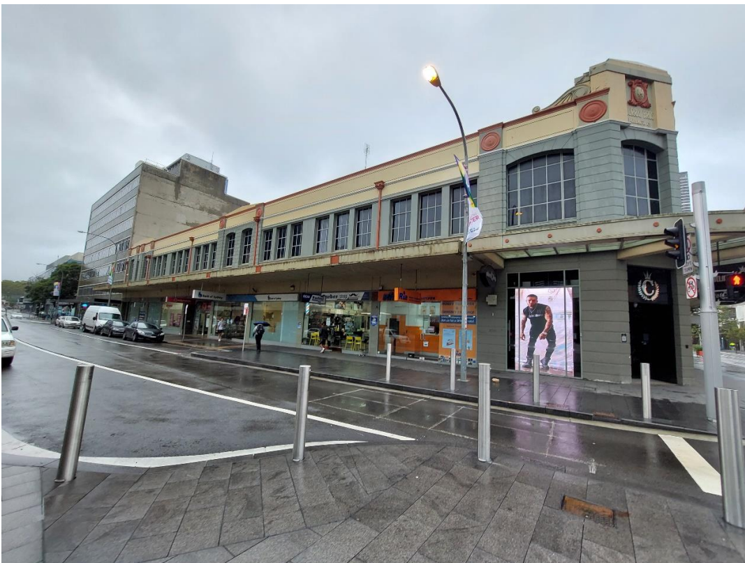
Plate 4.52: View north-west along Macquarie Street, showing Shop (and potential archaeological site) (Parramatta LEP Item No. I655) (RPS 2022)
