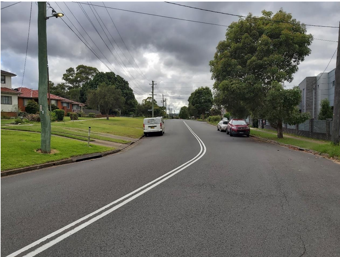
Plate 4.20: View east along Boronia Street near Spofforth Street (RPS 2021)
