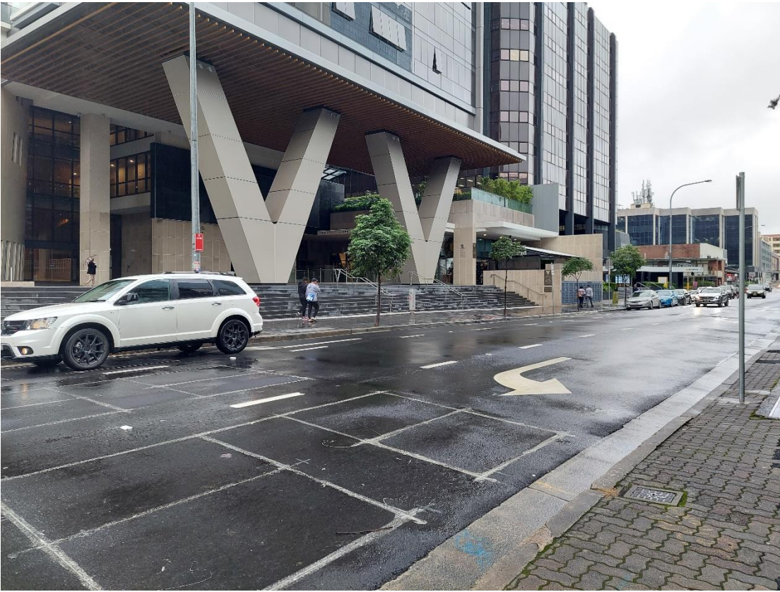
Plate 4.47: View west along southern side of Macquarie Street from Marsden Street (RPS 2022)
