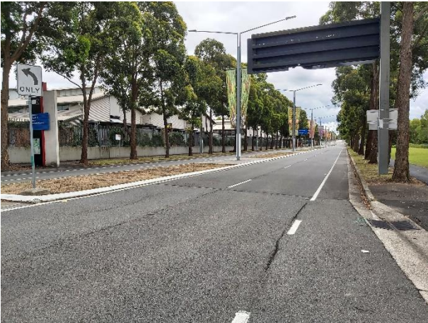
Figure 6-55: A streetscape in Sydney Olympic Park demonstrating the environment in the area
