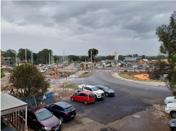
Figure 6-1: Grand Avenue, Camellia showing the general industrial nature of the suburb at present
