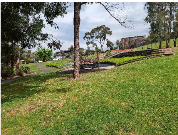
Figure 6-23: Ken Newman Park, Ermington. The project site includes a large section of this park.
