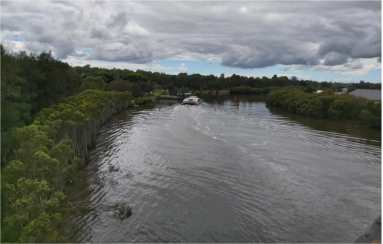
Figure 6-74: Approximate area of MAMU 01, adjacent to Rydalmere Wharf
