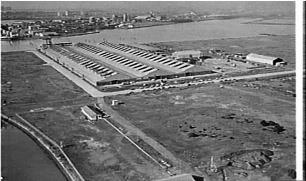
Figure 4-41: Aerial photograph of Ralph Symonds plywood factory, with unusual timber arch clerestory roof designed by Symonds, Homebush Bay. SLNSW, IE914726, FL914731
