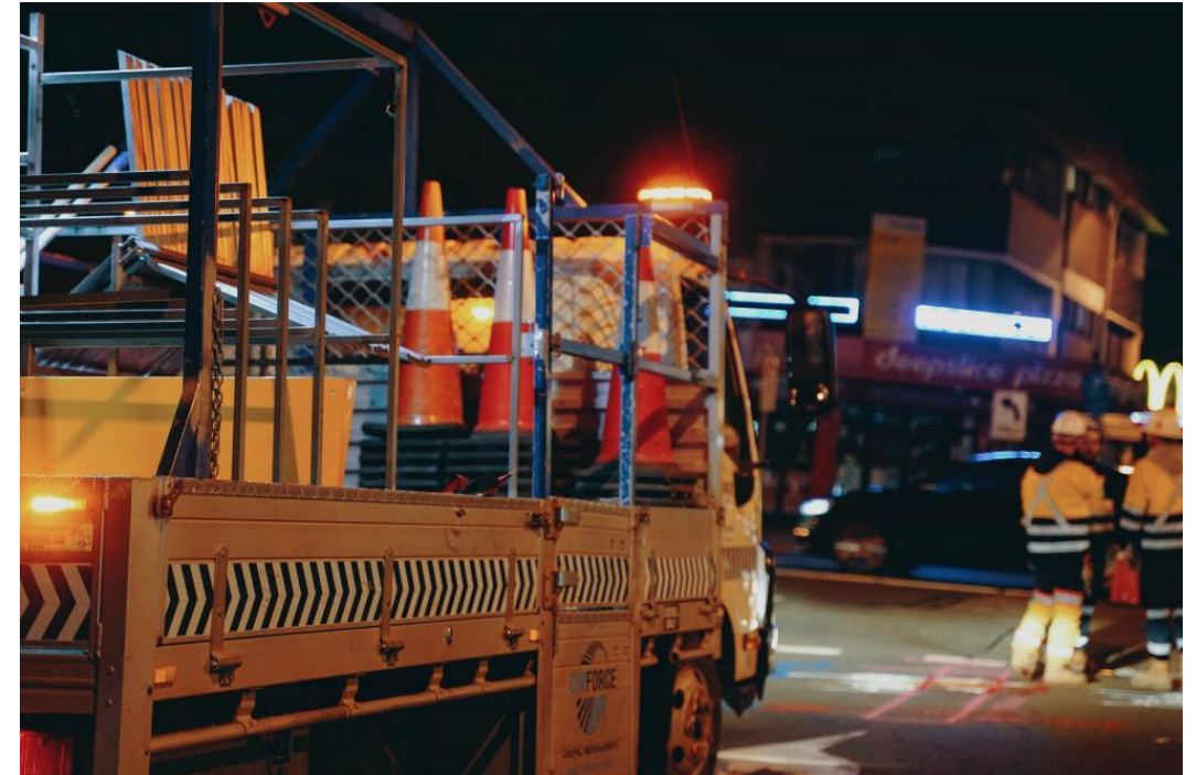
Parramatta Light Rail Stage 1 night time construction works
