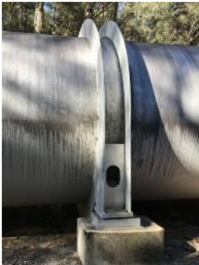
Picture 3-3. Example of a penstock saddle supports
