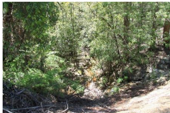
Trimbles Creek facing downstream of the existing surface pipeline anchor block
