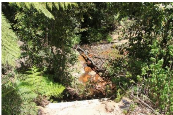
Trimbles Creek facing upstream of the existing surface pipeline anchor block
