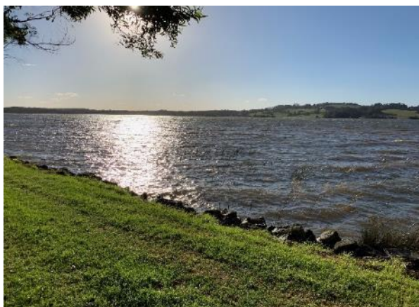
Fitzroy Falls Reservoir facing upstream toward the Burrawang Pumping Station
