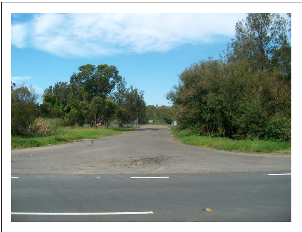
2. Existing 8.0 metre two way access from Andrews Road
