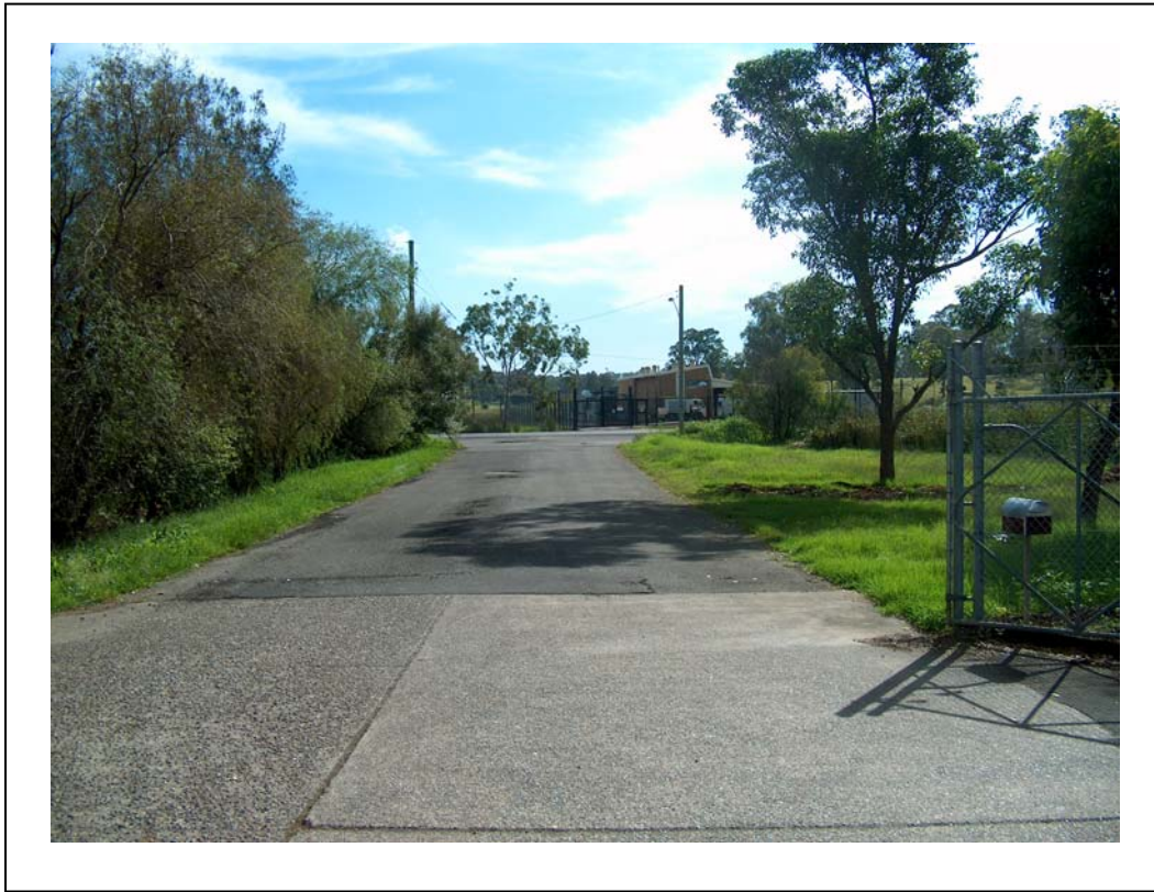
1. Existing 8.0 metre access to Andrews Road
