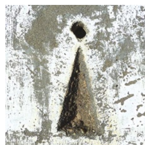
Drill Hole &amp; Wing in Kerb references adjacent boundary corner
